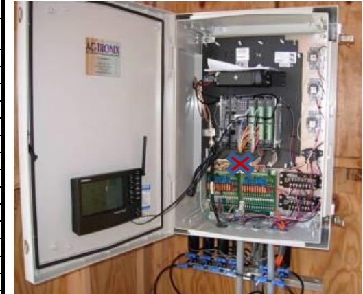
Irrinet system in wall cabinet.
