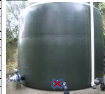
Plastic/Polyethylene water tank.
