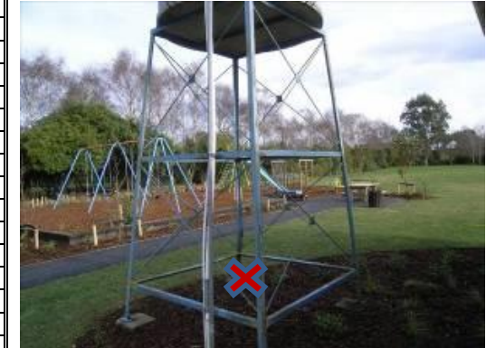
Steel water tower
