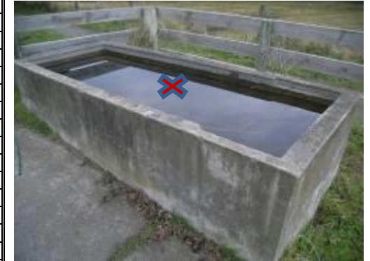
Rectangular concrete water trough, no ballcock.
