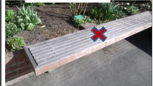
Wooden bench, steel frame, fixed within wall, varnished, and has no foot pad.
