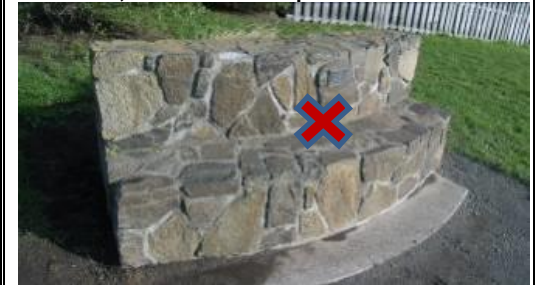
Stone seat, fixed to the ground, with a concrete footpad.
