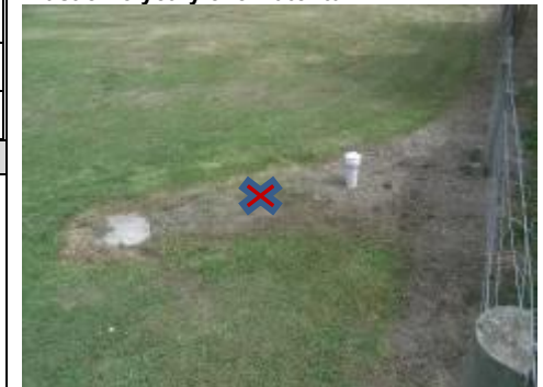
Buried Septic tank. Vent and access exposed.
