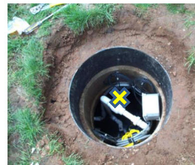
Centre of Pump X Y and Z (on pump)
