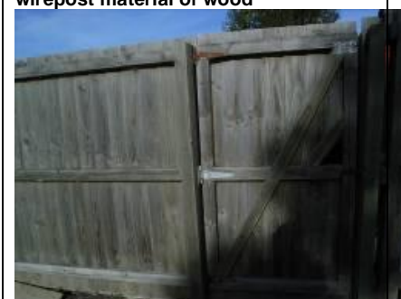
Gate type of pedestrian, gate style of paling, construction material of wood, post material of wood, surface finish of none.
