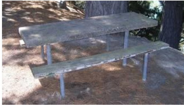
Picnic table with a concrete table top and steel frame. This table has no surface finish or footpad.
