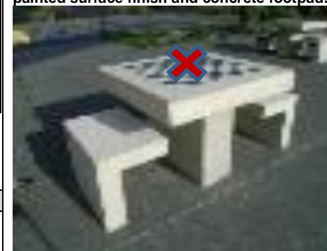
This chessboard on the table top gives it an artwork component. This is a concrete table with concrete frame, painted surface finish.
