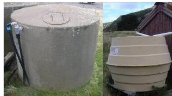
Concrete and Fibreglass Water Tanks
