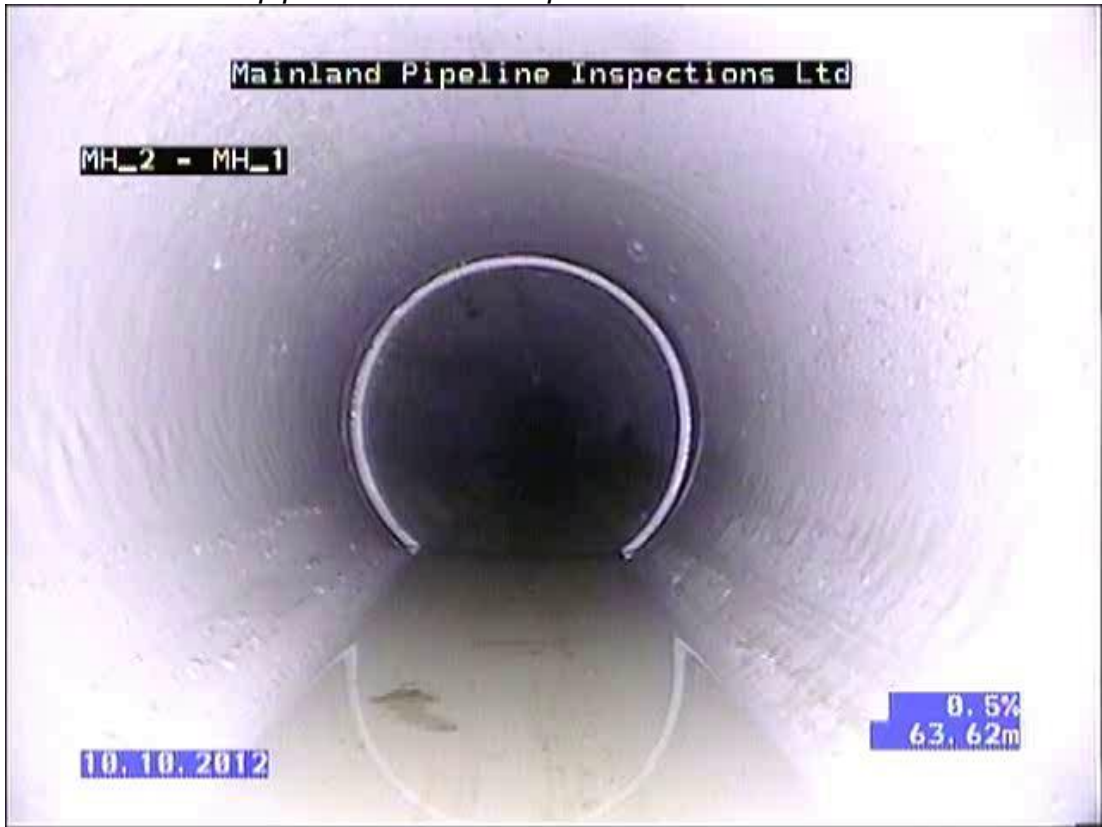
Photo 2: 225 mm pipe with a 20mm Dip
