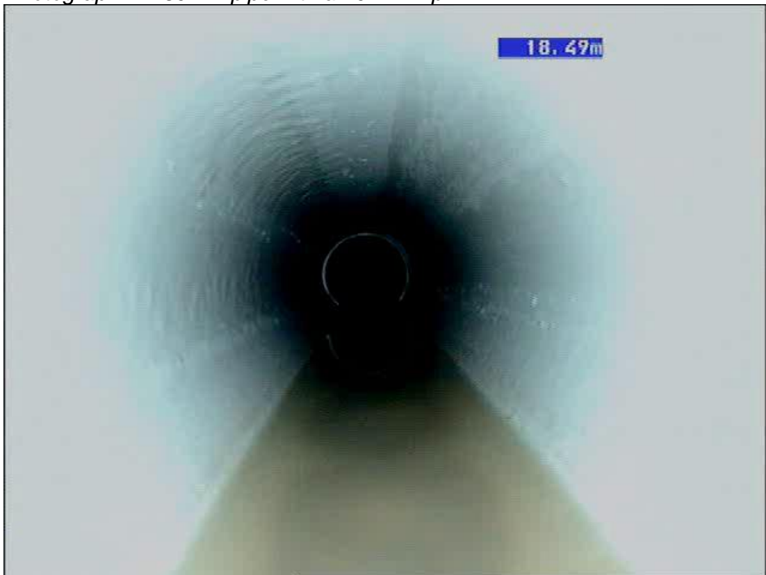
Photograph 1: 150mm pipe with a 20mm Dip
