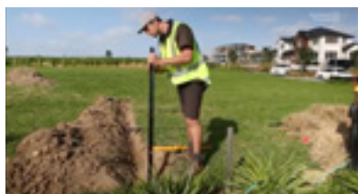
Building a silt fence and bunds 4:57
