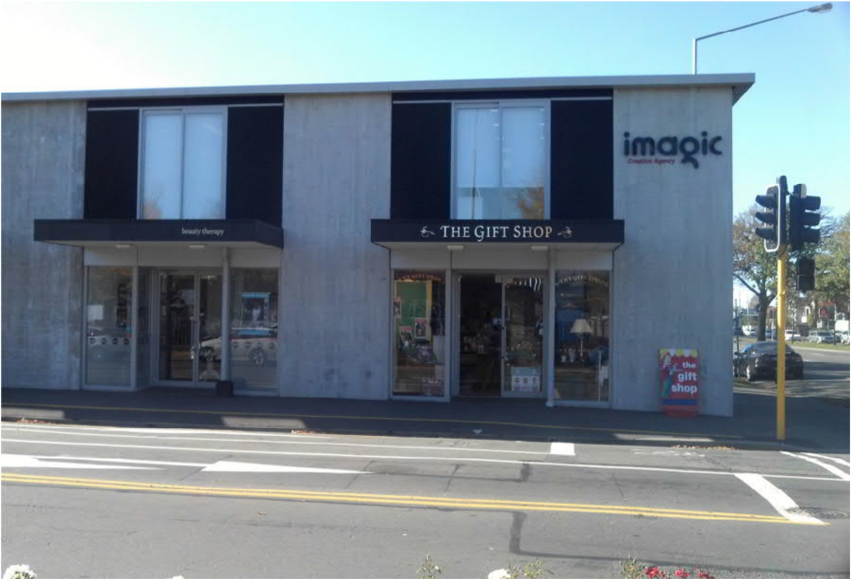
Colombo Street Looking east at Bealey Ave Intersection
