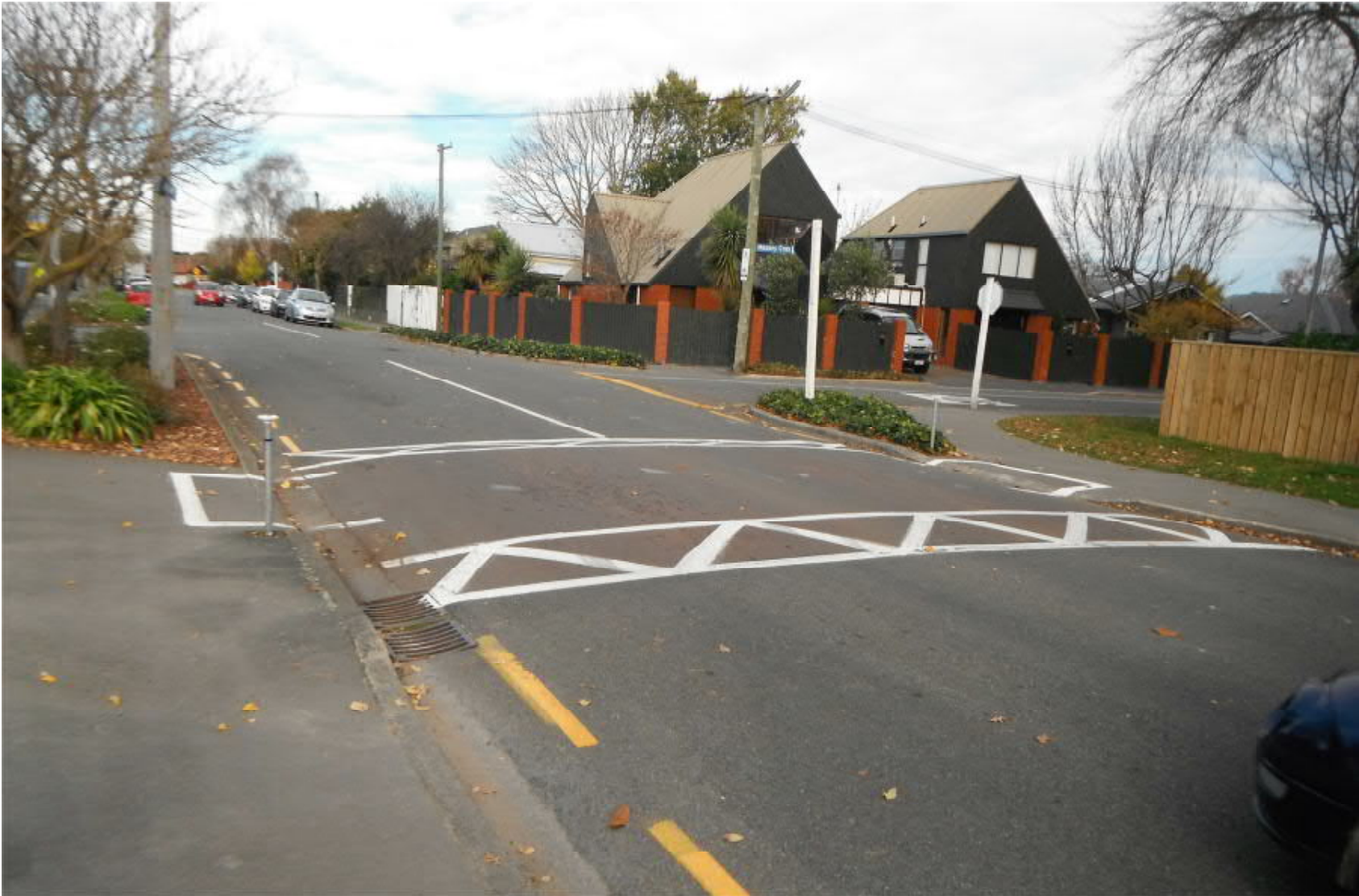
Looking south from Trafalgar Street towards Sheppard Place, Massey Cres Intersection
