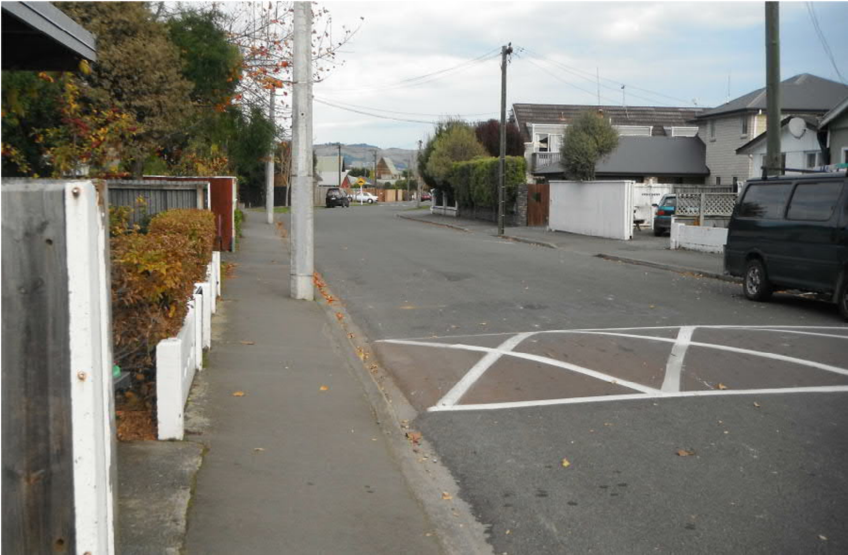
Looking south on Trafalgar St at traffic calming south of Coles Place
