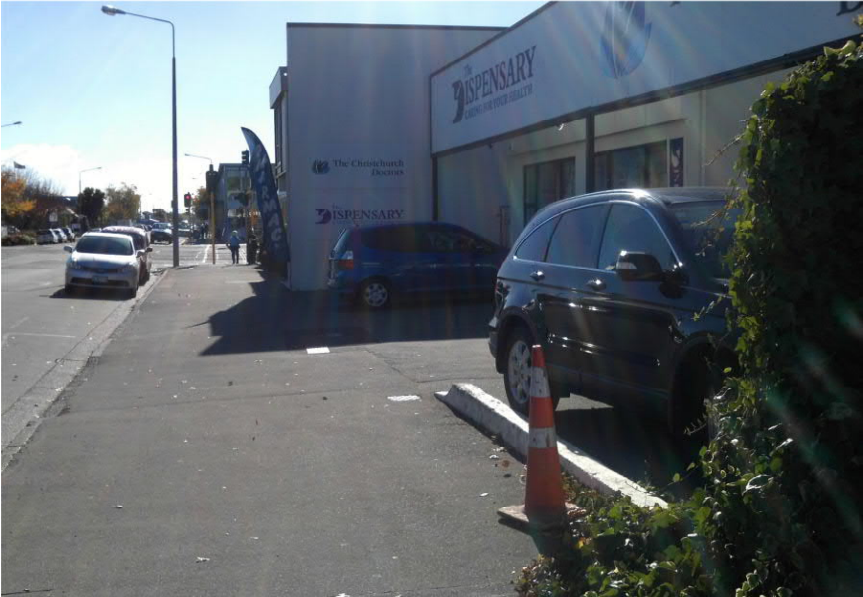
Colombo Street east looking north to Bealey Ave Intersection
