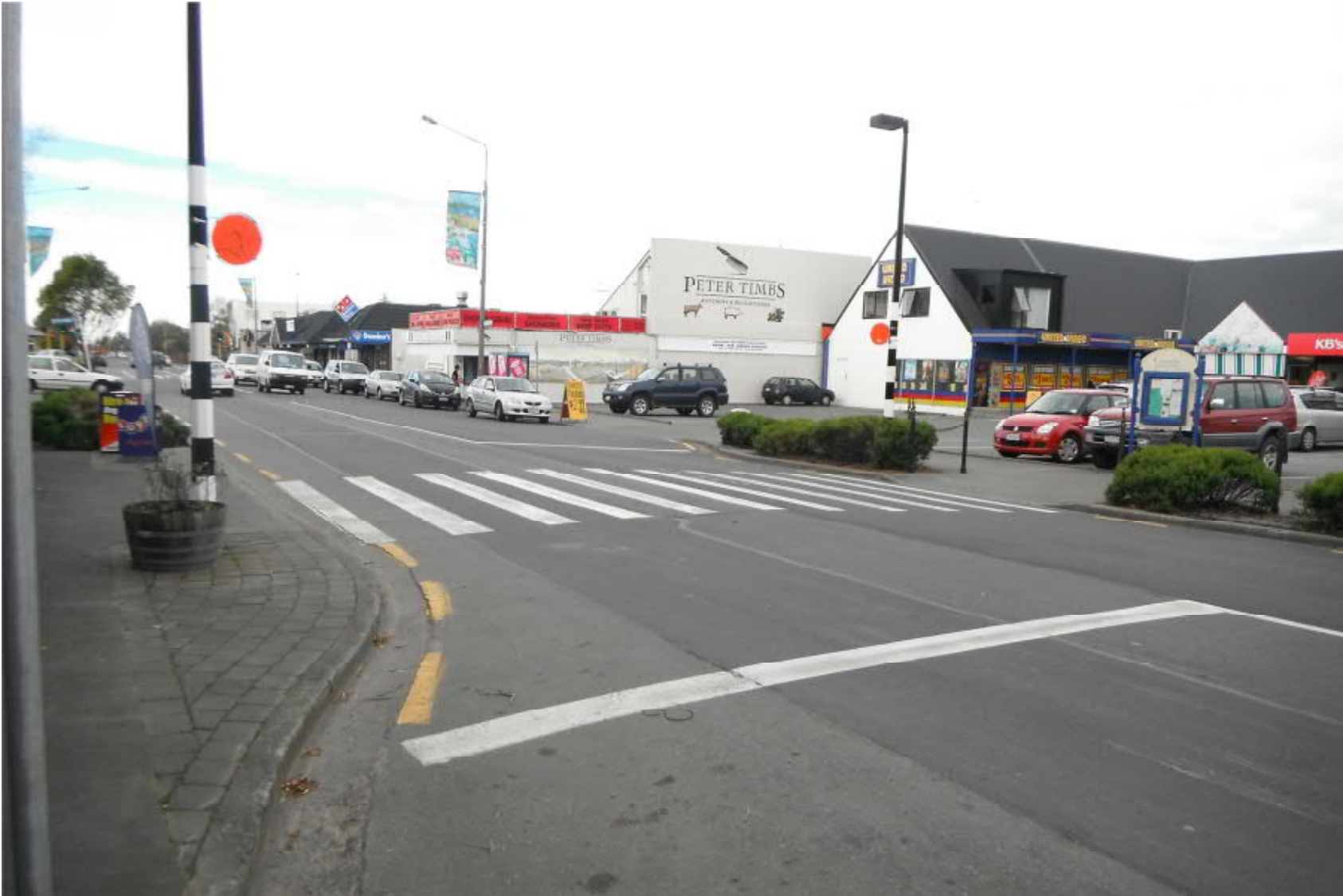
Looking east along Edgware Road at Colombo St Intersection, at existing Pedestrian Xing
