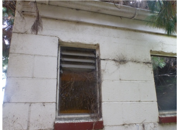
20. South Elevation – Horizontal cracks in masonry at lintel height
