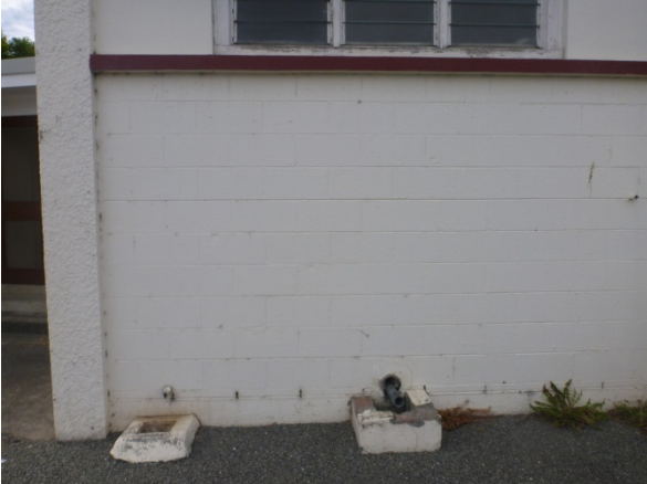
13. West Elevation – Stepped Cracks in blockwork
