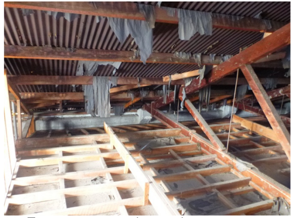
22. Truss supports and eaves beam
