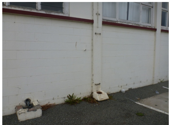
16. West Elevation – stepped cracks in masonry panels
