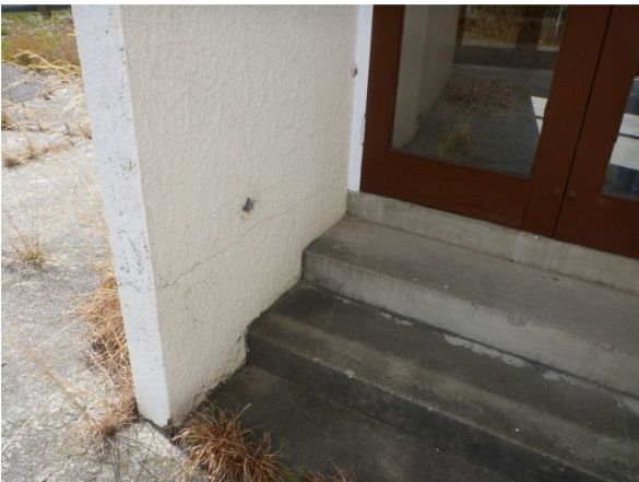
11. Wing wall at Entrance (North/West Elevation) - Horizontal cracking
