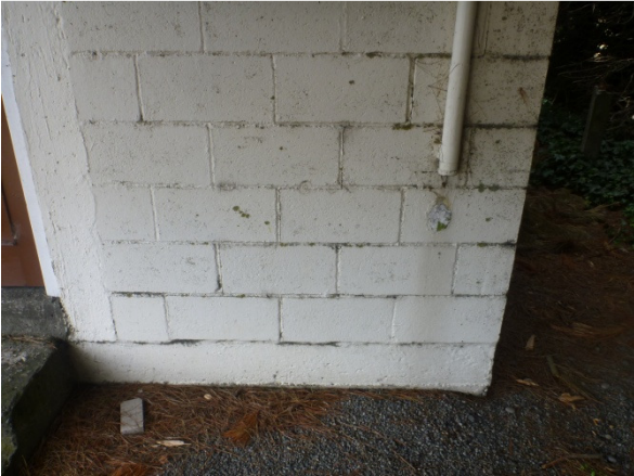
19. West Elevation – south corner – stepped crack in masonry
