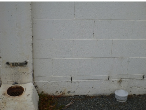
17. West Elevation - Stepped cracking in masonry wall panel
