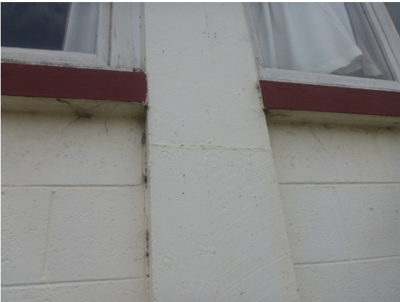
15. West Elevation – Horizontal cracks to columns at construction joint locations below windows
