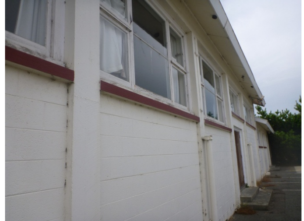
14. West Elevation – separation cracks between columns and masonry panels
