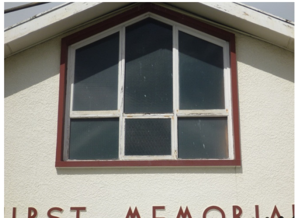
12. North Elevation – Vertical Cracks either side columns of concrete frame
