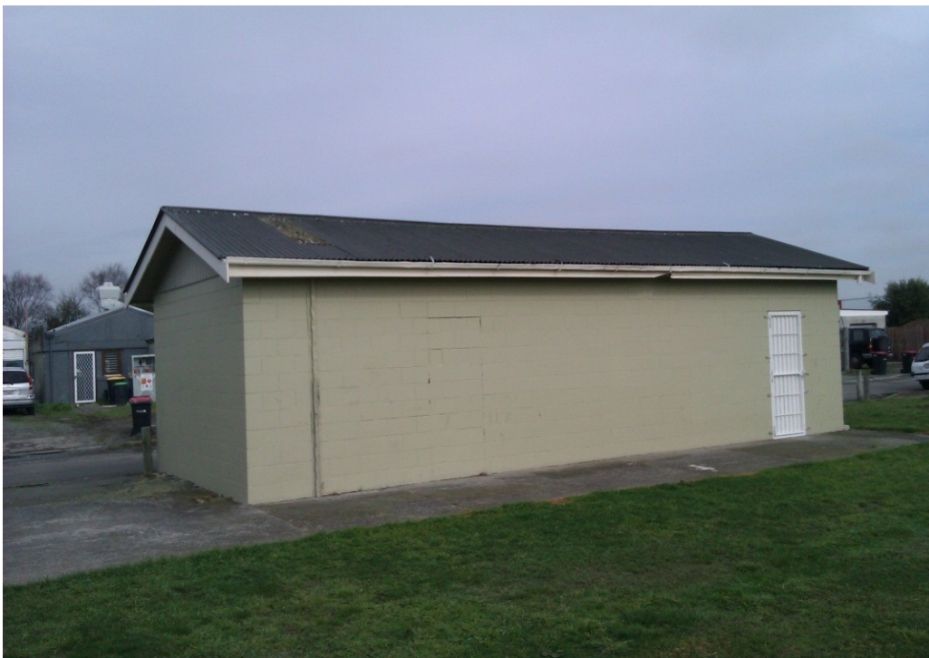
Photo 2: View of Exterior
