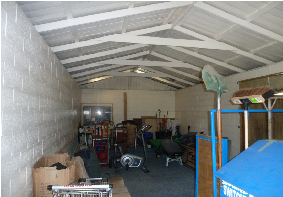
Photo 3: View of Interior
