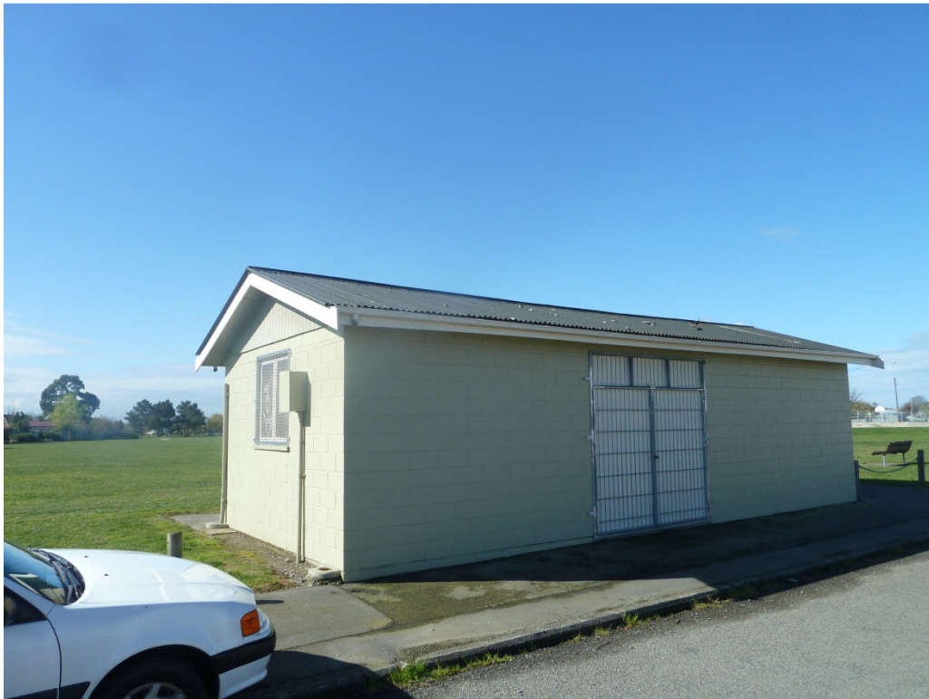
Photo 1: View of Exterior
