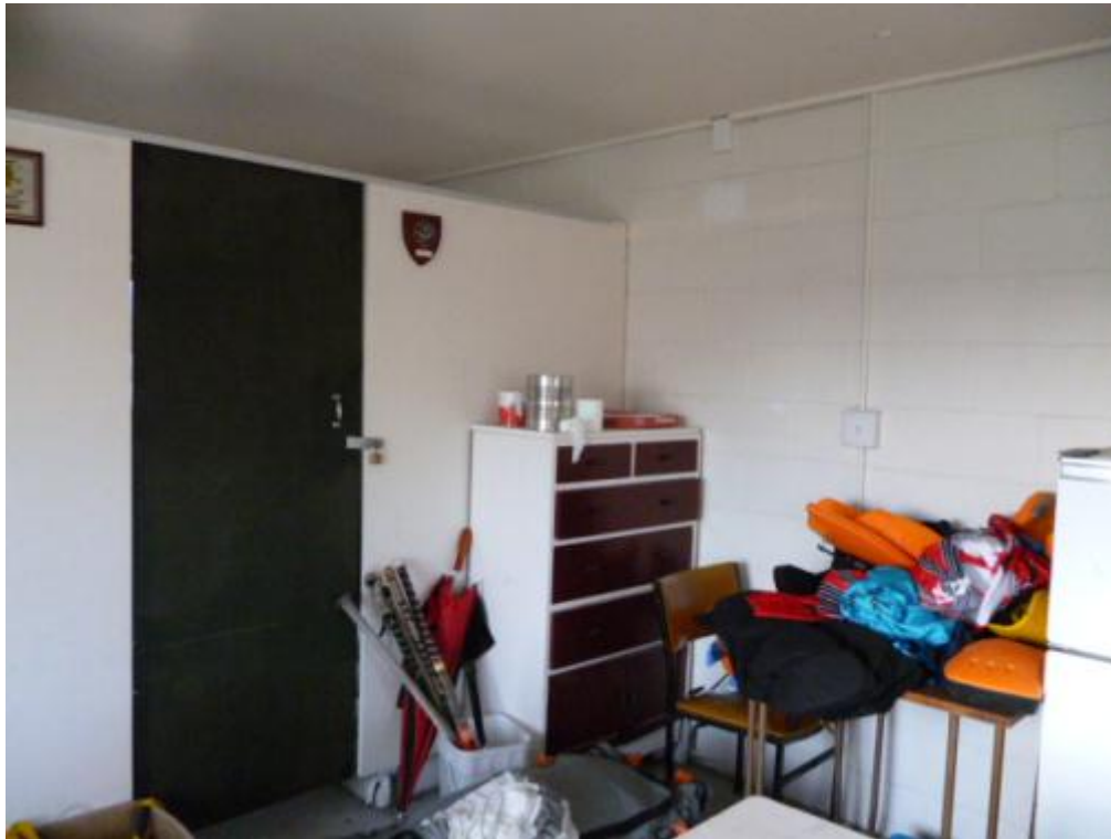
Photograph 5. Partial Height Partition.
