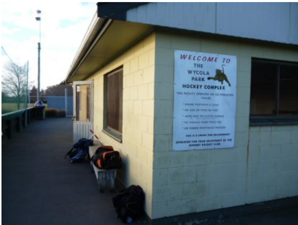
Photograph 2 View of the structure from the Southwest.
