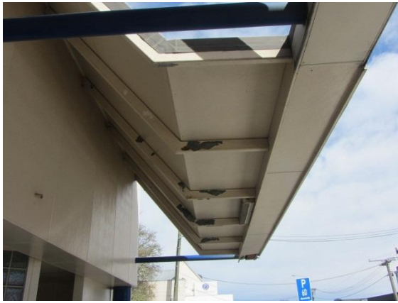
Photo 29: Paint peeling off of structural steel members supporting canopy
