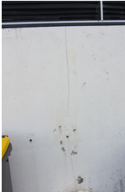
Photo 13: Detail view of cracks in Photo 10, bottom middle
