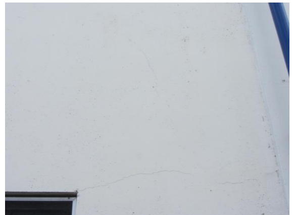
Photo 16: Detail view of cracks in Photo 10, top east corner
