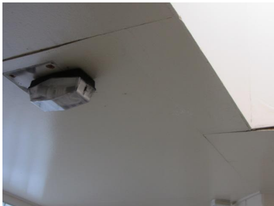
Photo 27: Sagging gib ceiling panels
