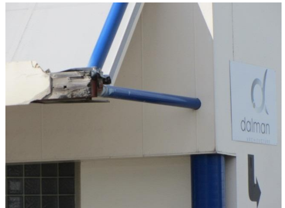
Photo 28: Cladding broken on west side of canopy
