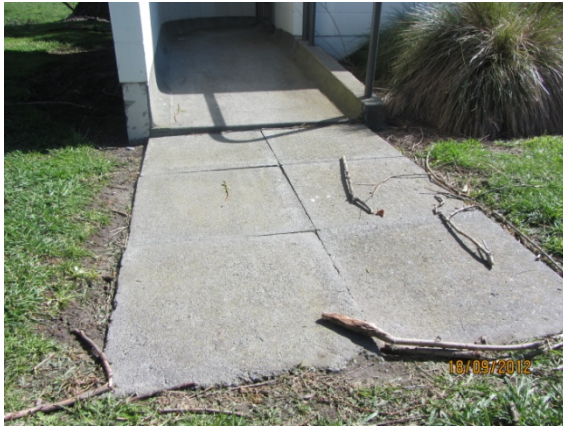
Photo 5: Pavement leading to womens toilet entrance
