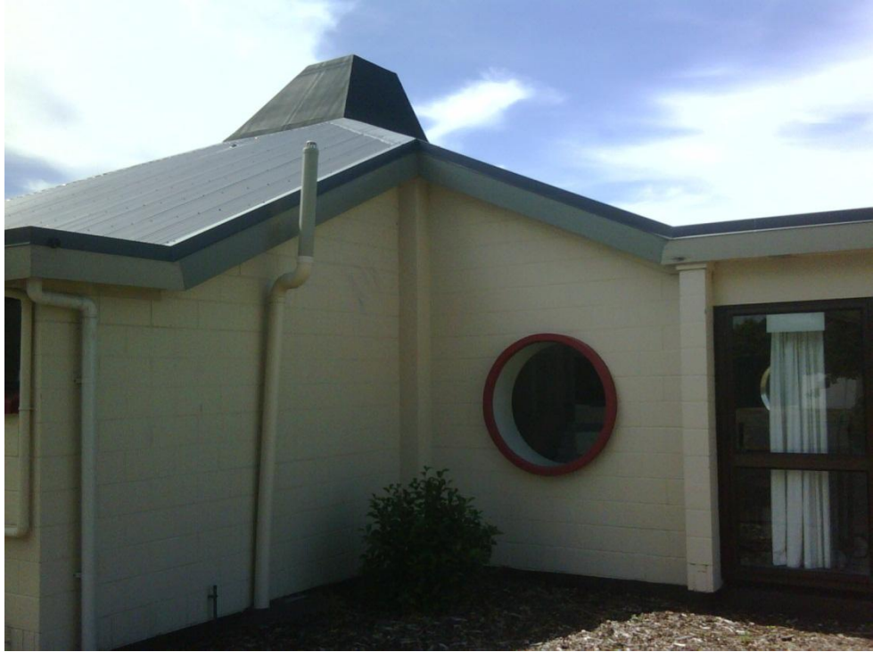
Photograph 15 External concrete masonry piers
