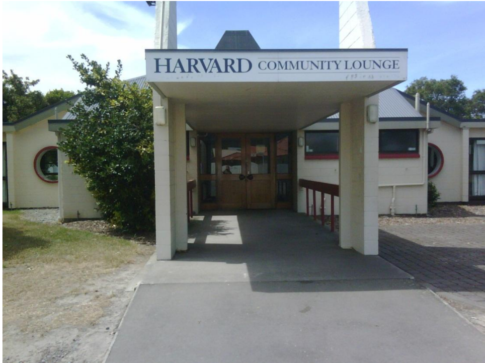
Photograph 1 View of entrance canopy.
