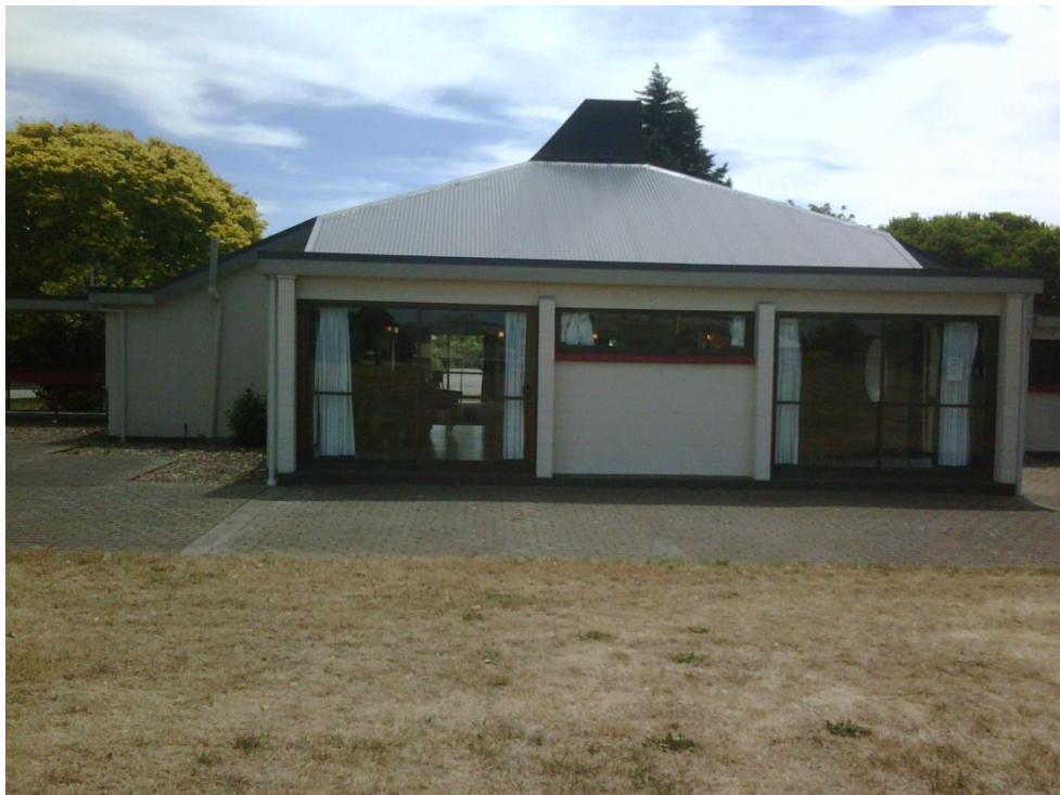
Photograph 6 View from the south.
