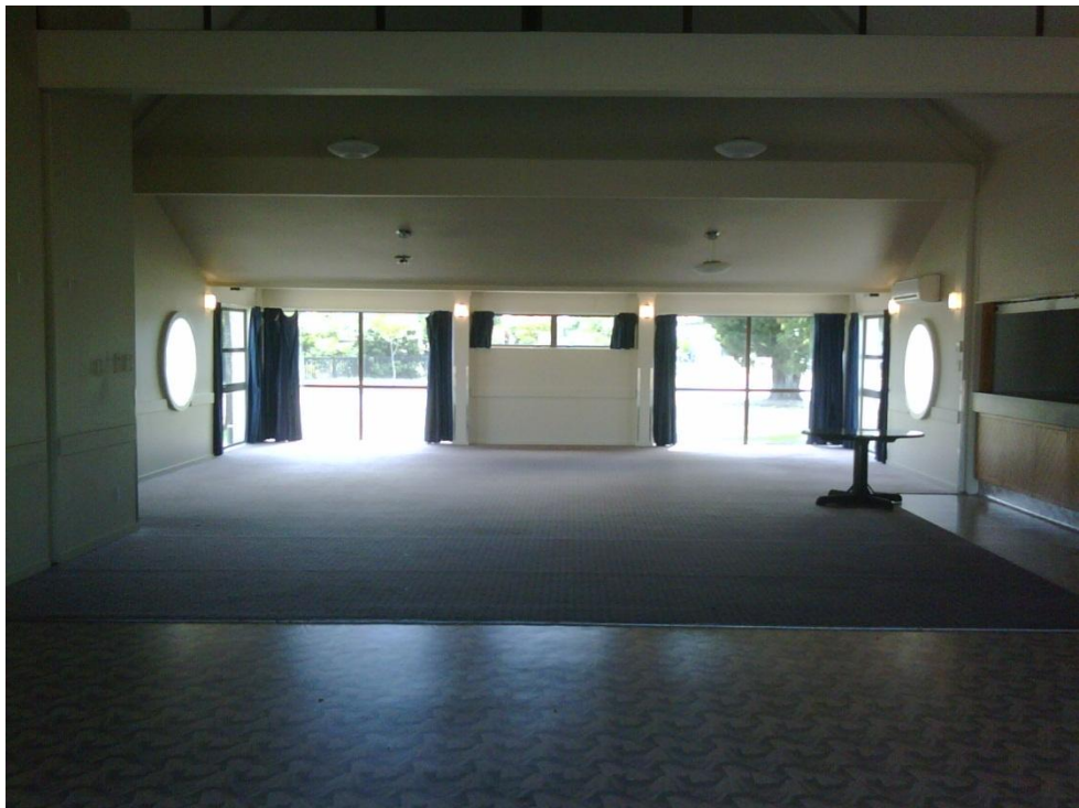
Photograph 10 Internal view of lounge area and concrete masonry piers.
