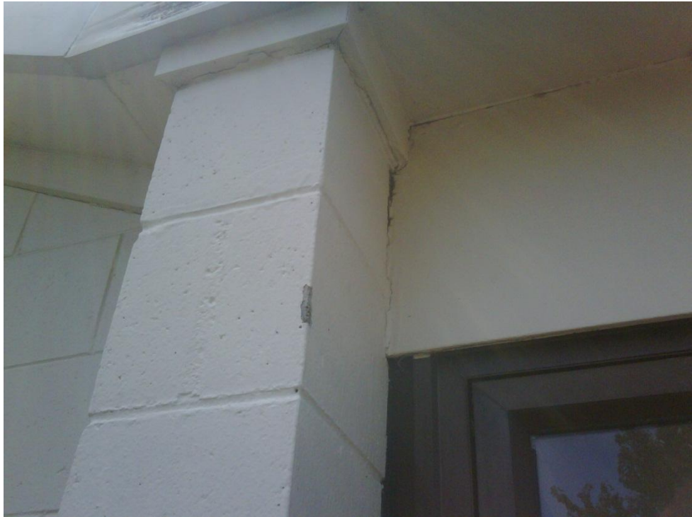
Photograph 5 Cracking between the external cladding and the top the concrete masonry piers.
