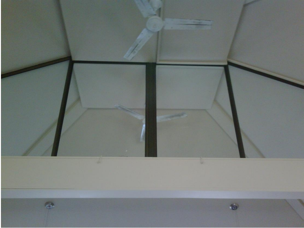
Photograph 11 Steel RHS post supporting the steel rafters.
