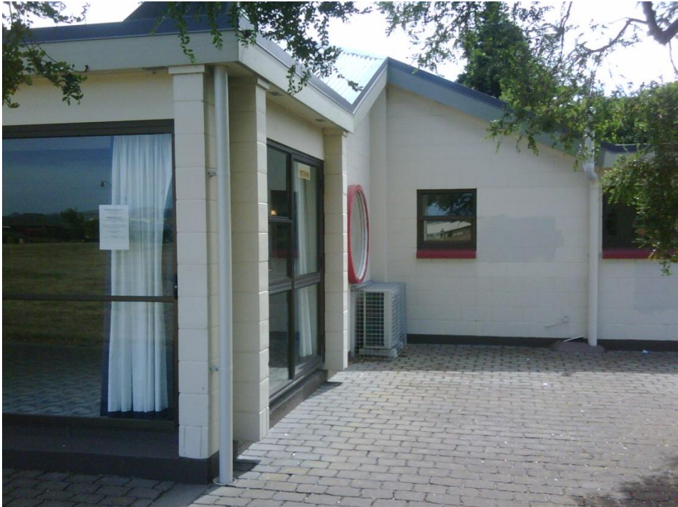
Photograph 7 External concrete masonry piers.
