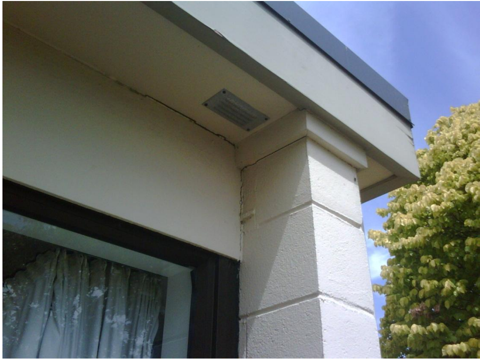
Photograph 9 Further cracking between the external cladding and the top the concrete masonry piers.
