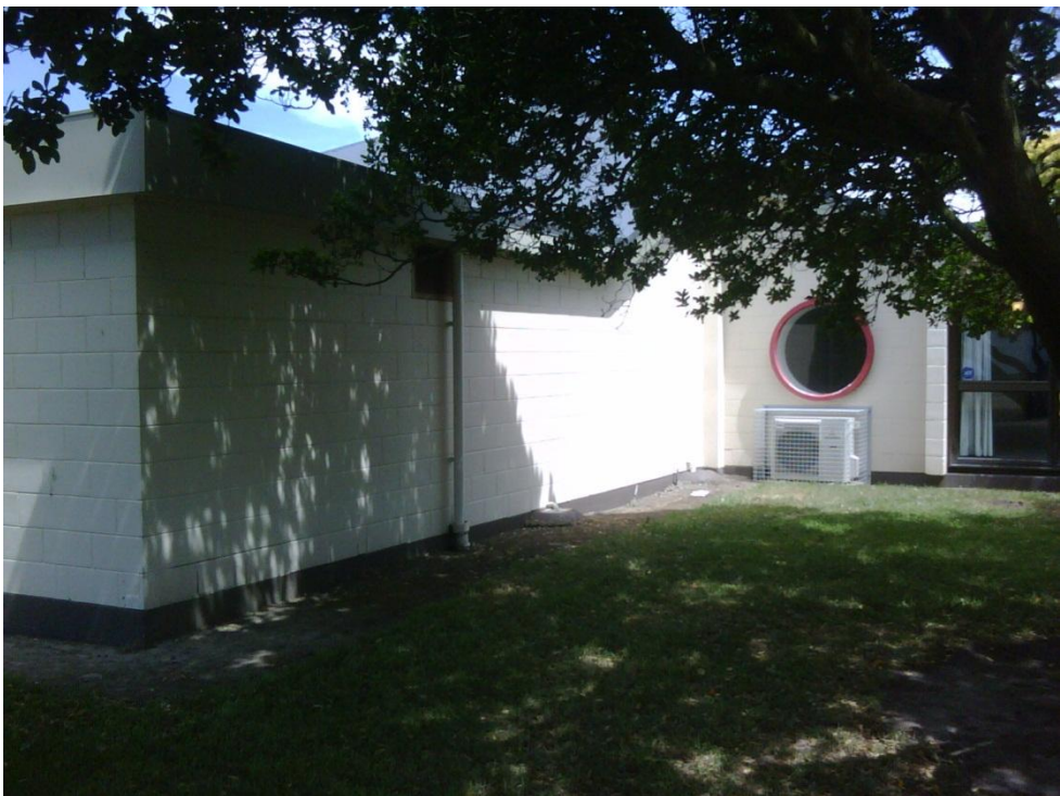
Photograph 8 Concrete masonry walls on the north-west face of the building.
