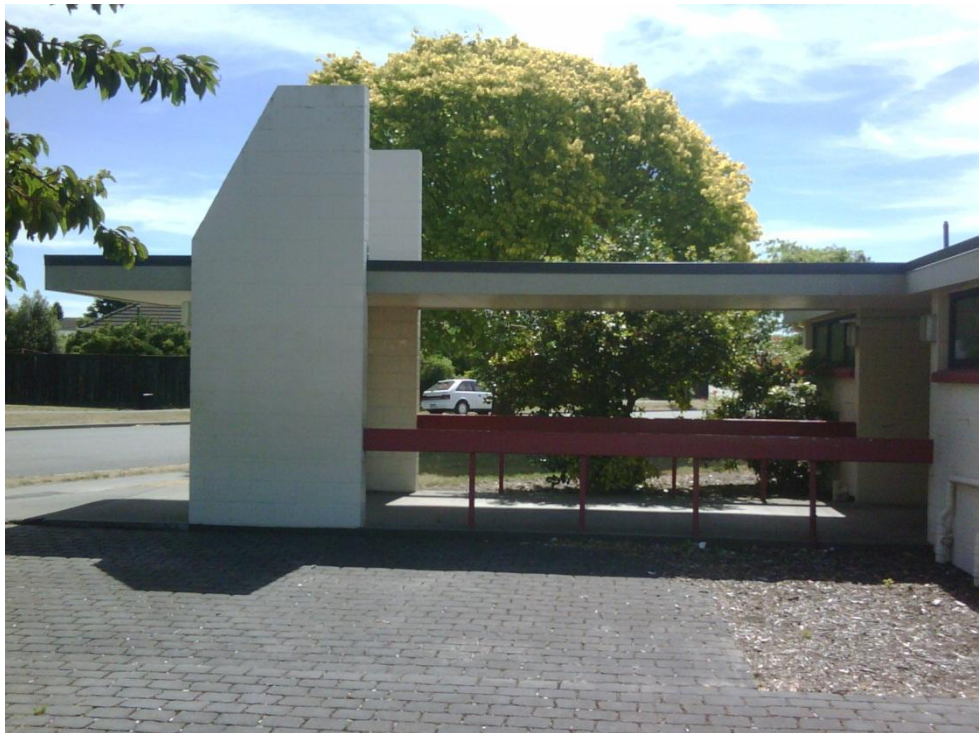
Photograph 14 View at entrance canopy
