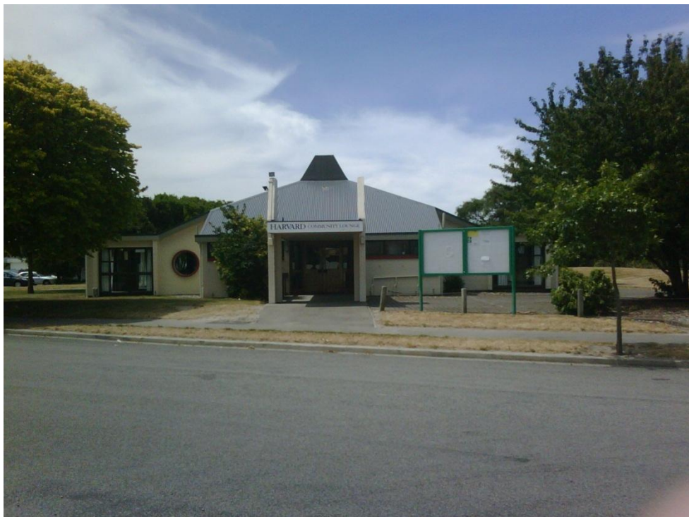
Photograph 2 View of the entrance from Corsair Drive.
