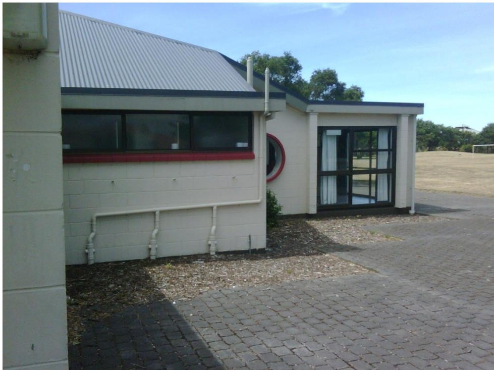
Photograph 4 View looking east.
