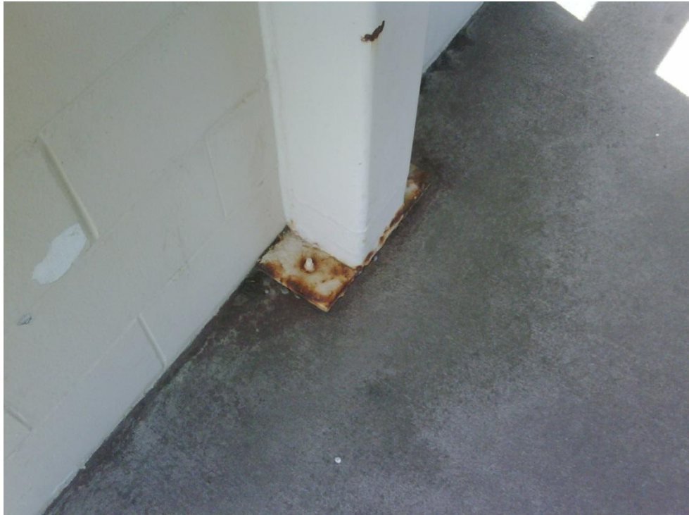
Photograph 3 Connection at base of RHS posts supporting the entrance canopy.
