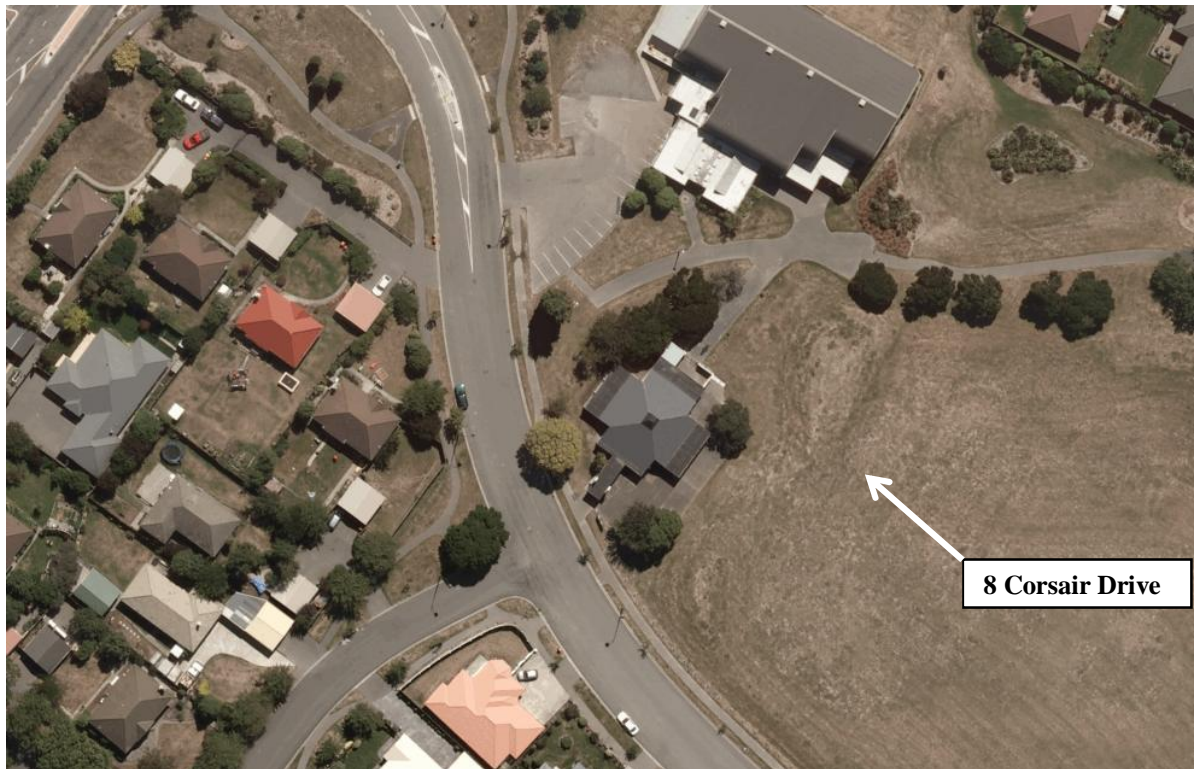
Figure 8-1 Post February 2011 Earthquake Aerial Photography 2
