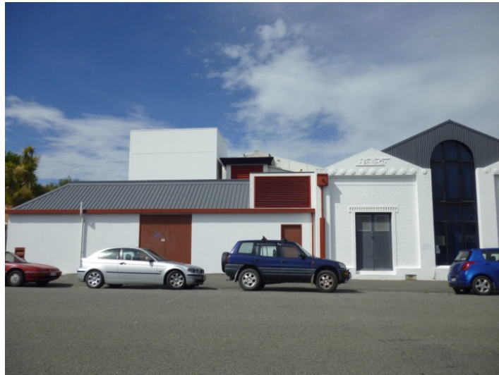
Photo 2 – North elevation (east end)
