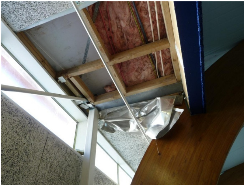
Photo 7 – View of top of steel vertical cross bracing on the western wall
