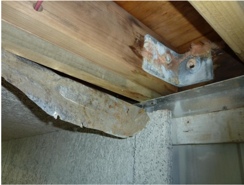
Photo 6 – Connection between eastern wall and portal frame
