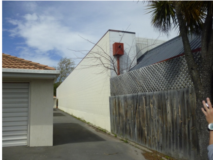
Photo 1 – Eastern perimeter wall
