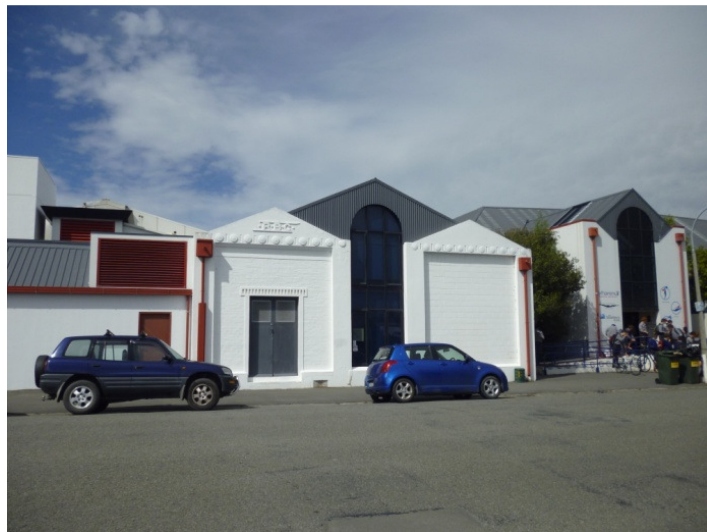
Photo 3 – North elevation (west end)
