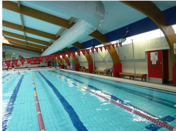
Photo 5 – Internal view of portals frames and cross bracing elements on western wall
