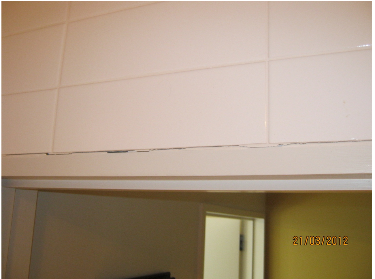
Photo 1: Crack in wall above bathroom door
