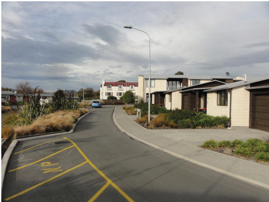
Figure 10: Heave in the pavement along the western boundary.
