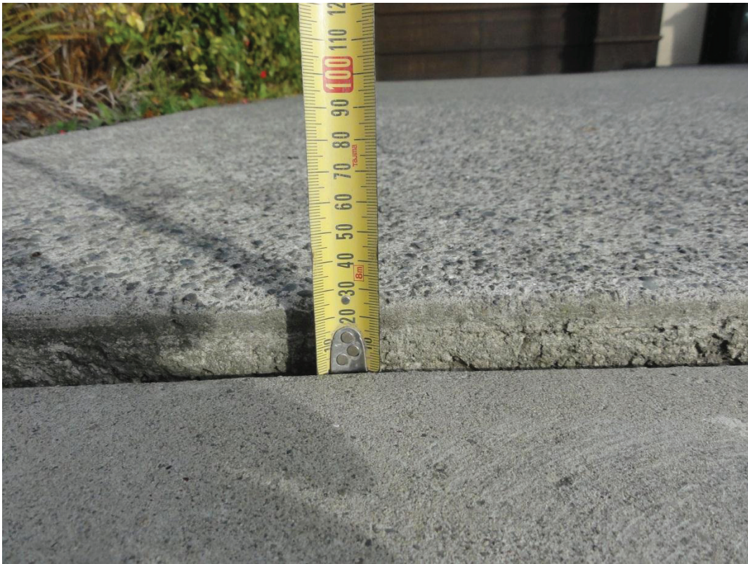
Figure 9: Approximately 20mm of vertical settlement in footpath outside Block B.
