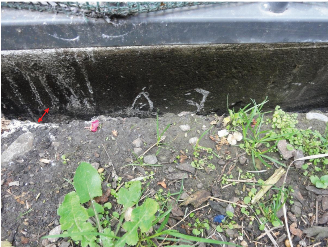
Figure 12: A gap up to 50mm is evident between a garden and concrete patio north of Block A.
