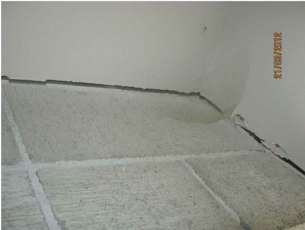
Photo 3 – Separation of timber framing from garage block wall – Unit 55
