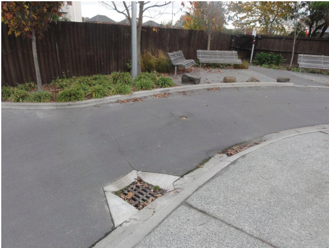
Figure 5: Up to 200mm of heave in pavement south west of Block A.
