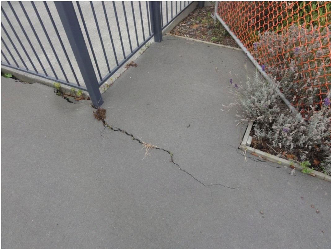
Figure 11: A gap up to 50mm is evident between the asphalt and concrete patio north of Block A.
