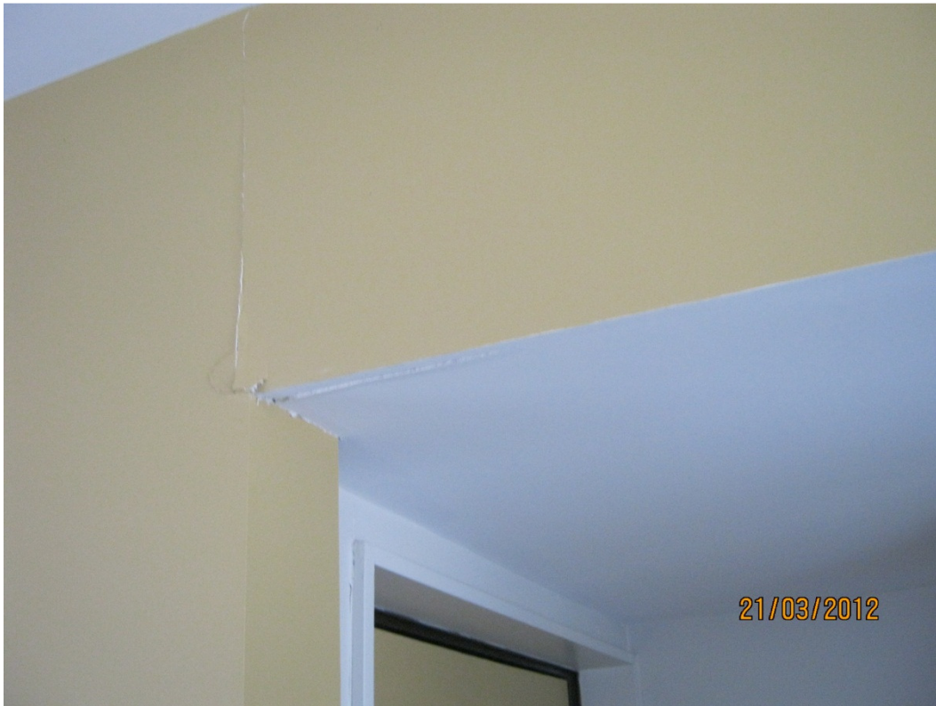
Photo 1 – Plasterboard lining cracking at wall opening.
