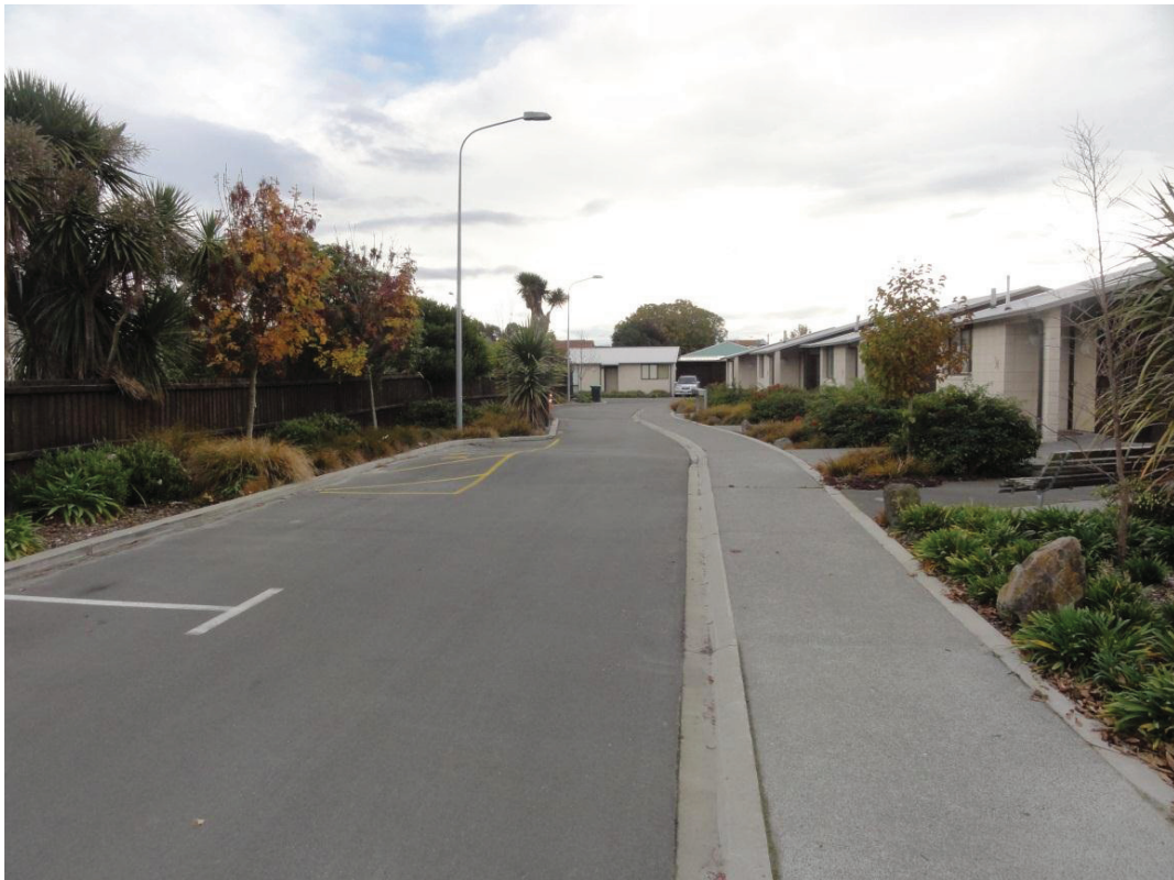
Figure 6: Up to 300mm of heave in the pavement along the western boundary.
