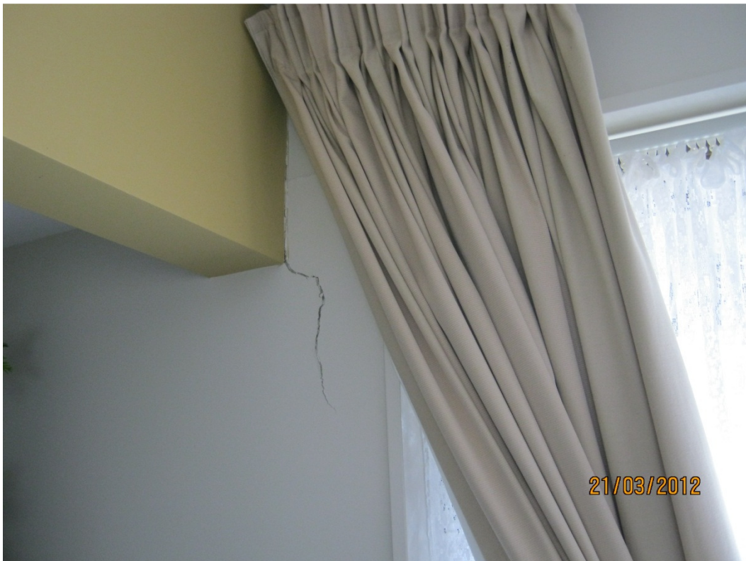
Photo 2 – Wall crack at roof beam and lintel junction
