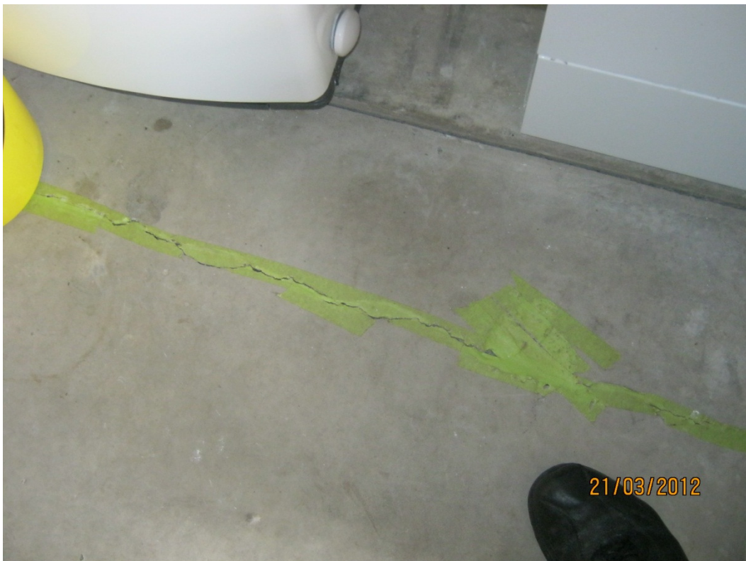
Photo 4 – Crack in garage floor slab
