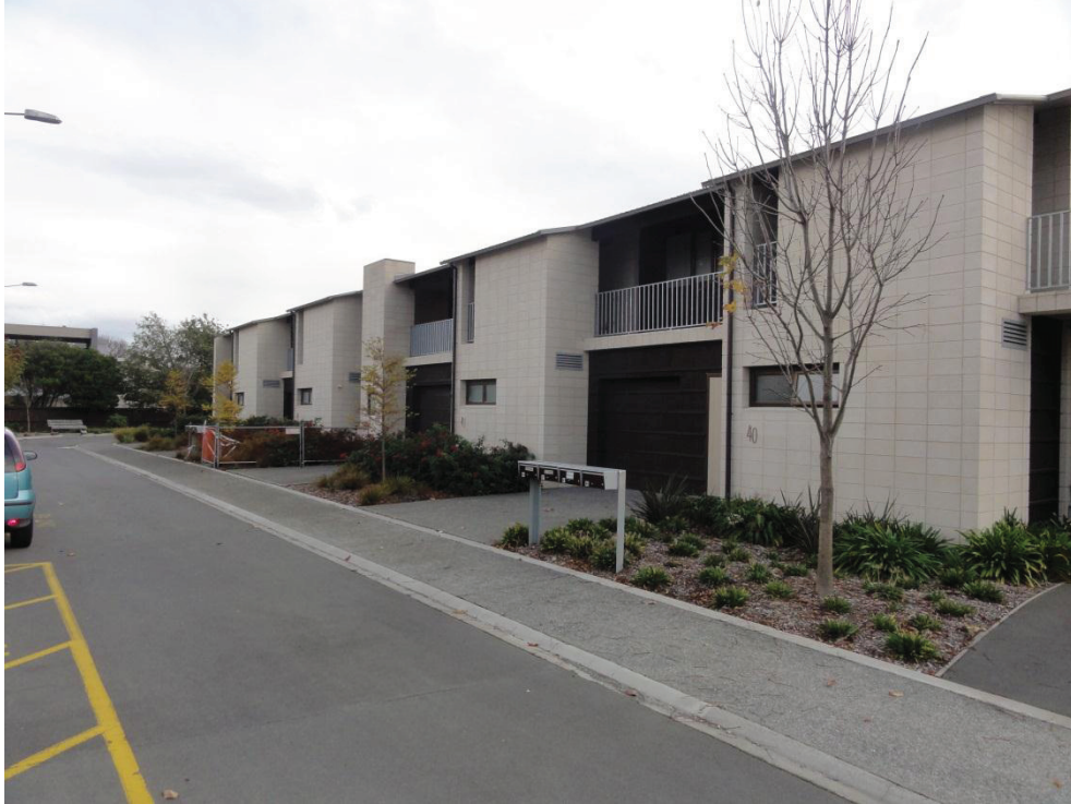
Figure 1: South elevation of Block A.
