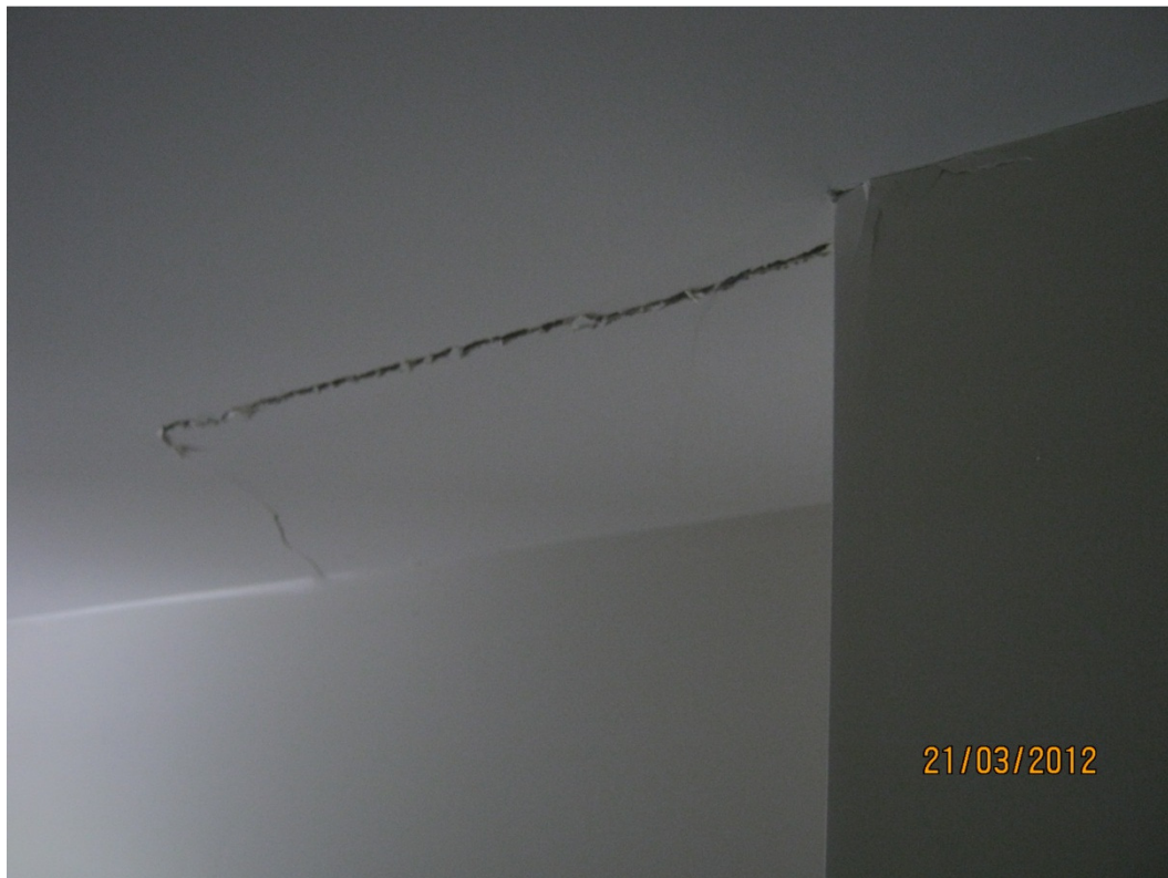
Photo 3 – Crack in ceiling lining
