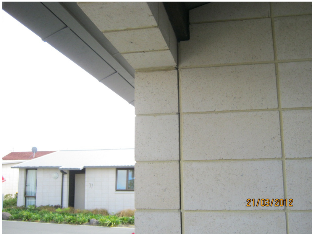
Photo 1 – Block veneer supporting block lintel and veneer separation at entry
