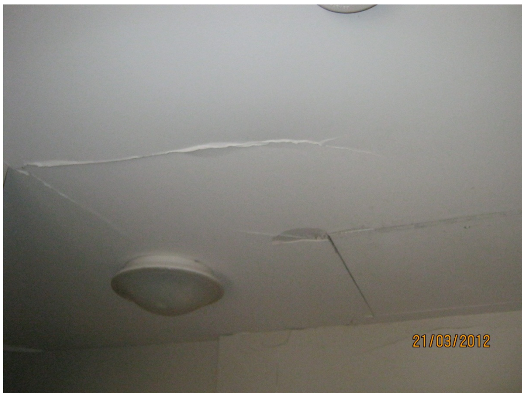
Photo 4 –Cracking to ceiling and wall linings
