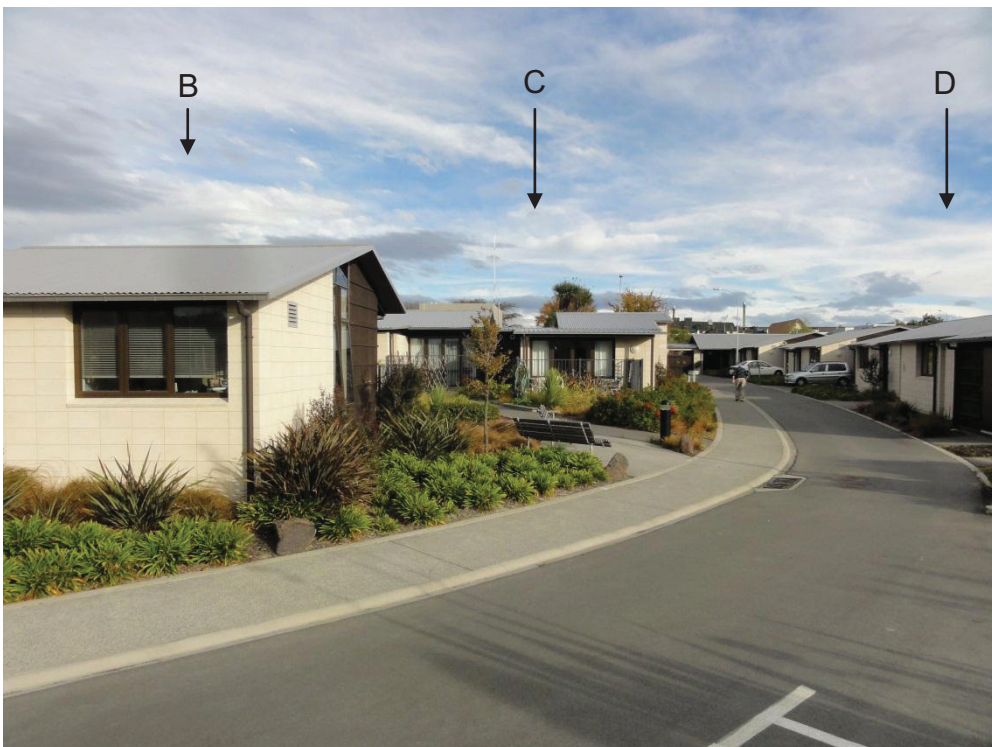
Figure 2: East elevation of Block B, C and D.
