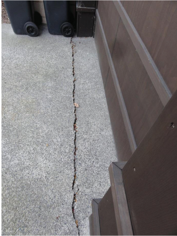
Figure 3: Up to 10mm lateral and 20mm of vertical movement.
