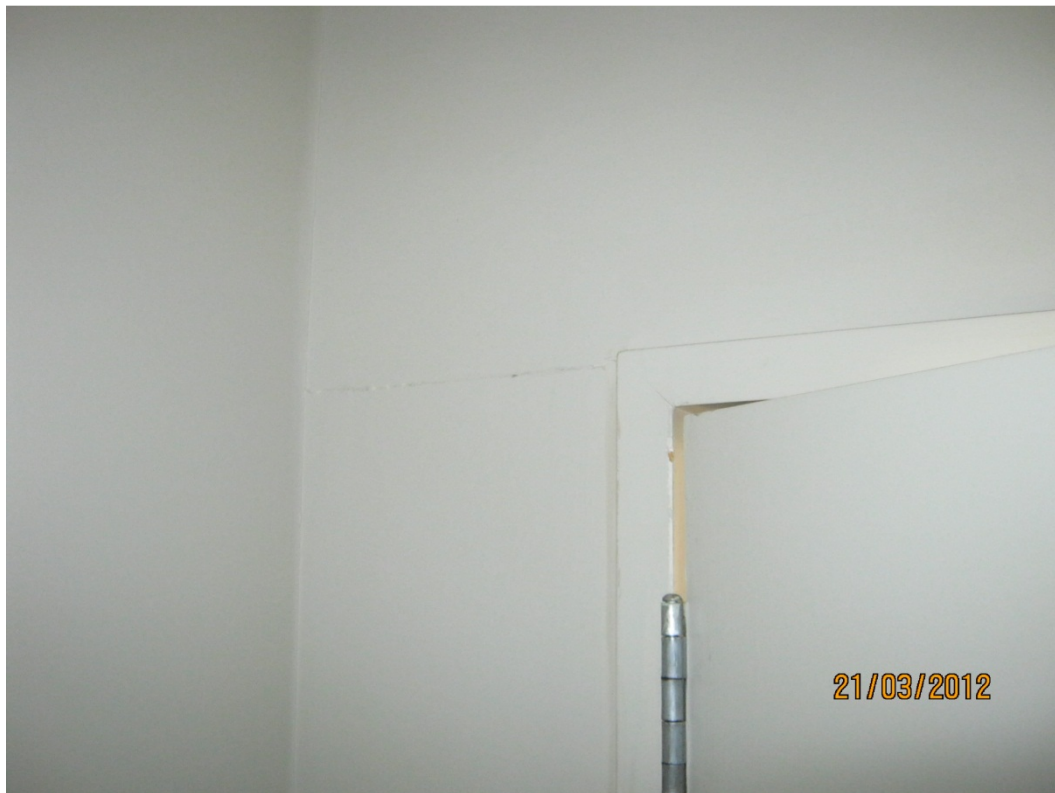
Photo 6 – Crack in wall lining at door opening
