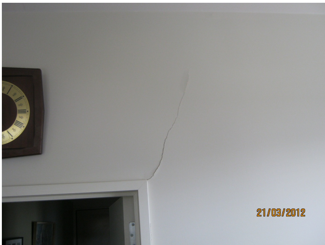
Photo 7 – Crack in wall lining at door openings
