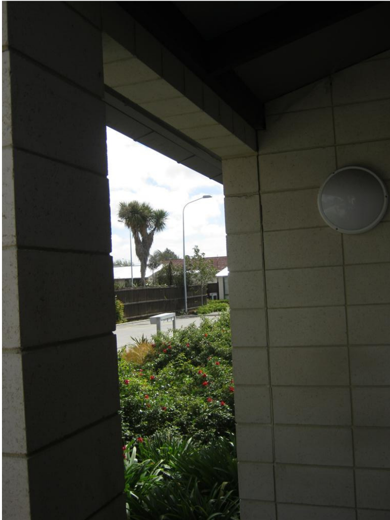
Photo 2 – Block lintel on veneer / separation of veneer at entry
