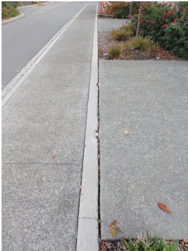
Figure 4: Up to 30mm of lateral movement.
