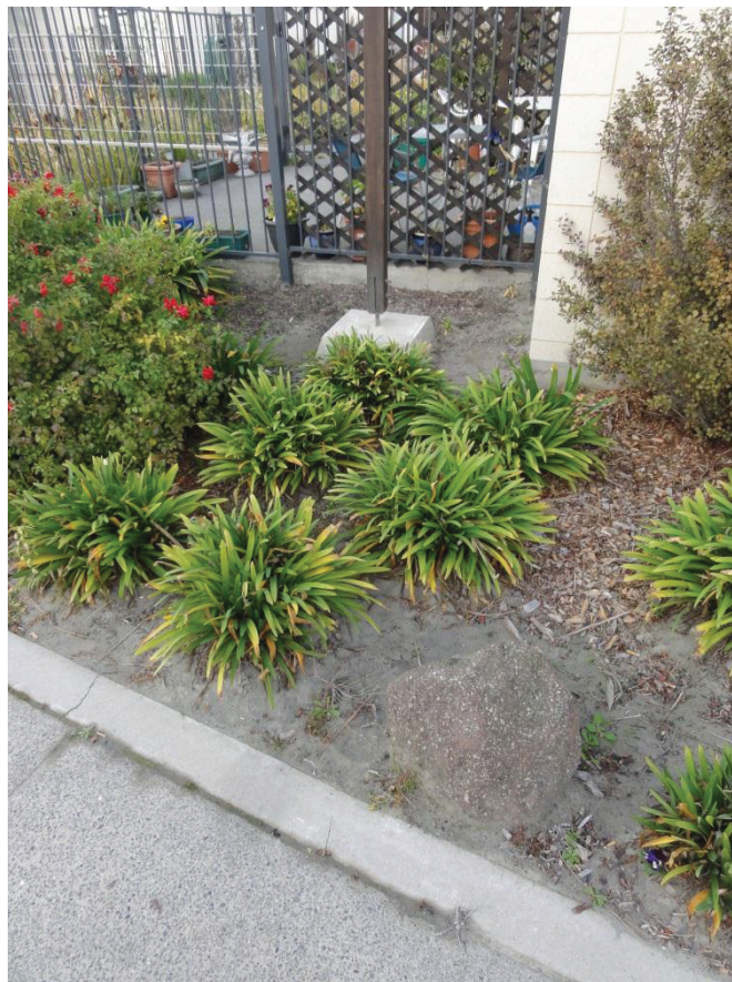
Figure 8: Liquefaction ejected material is evident in gardens around the site.
