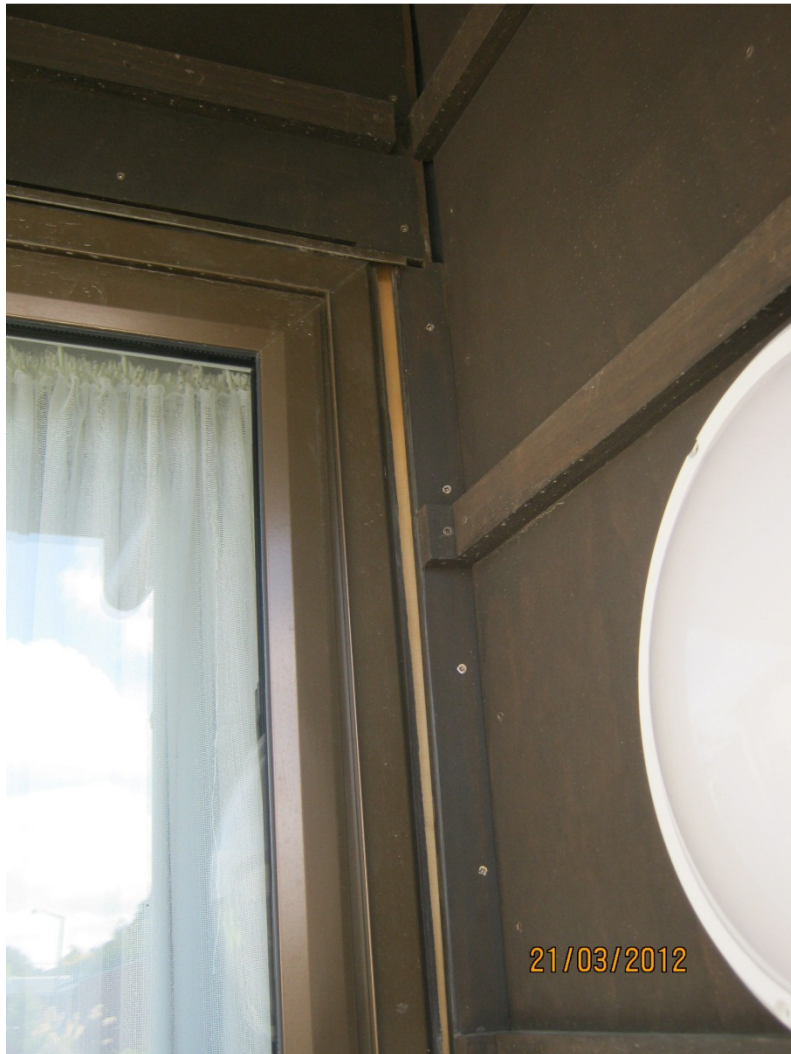
Photo 5 - Separation of wall framing and window frame
