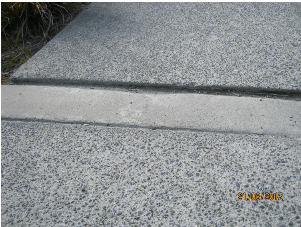
Photo 9 – Differential settlement or heave in patio slab
