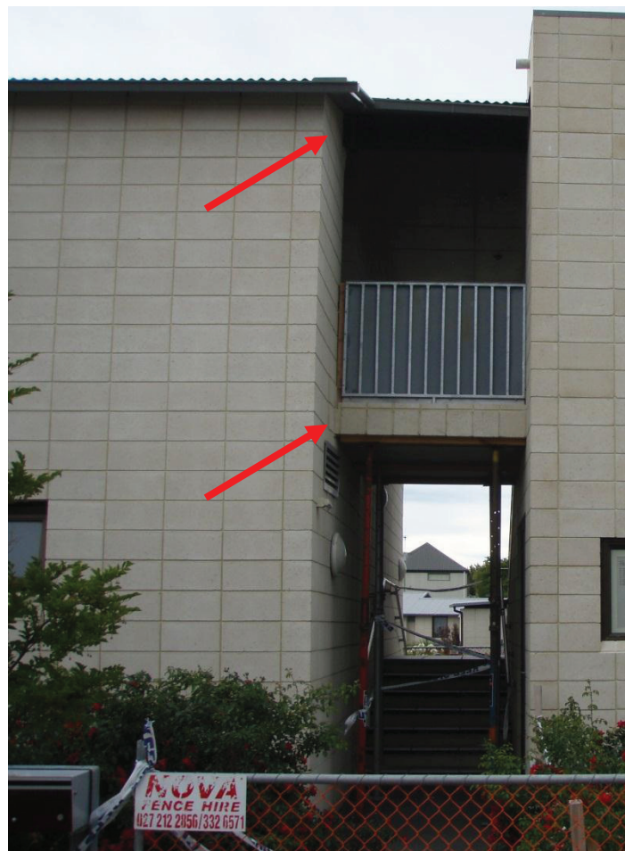
Figure 14: Separation between west side of Block A and the stair well.
