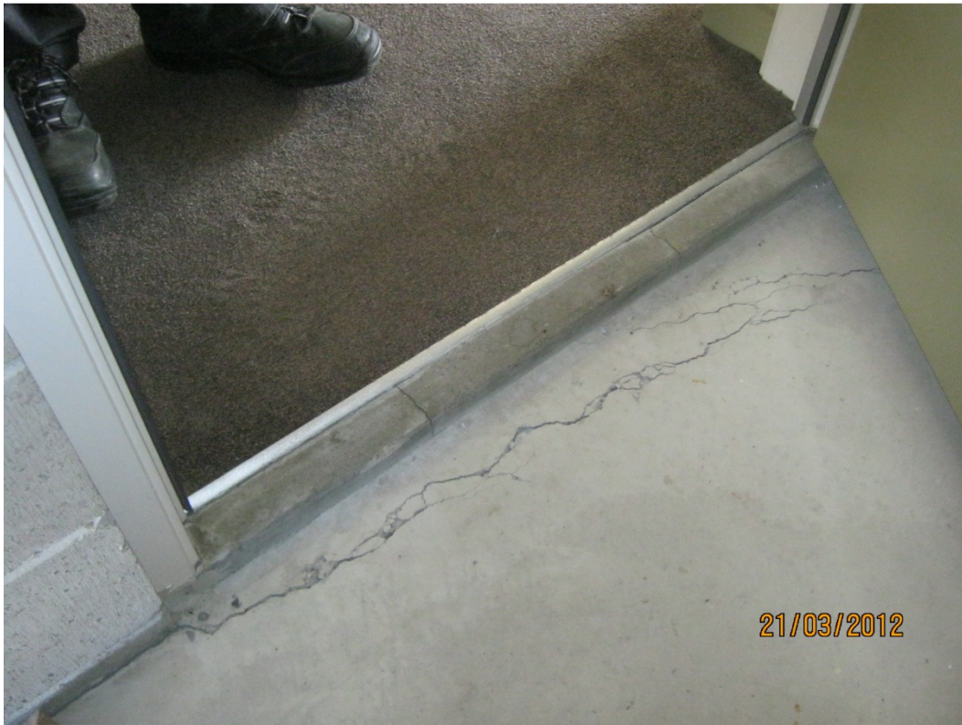
Photo 8 – Crack in garage floor
