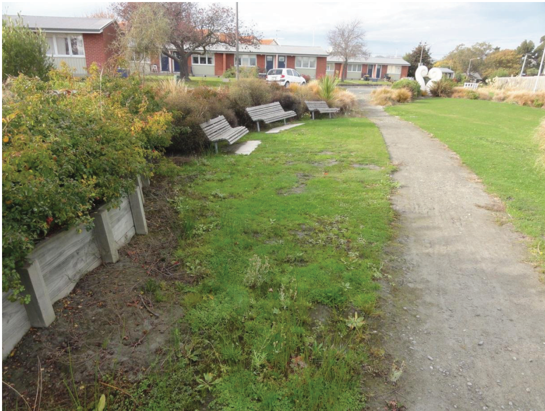
Figure 13: Liquefaction induced settlement of the park benches east of the site.
