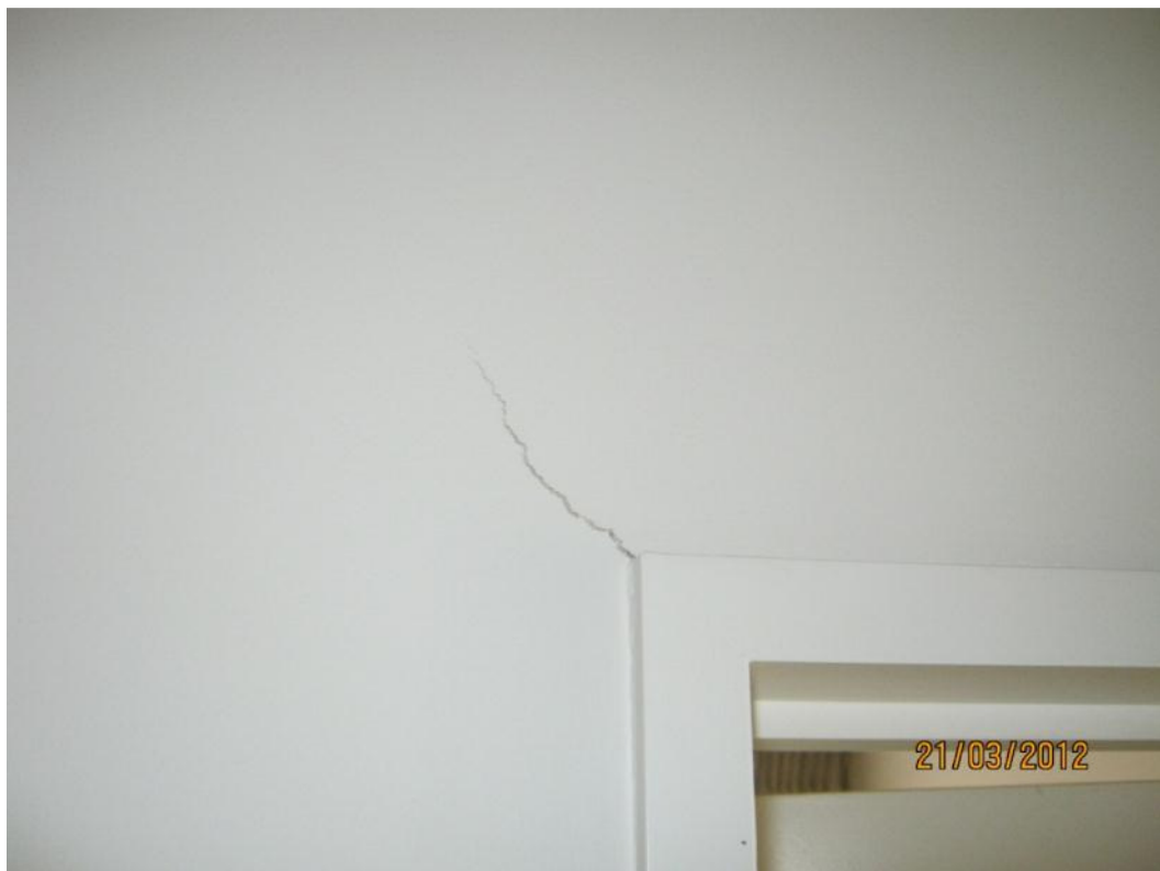
Photo 2: Crack in wall over bedroom doors.
