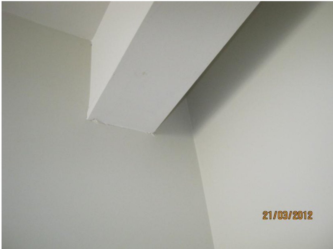
Photo 1: Crack in Unit 50 wall – beam joint.
