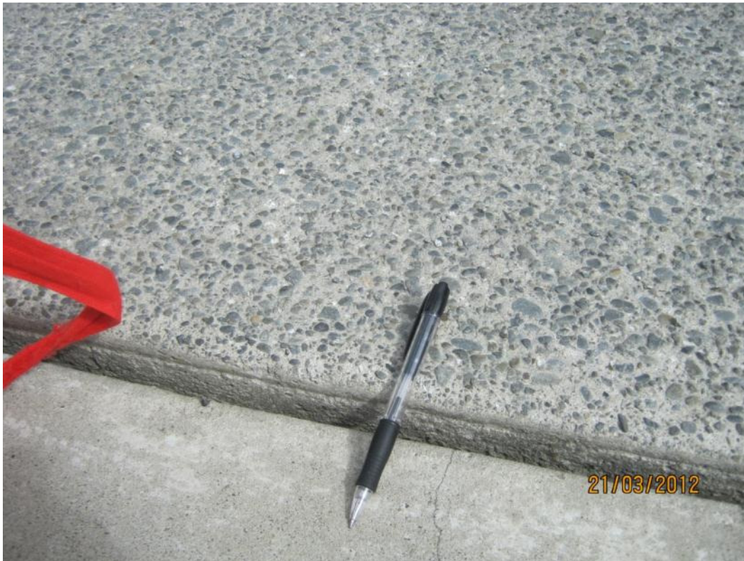
Photo 3: Separation and settlement of patio slab.
