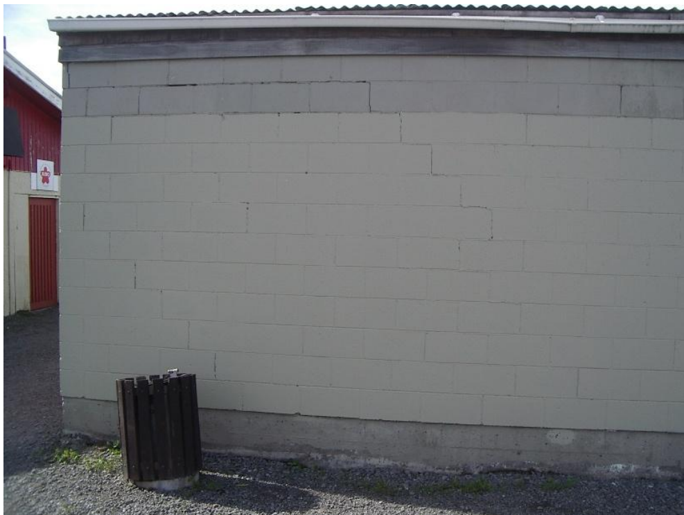
■ Figure 7 Observed cracks in the Westminster Street community building
