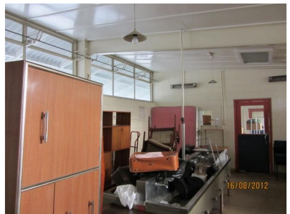
Photo 14: Interior view of the east partition (2)
