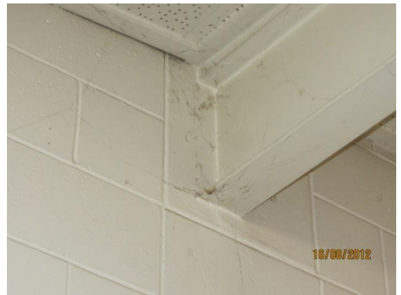
Photo 12: View of the beam and wall connection
