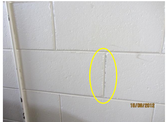
Photo 16: Close up view of one of the interior masonry walls in the east partition, showing location of crack (2)
