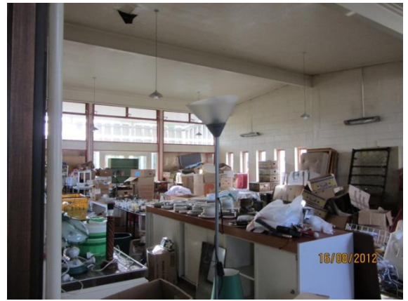
Photo 10: Opening in the east end of the building (1)
