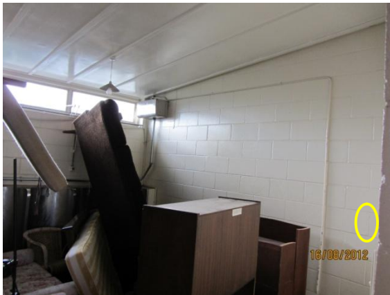
Photo 15: View of one of the interior masonry walls in the east partition, showing location of crack (1)
