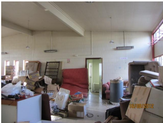
Photo 11: Opening in the east end of the building (2)
