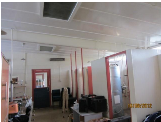
Photo 13: Interior view of the east partition (1)
