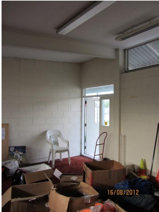
Photo 5: View of the partition wall with the portal frame and the concrete encased column
