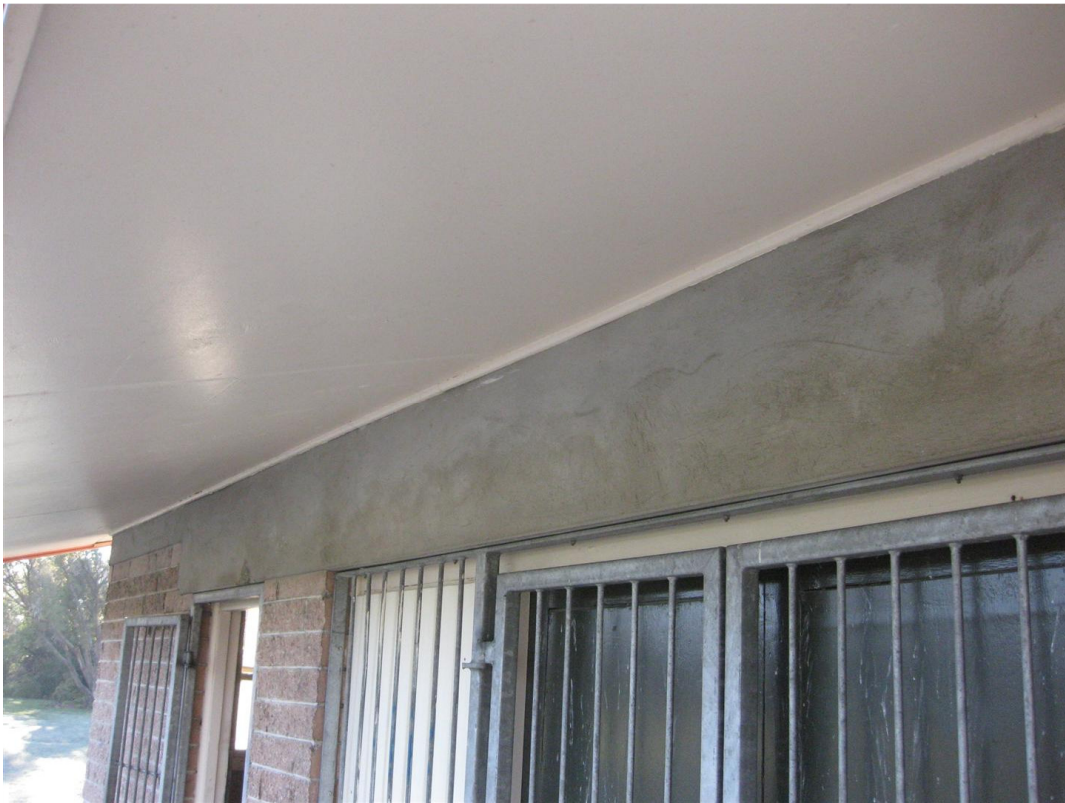
Photo 5: Front wall lintel
