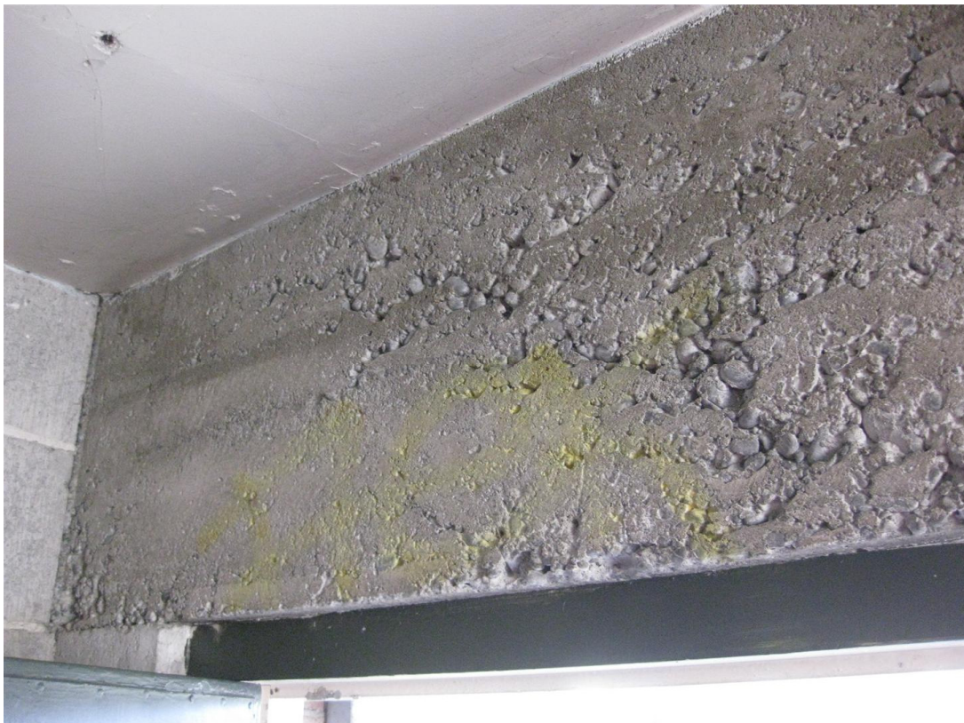
Photo 8: Front wall lintel
