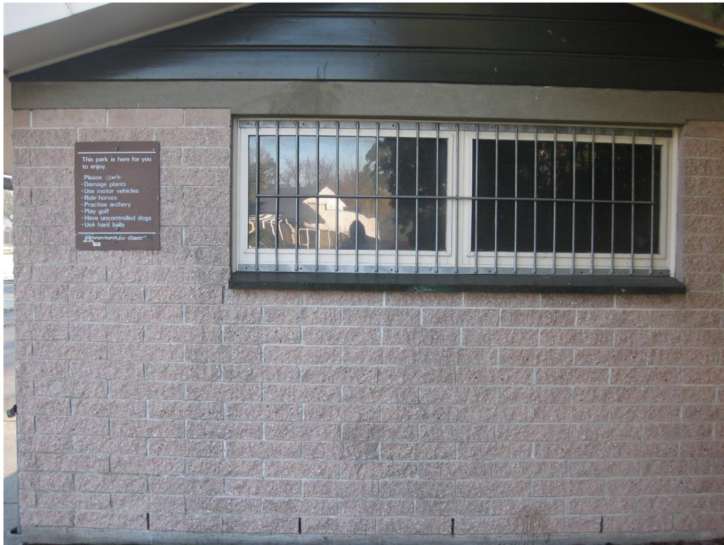
Photo 3: Right side wall
