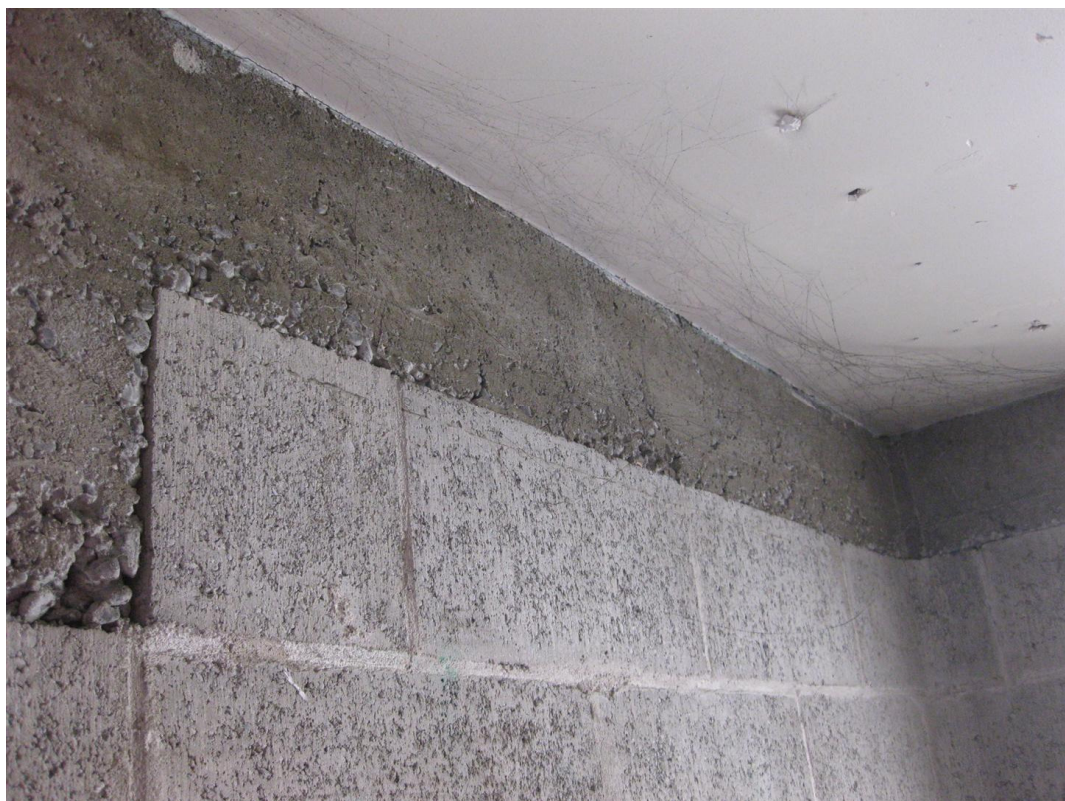
Photo 6: Internal wall, bond beam and ceiling
