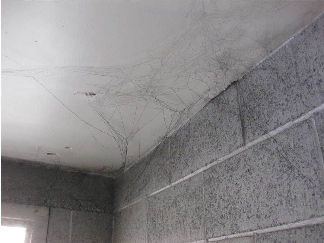
Photo 7: Internal wall, bond beam and ceiling
