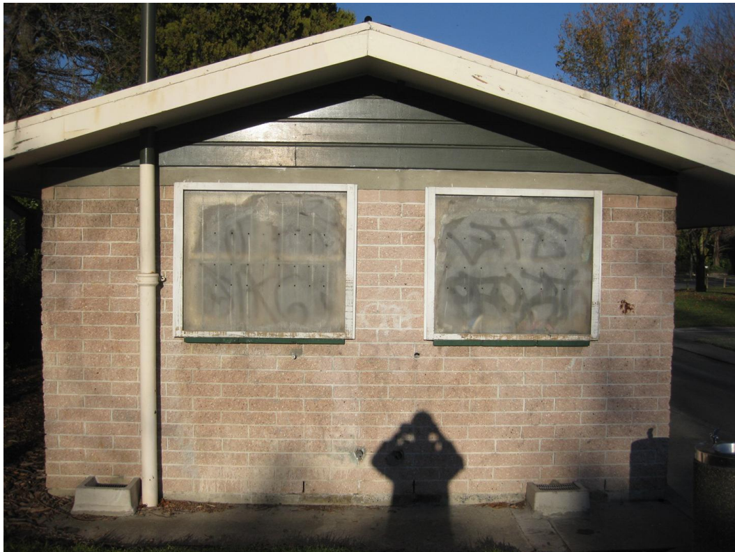
Photo 2: View of the building from left side
