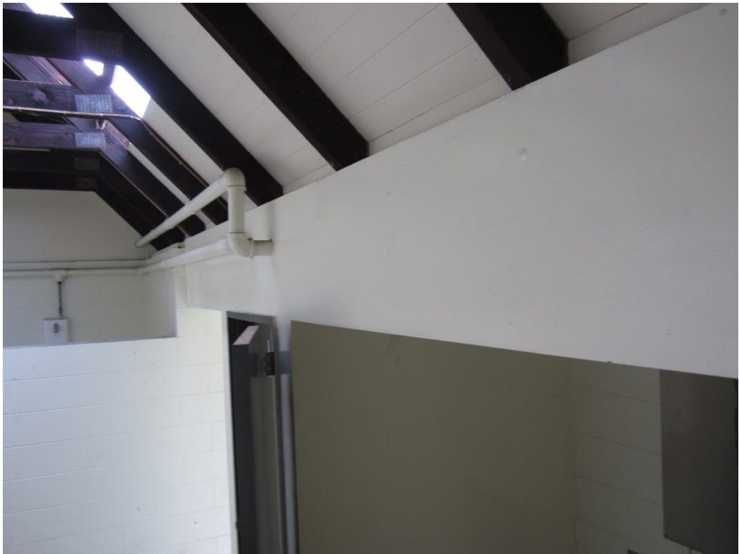
Photograph 5 Unrestrained concrete masonry shower partition walls
