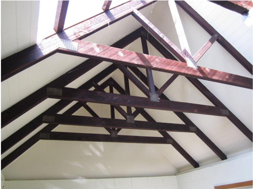
Photograph 1 Nail plate timber trusses
