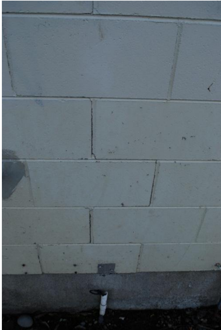
Photograph 9 Minor step cracking in the mortar on the south-eastern elevation of the building
