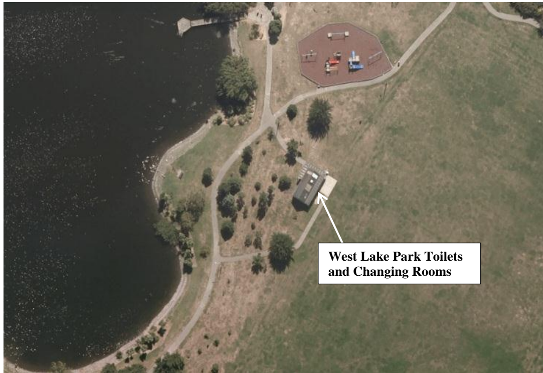
Figure 4 Post February 2011 Earthquake Aerial Photography 3
