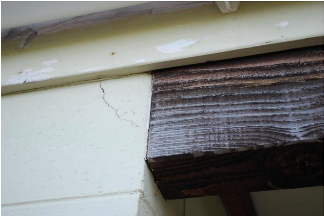
Photograph 8 Cracking in the concrete masonry unit at connection with an external timber roof beam
