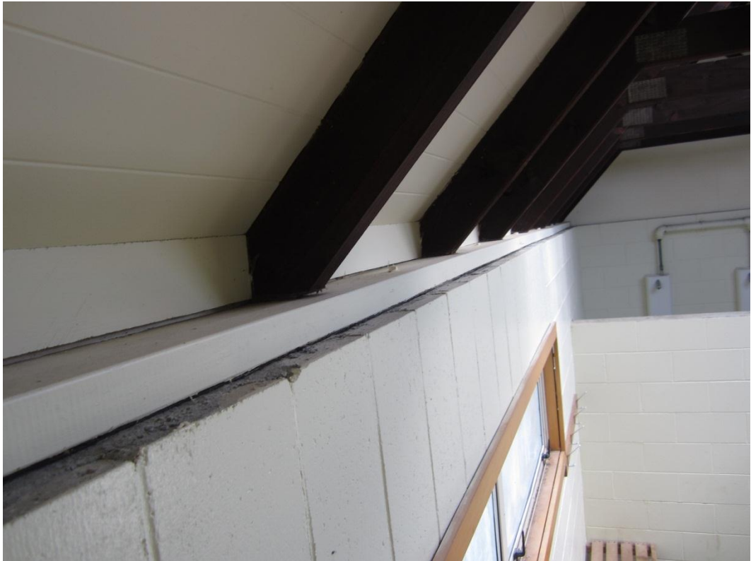
Photograph 7 Wall plate connection between timber trusses and concrete masonry walls
