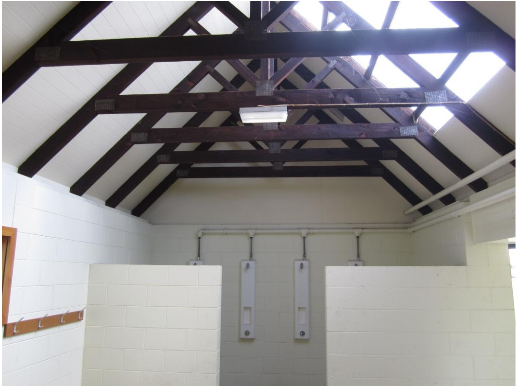
Photograph 5 Unrestrained concrete masonry shower partition walls
