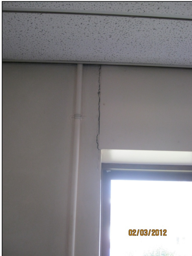
Photo 5: Cracks between panel joints
