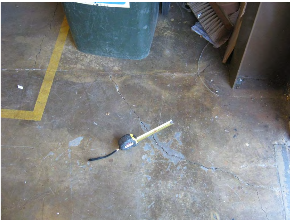
Photo 4: Cracks observed within floor slab, 1mm to 2mm wide.
