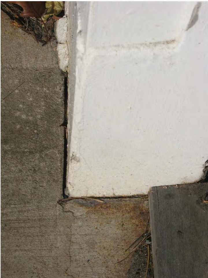
Photo 14: Minor gap opened up between eastern side of the building and the asphalt carpark.
