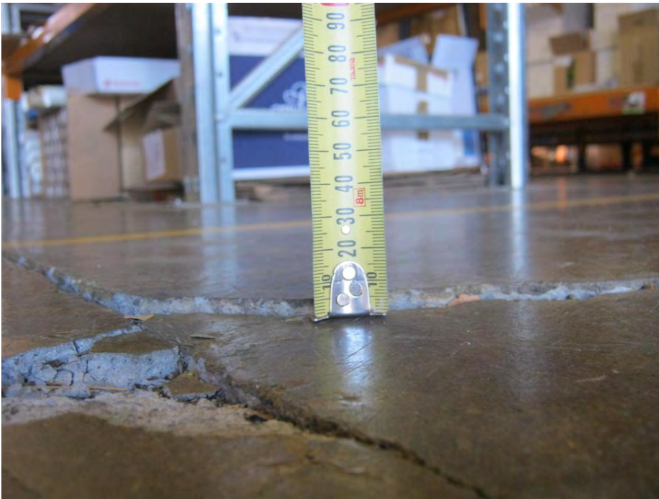
Photo 9: Differential Settlement of 5mm across a crack within the floor slab.
