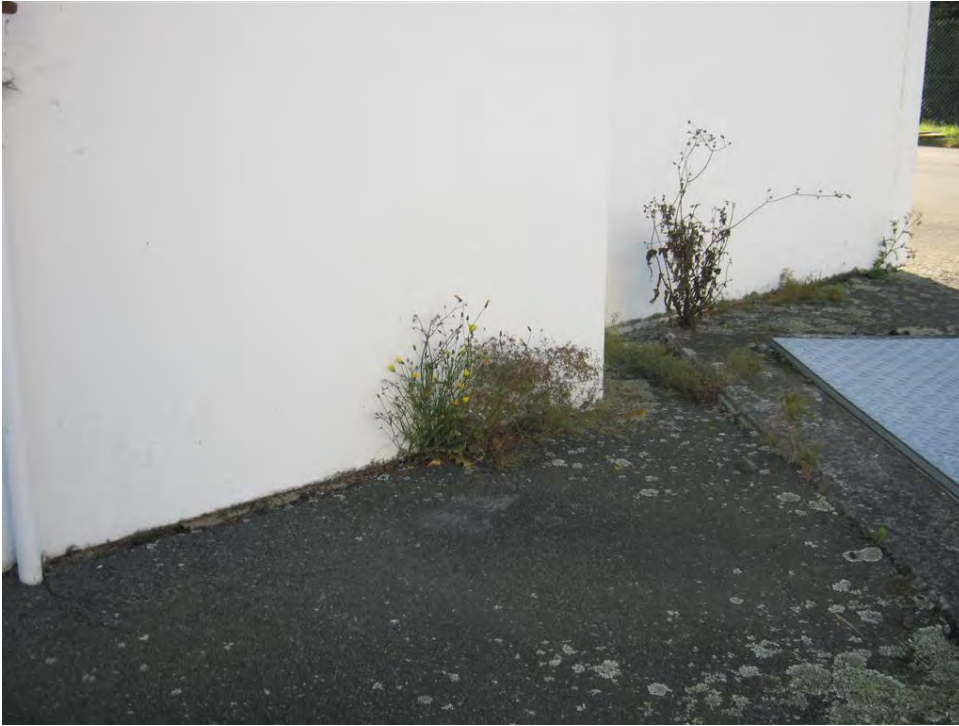
Photo 11: Land settlement around manhole and south-eastern corner of building, maximum settlement 30mm.
