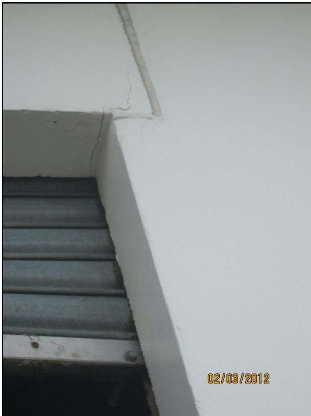
Photo 6: Crack at panel seating
