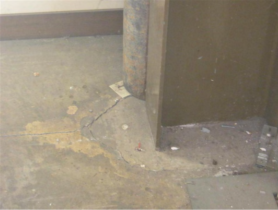
Photo 5: Cracks observed at the base of column, 1mm to 2mm wide.
