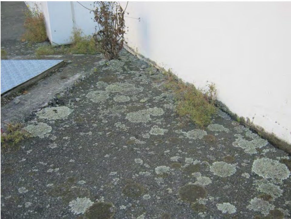
Photo 12: Land settlement around manhole and south-eastern corner of building, maximum settlement 30mm.
