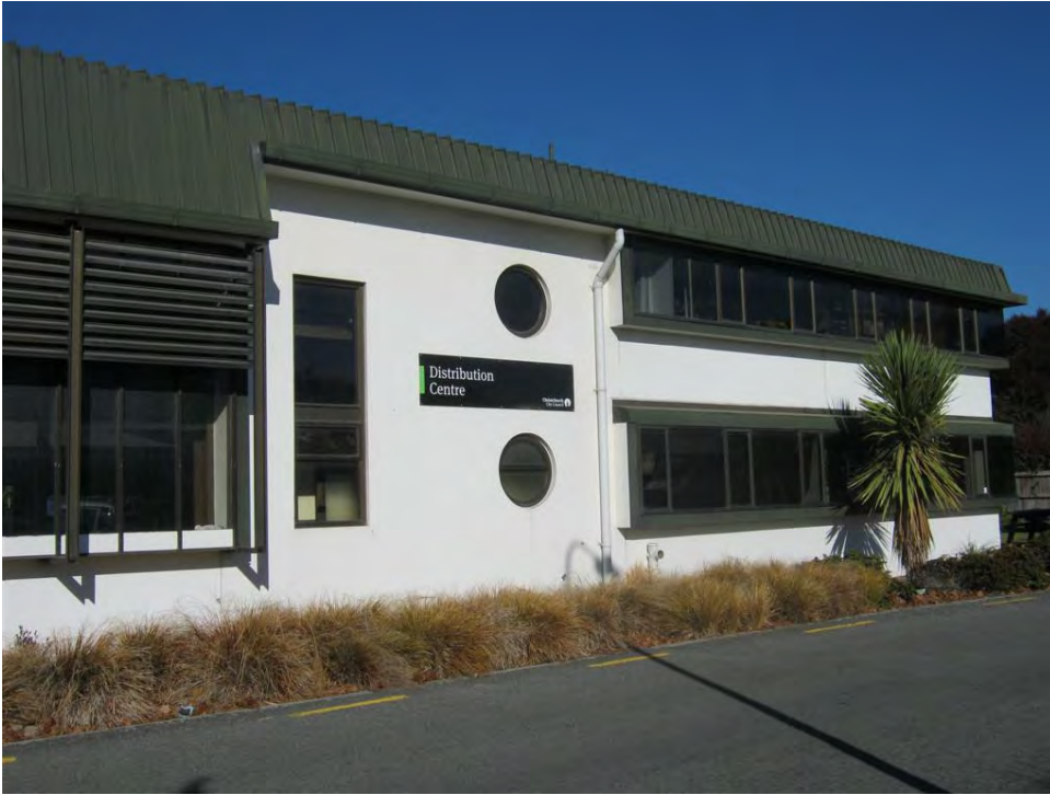
Photo 1: Northern elevation, Waterworks MPS - Workshop, 54 Colombo Street.
