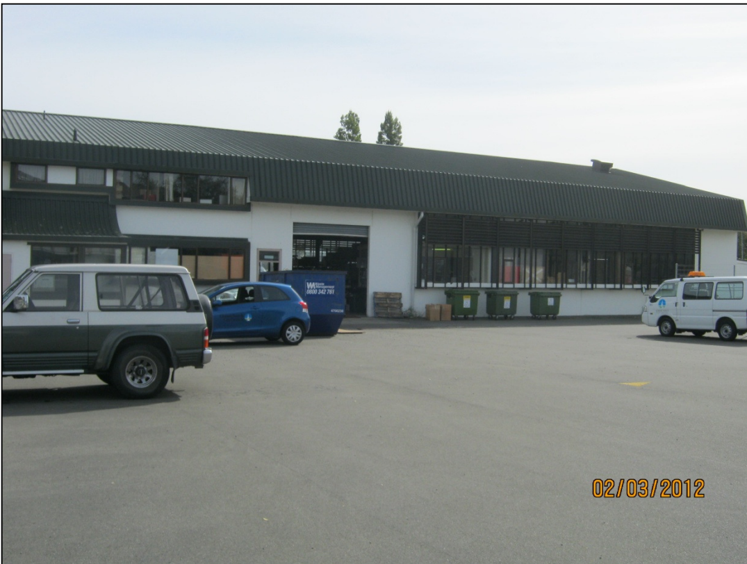
Photo 2: South facing wall
