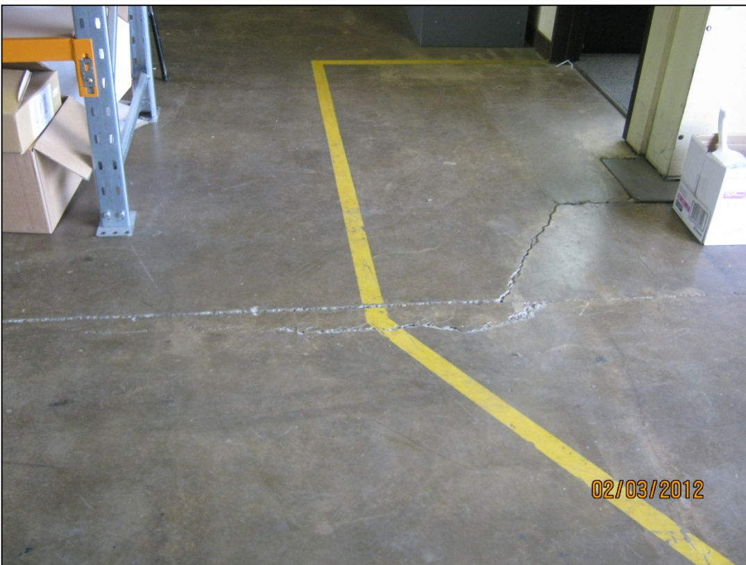
Photo 4: Cracking of floor slab
