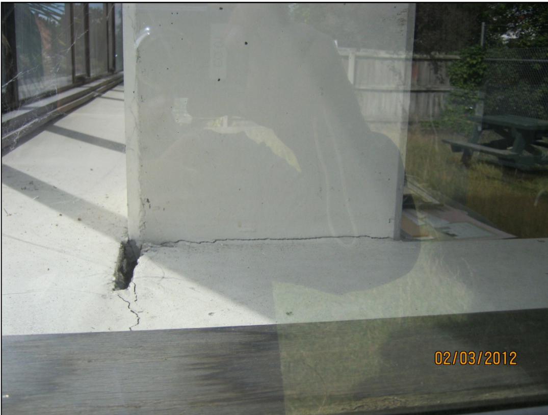
Photo 3: Misalignment of wall panel at western end
