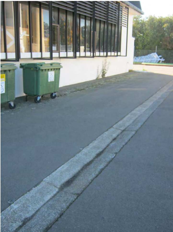
Photo 10: Raised drainage channel by approximately 1mm to 2mm.
