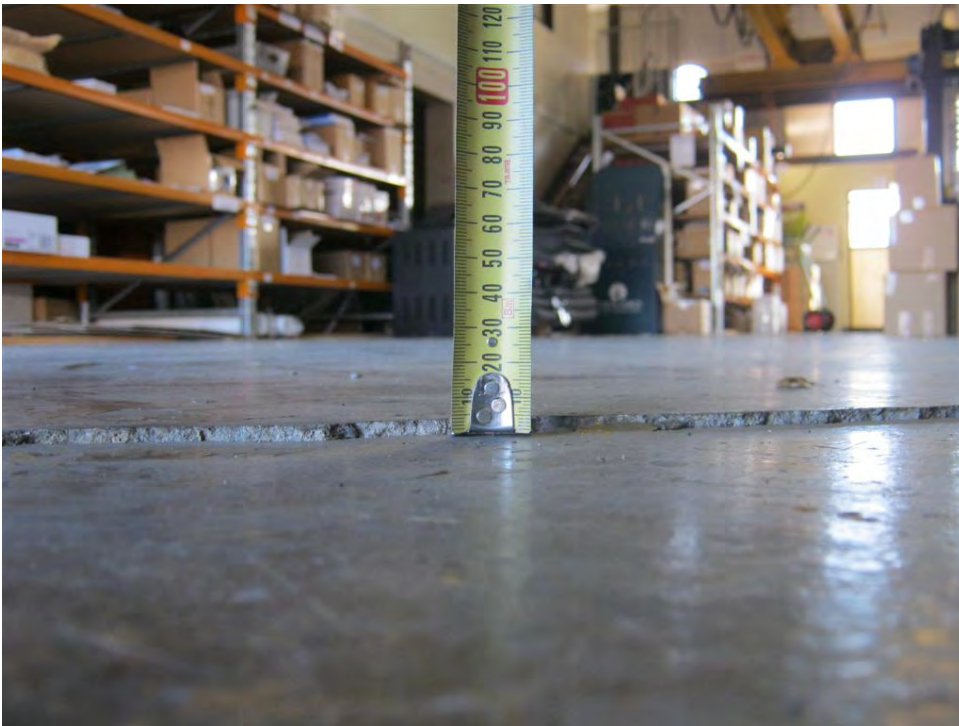
Photo 8: Differential Settlement of 5mm across a crack within the floor slab.
