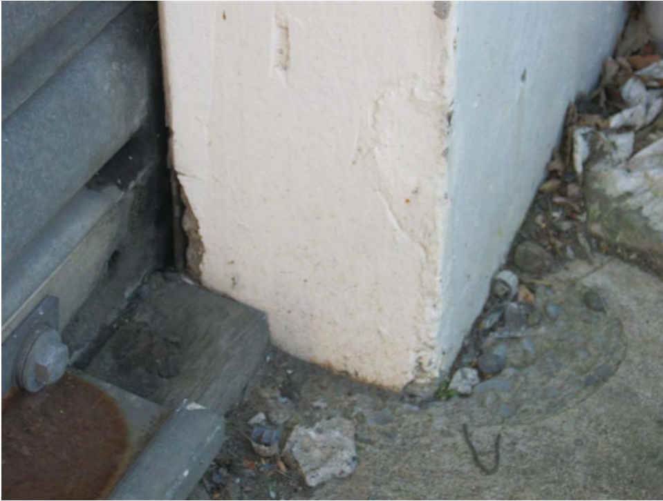
Photo 13: Minor spalling of concrete at the eastern roller door.
