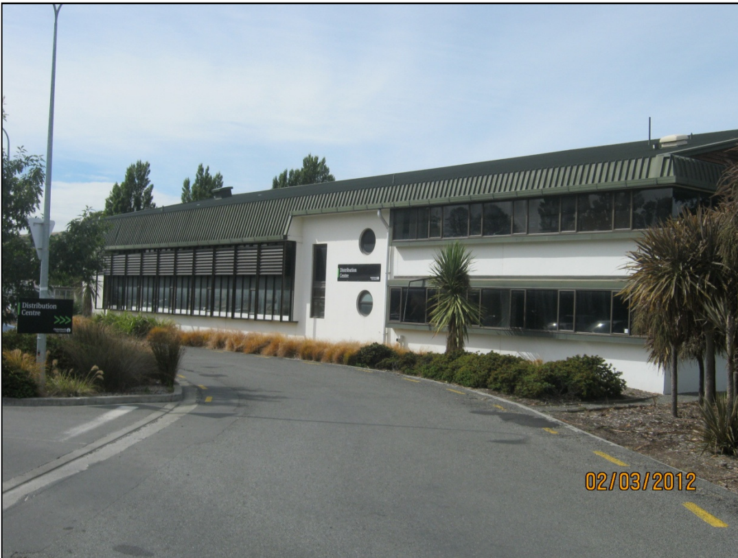
Photo 1: North facing wall
