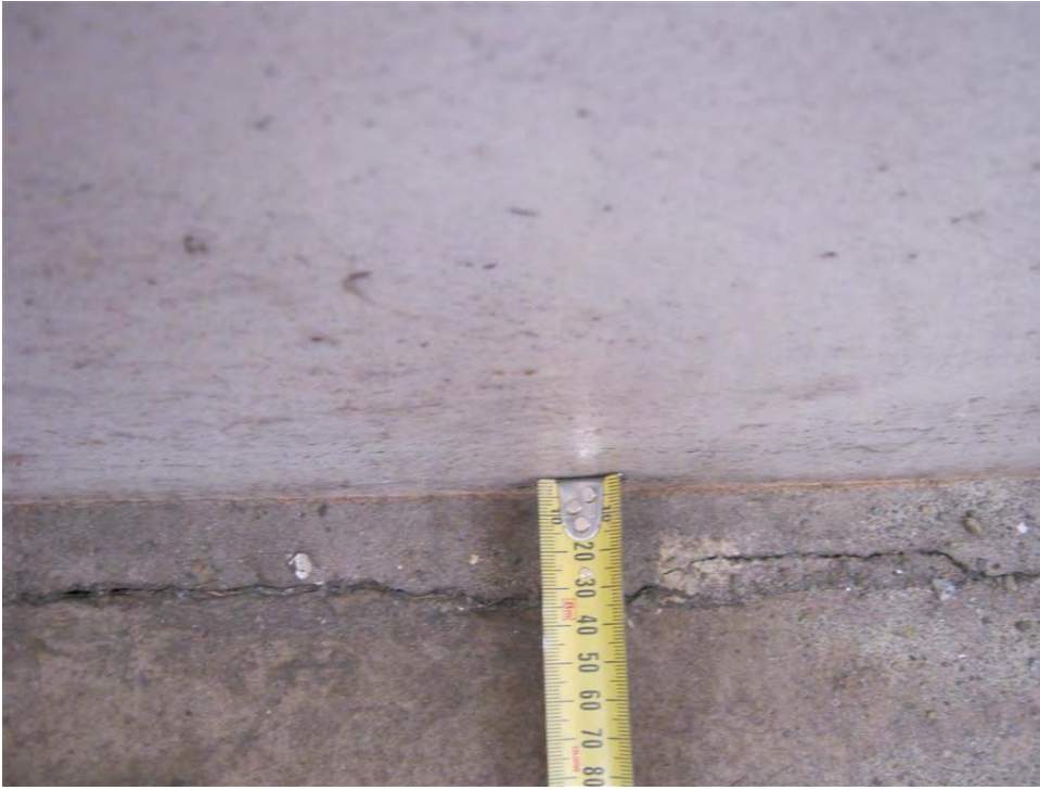
Photo 7: Crack at the base of the wall, 1mm to 2mm wide.
