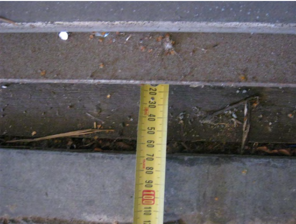
Photo 6: Gap opened up between the base of the roller door on the eastern side of the building and the floor slab.
