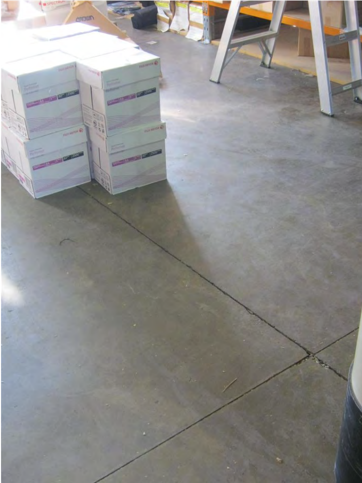
Photo 3: Gaps opened up between floor slabs, maximum 10mm wide.
