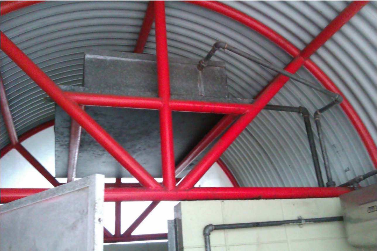
Photo 3: Internal View of Roof
