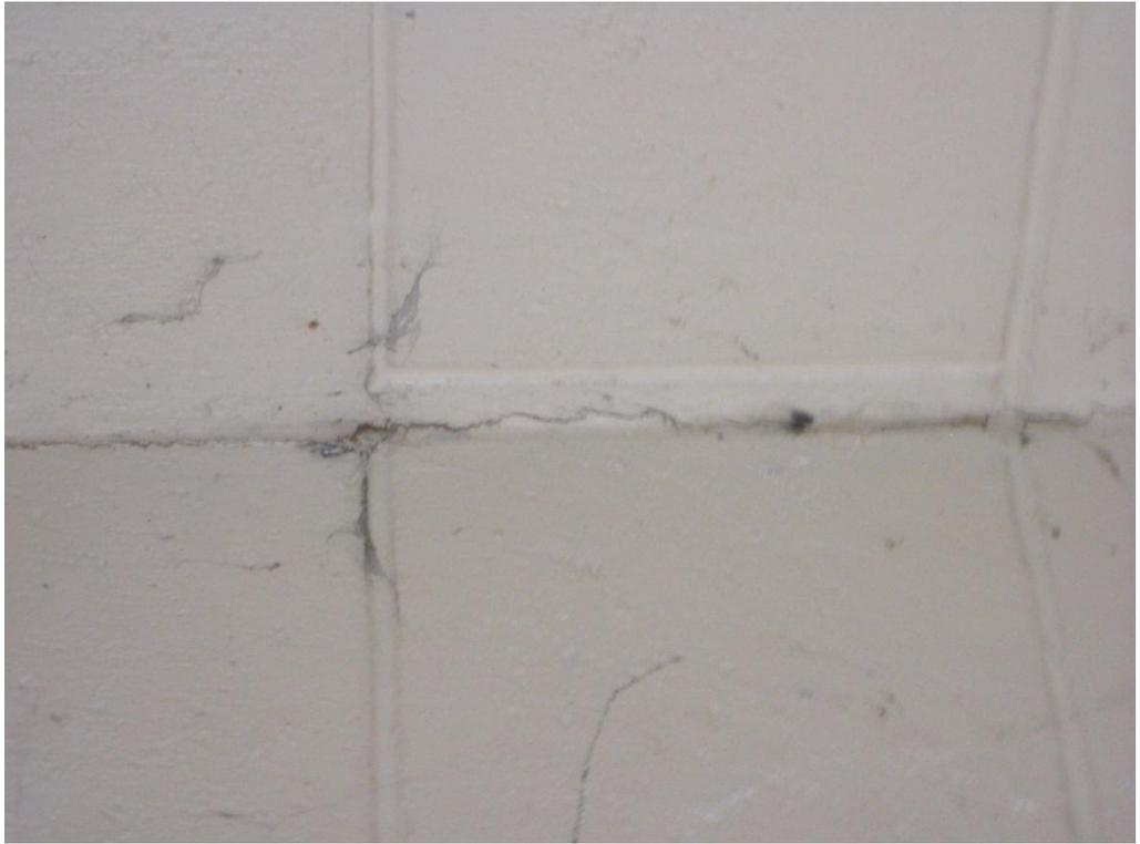
**Photograph 7: Seismic damage to front external wall.**
