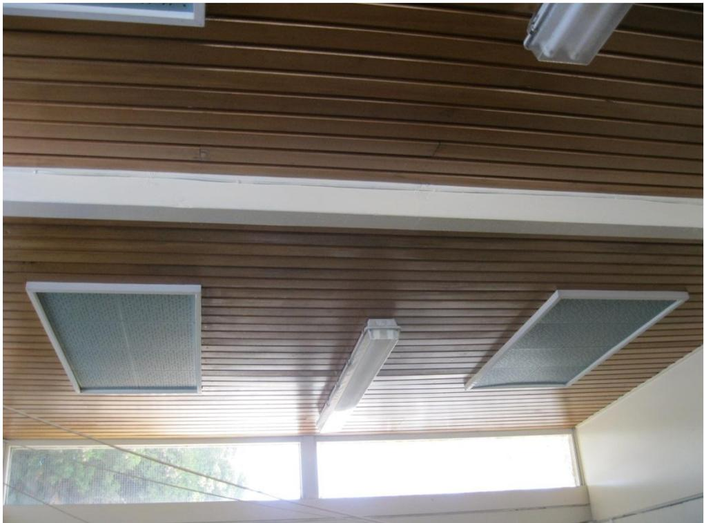
**Photograph 4: Timber ceiling battens.**
