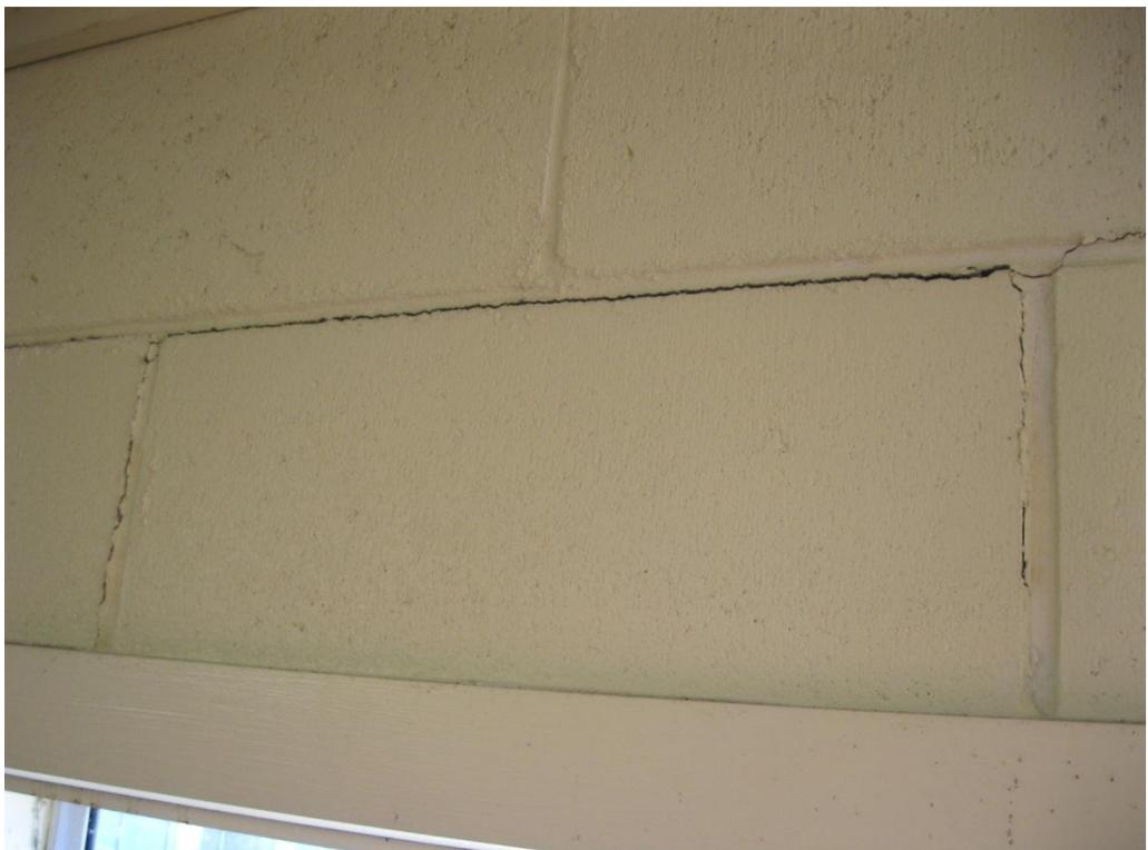
**Photograph 6: Seismic damage to front external wall.**
