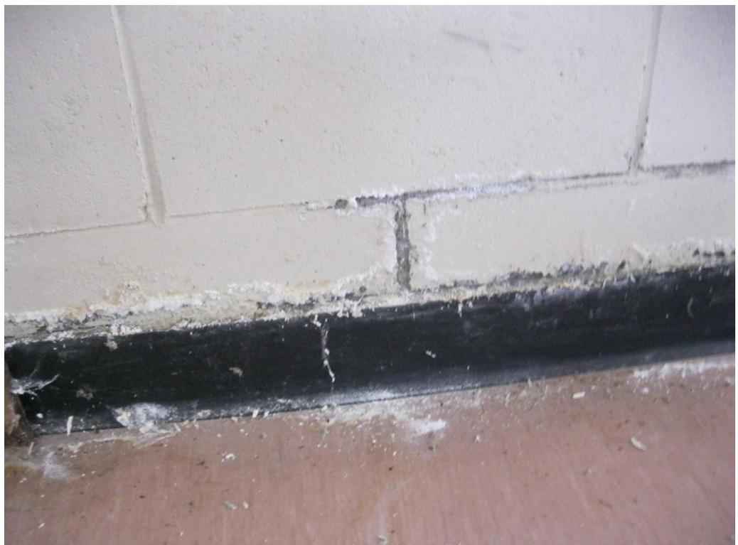
**Photograph 8: Chloride deterioration at base of front external wall.**
