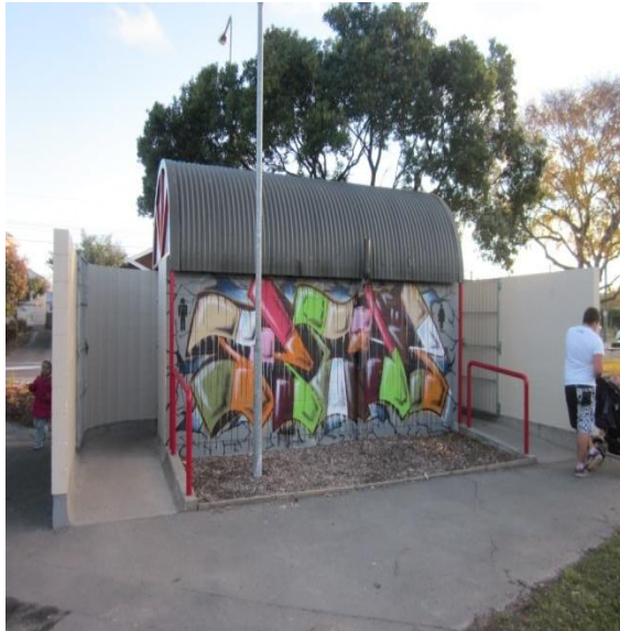
Photo 1: The east elevation of Building 6
