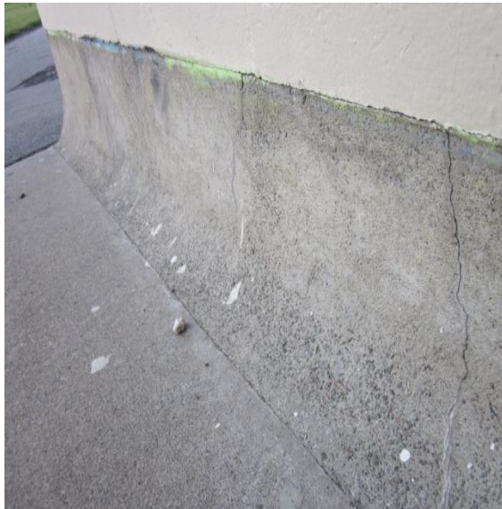
Photo 3: Non-earthquake related cracking in the concrete fillet at the base of the masonry walls
