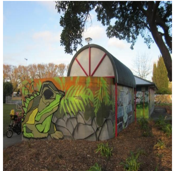
Photo 2: The north and west elevations of Building 6
