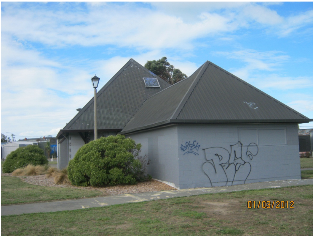
Photo 4: Right Flank (West Elevation)
