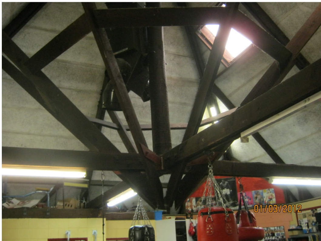
Photo 16: Trussed Roof of Original Building
