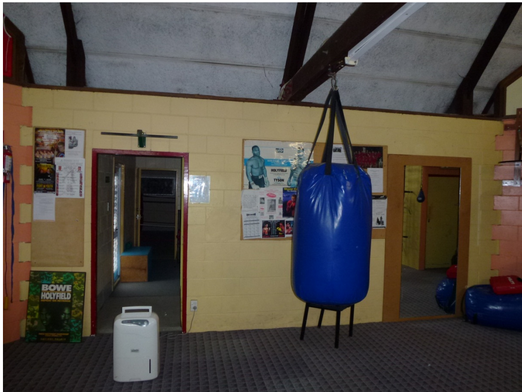
Photo 10: West Wall of Original Building (Internal View)
