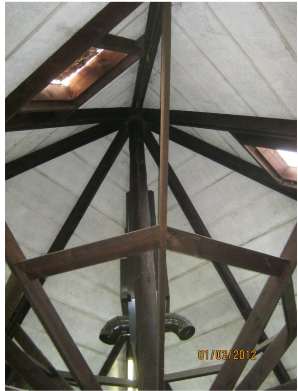
Photo 17&18: Trussed Roof of Original Building
