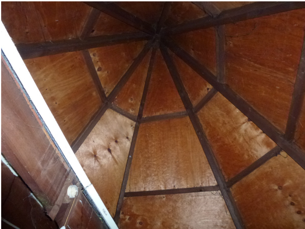
Photo 21: Kitchen Addition (East) Main Roof
