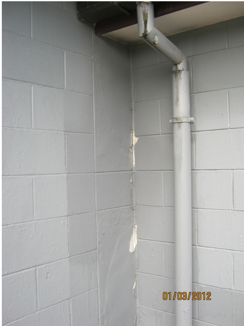
Photograph 3. Hairline crack in brick wall (does not extend into foundation)
