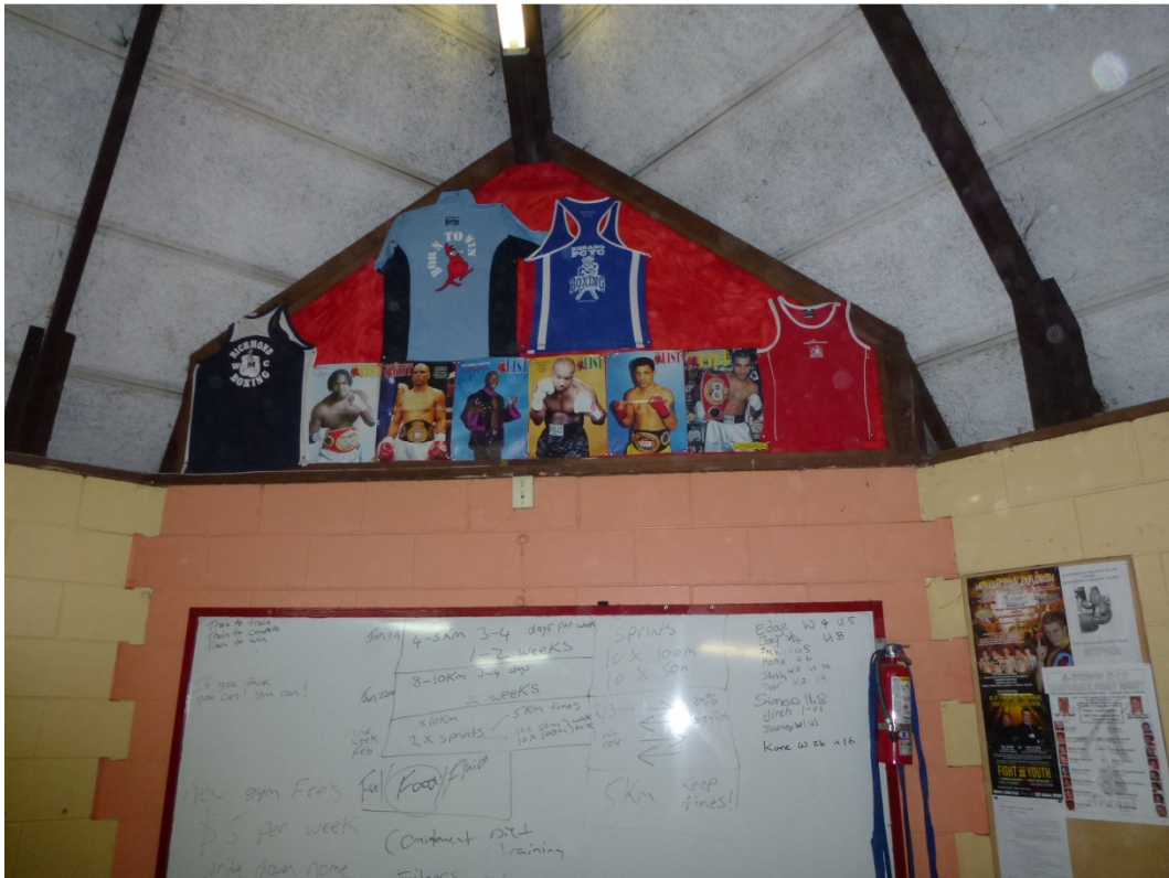
Photo 15: South-West Corner of Original Building (Internal View)
