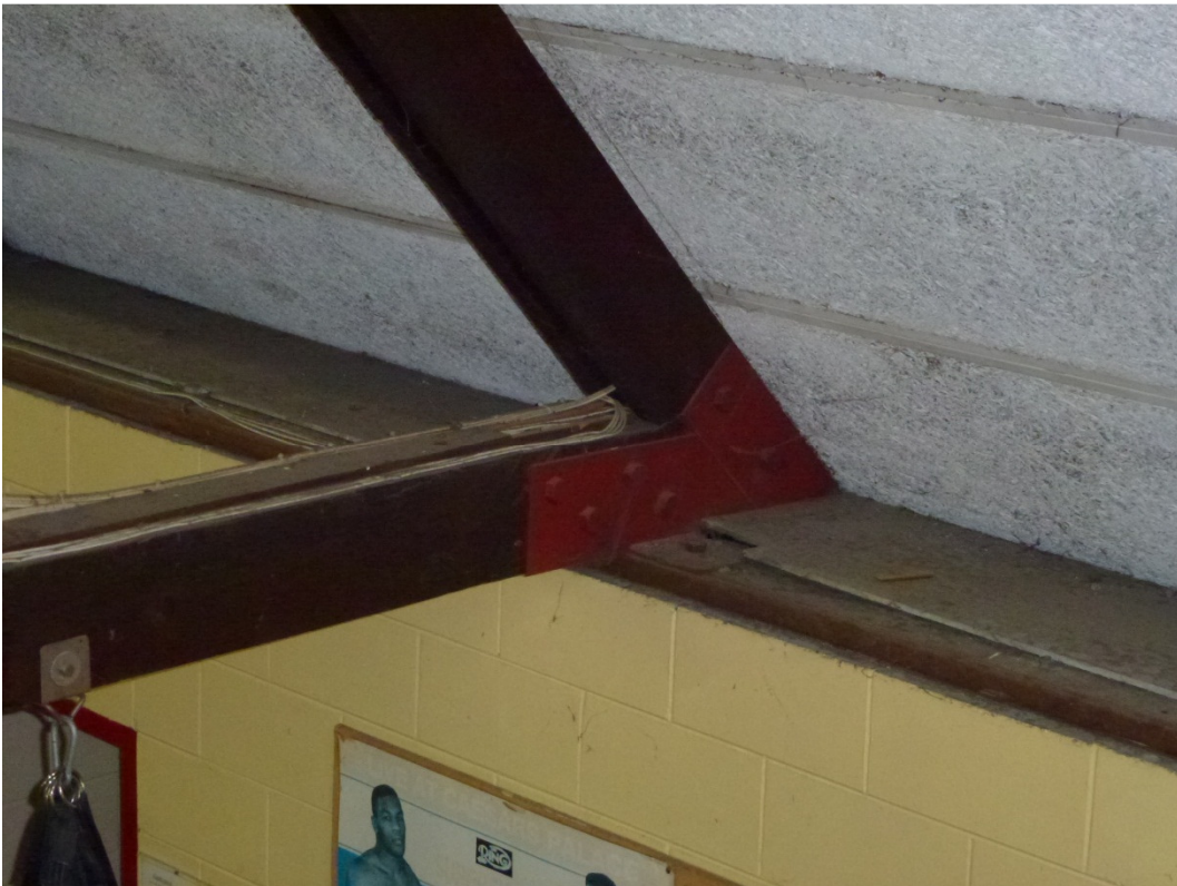
Photo 20: Typical Main Roof Truss Connection
