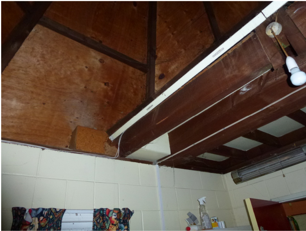
Photo 22: Junction between Kitchen Addition & Main Building
