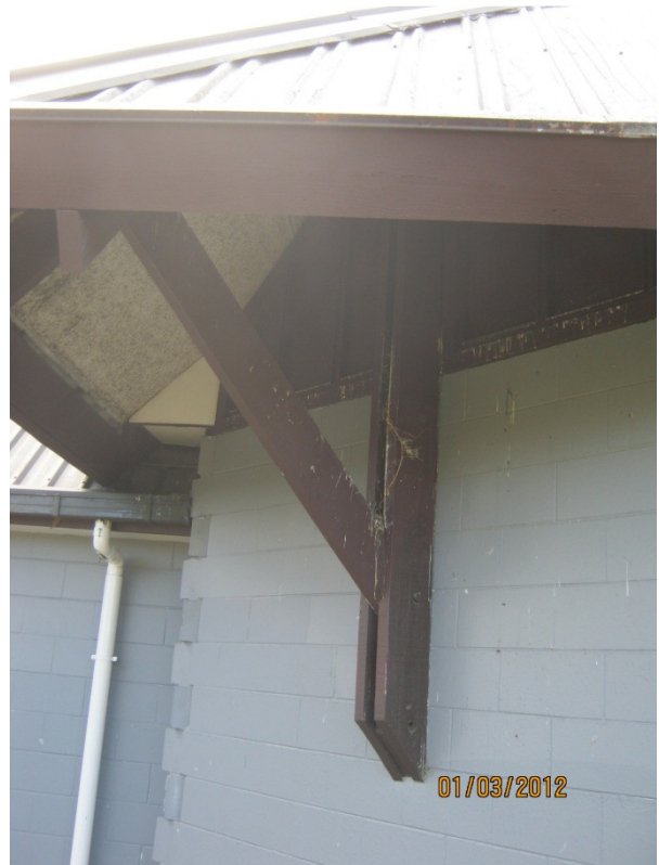
Photo 6: Overhang & Bracket to Main Roof
