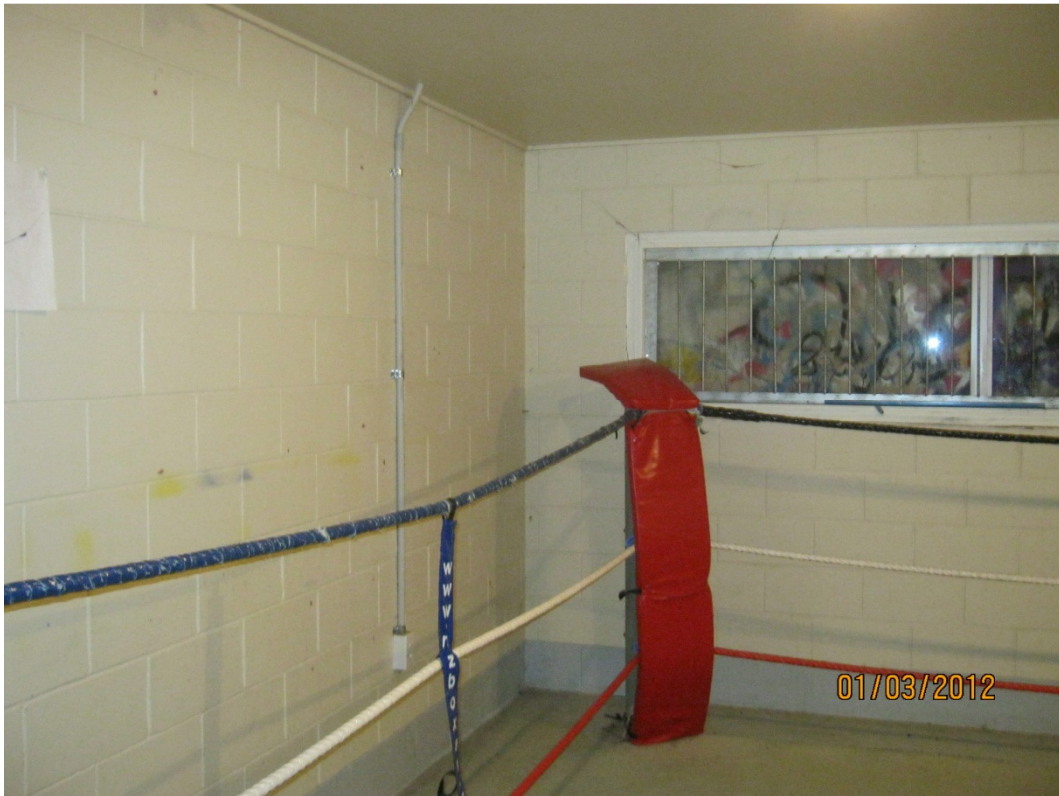
Photo 9: South-West Corner of Main Addition (Internal View)
