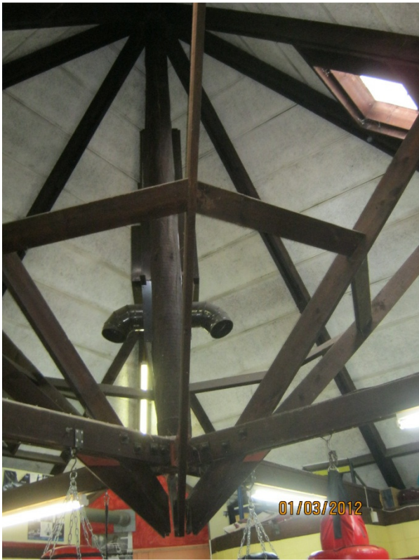
Photo 17&18: Trussed Roof of Original Building
