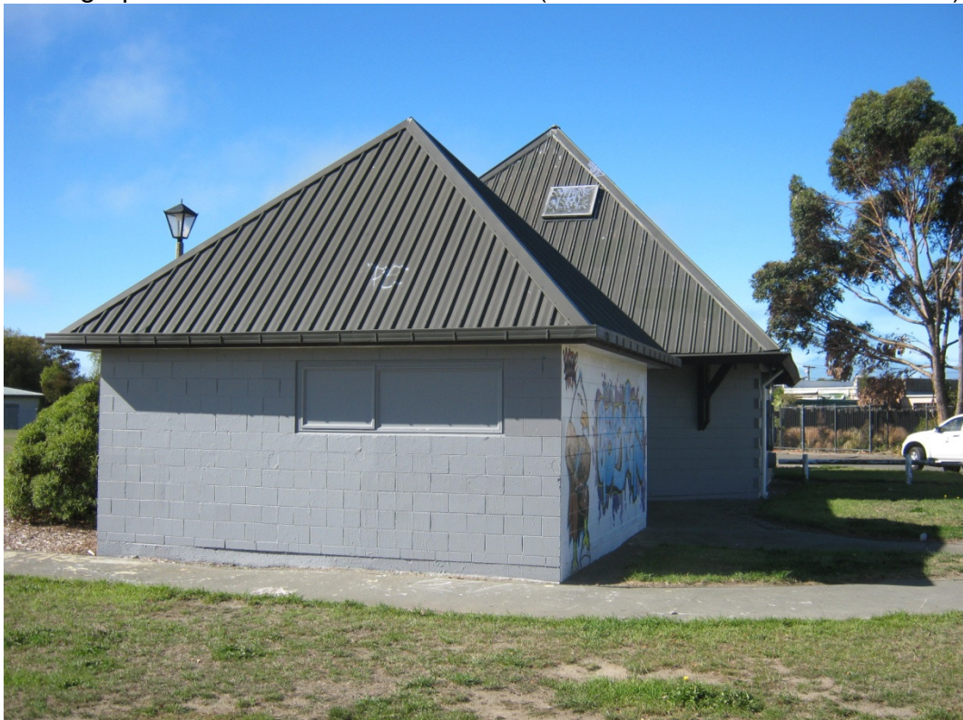
Photograph 4. Western elevation of the building
