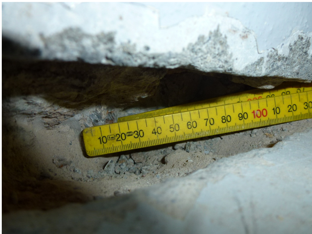
Photo 23: Confirmation of Main Vertical Reinforcement
