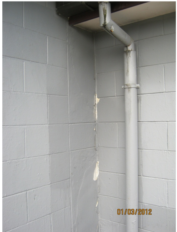
Photos 7&8: Cracking Between Original Building & Main Addition
