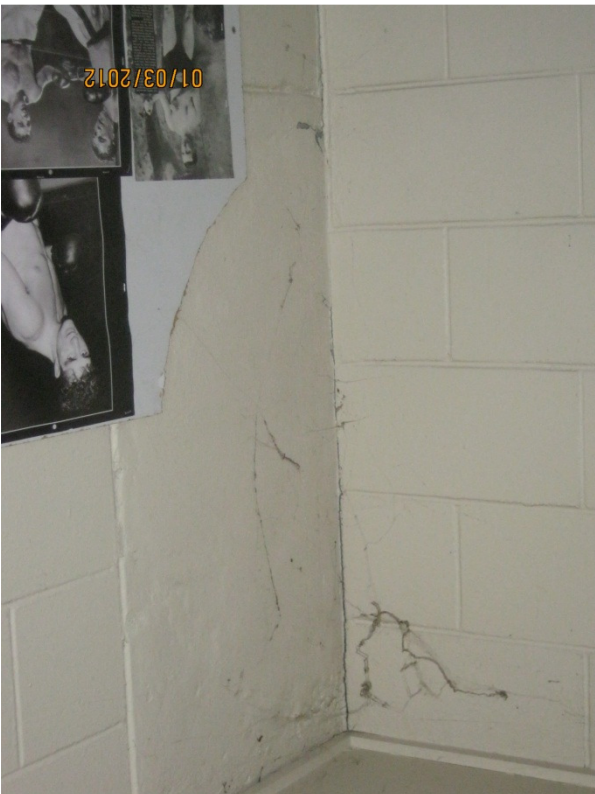
Photos 7&8: Cracking Between Original Building & Main Addition
