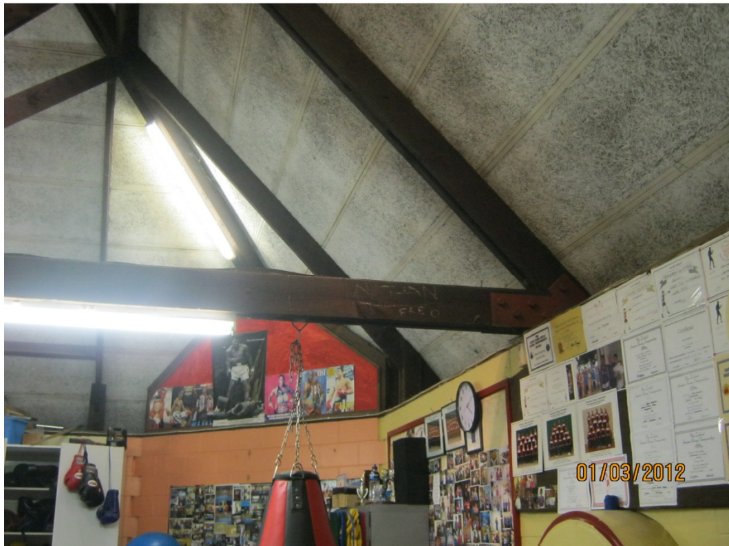
Photo 19: Typical Roof Bearing (Internal View)
