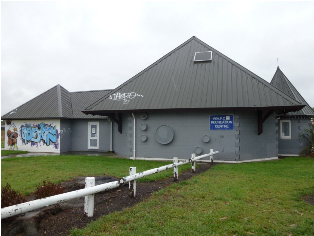
Photo 3: Rear (South Elevation)
