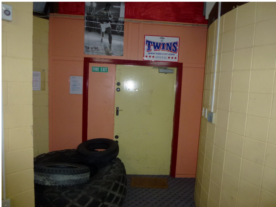
Photo 14: Entrance at North-East Corner of Original Building (Internal View)
