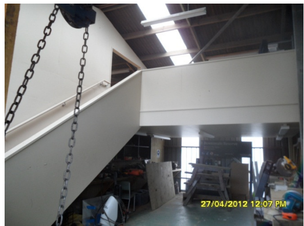
View of the mezzanine on the south end of the building from the ground floor.
