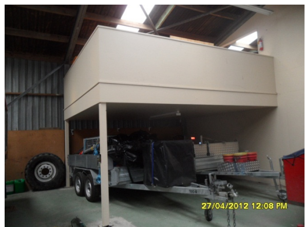
View of the mezzanine on the north end of the building from the ground floor.
