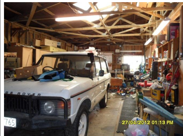
Internal view of the south end of the building.
