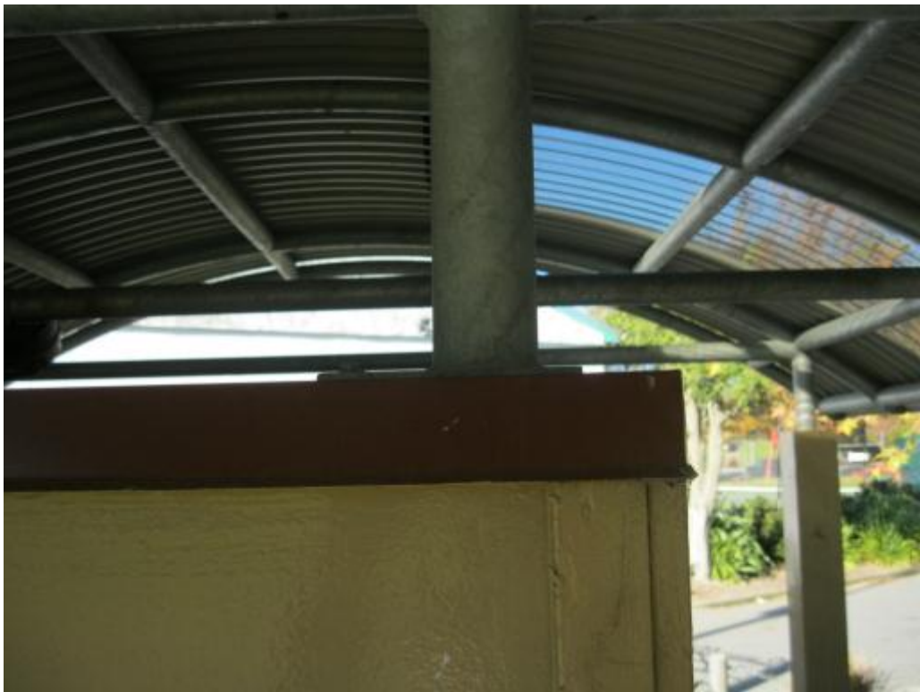
Photo 4. Steel tube post supported on load bearing timber frame wall.
