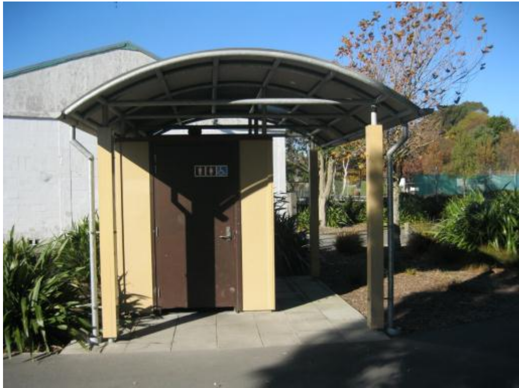
Photo 1. View of toilets from the northwest.
