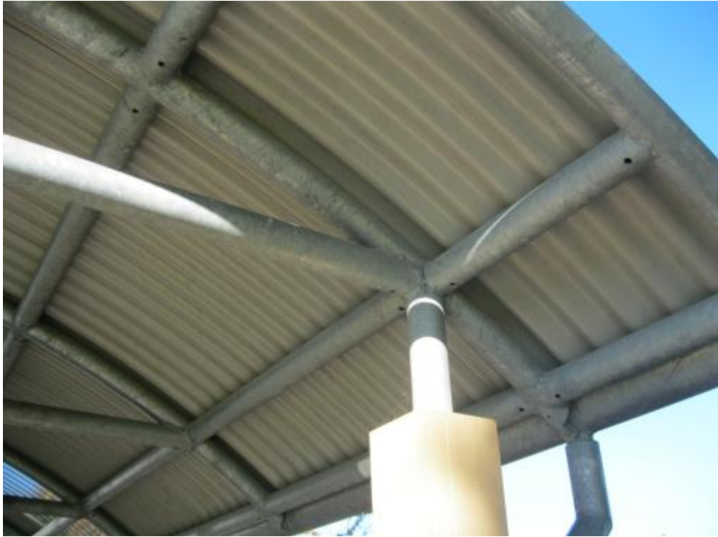
Photo 3. Rigid frame formed from fixed connections of steel tubes.
