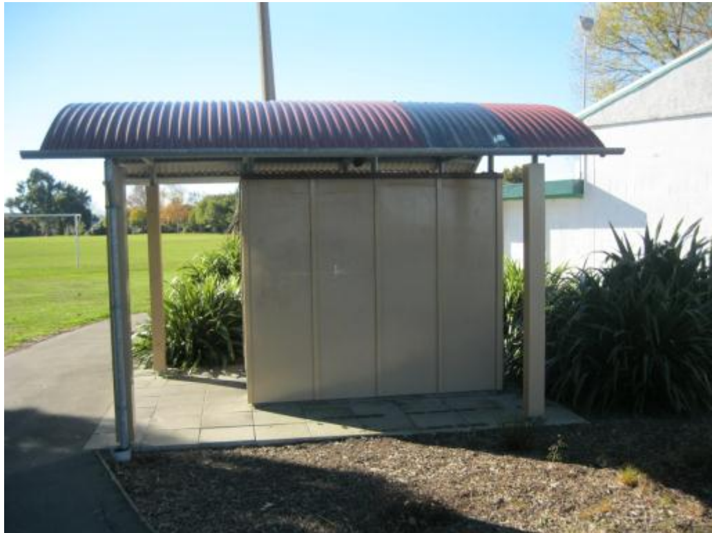
Photo 2. View of toilets from the southwest.
