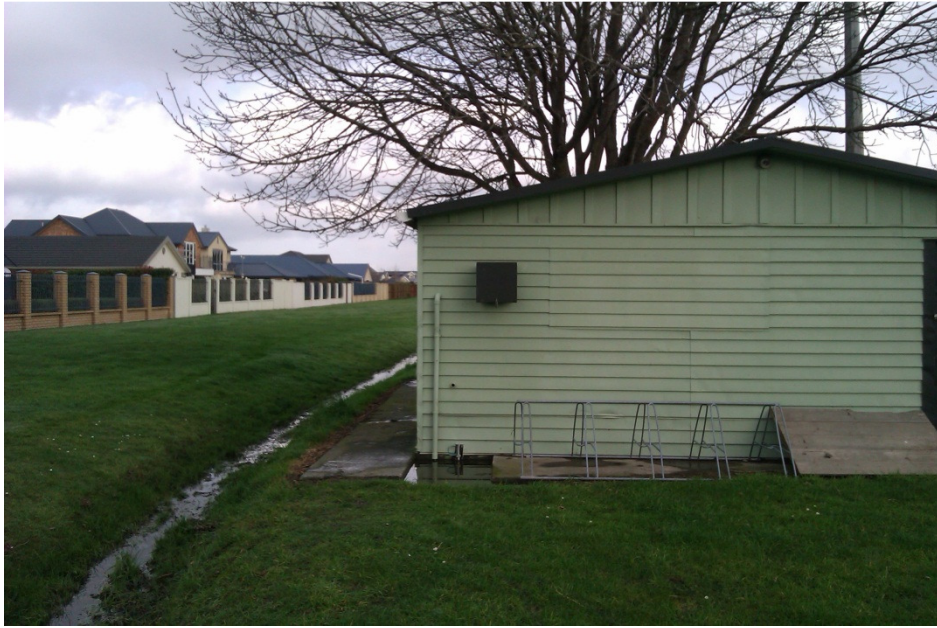
Photo 3: View of the front and drainage ditch
