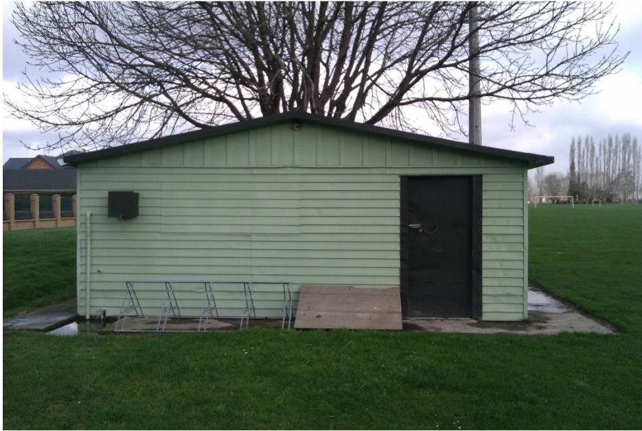
Photo 1: View of the front of the building
