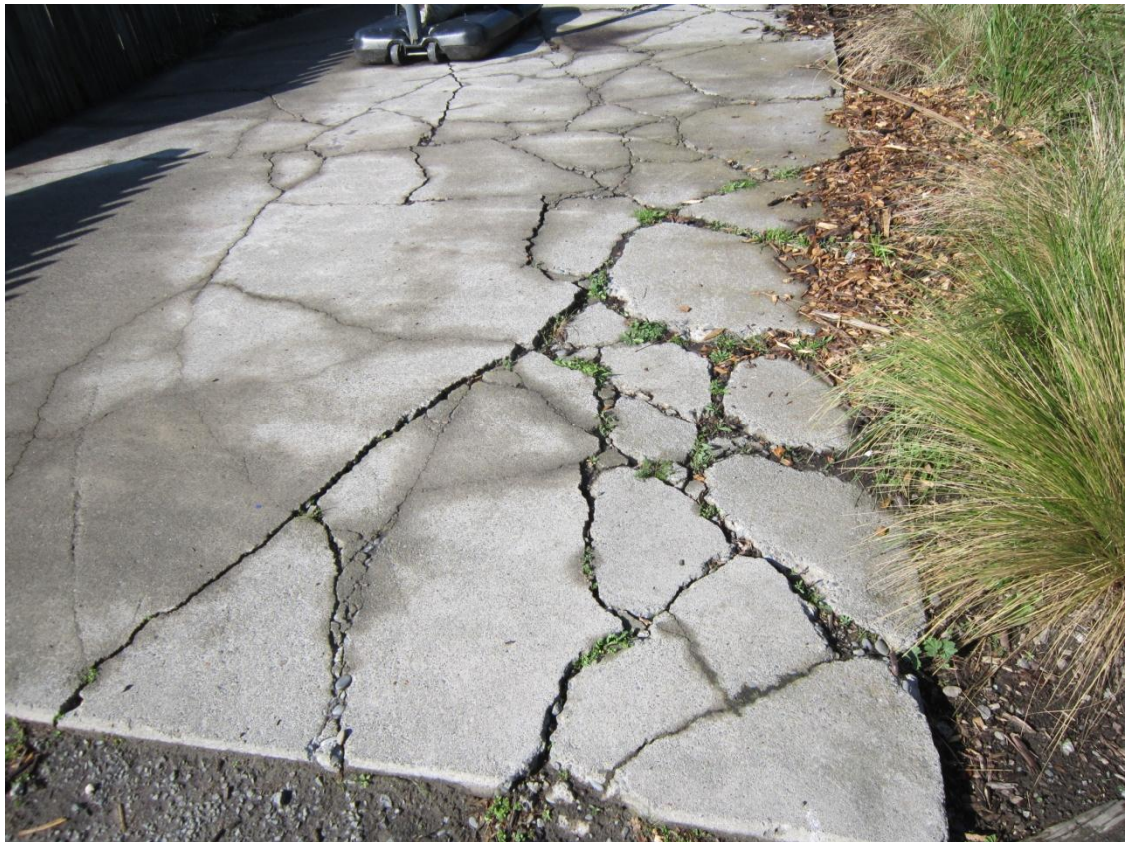
■ Figure 16 - Significant cracking of the slab west of the building
