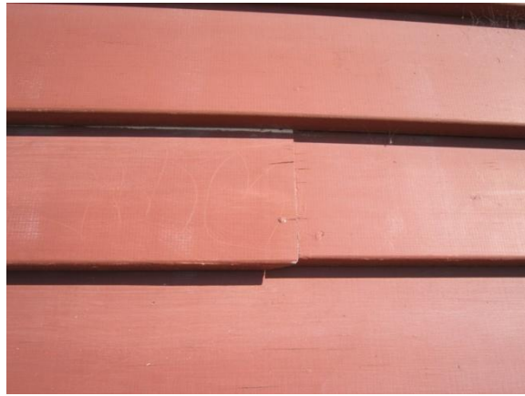
Photo 5: Dislodged weathboard on east wall
