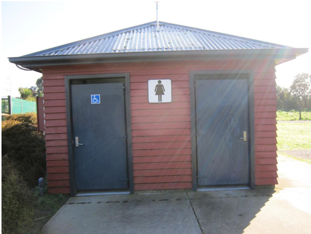
■ Figure 8 - Small separation of the pavement slabs
