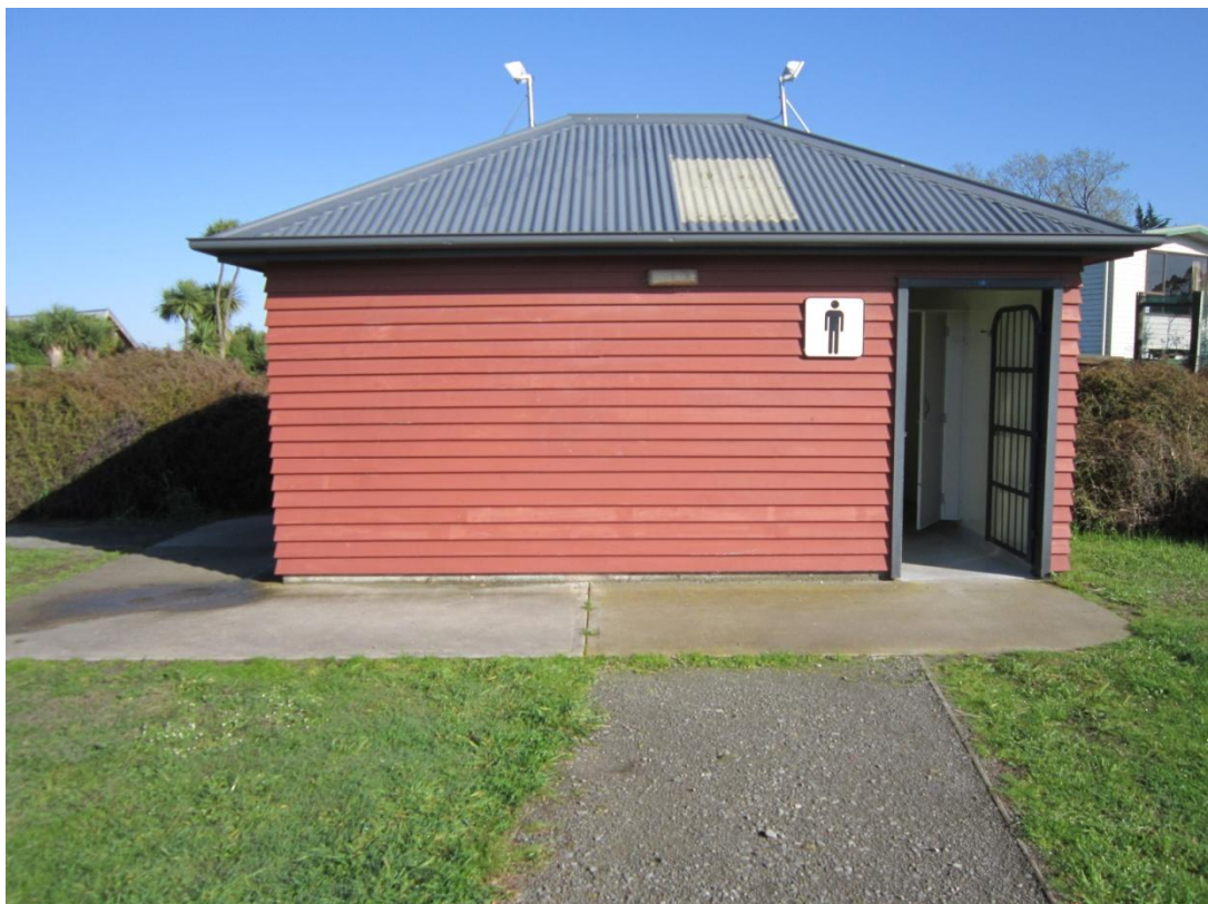
■ Figure 7 - Overview of the toilet block
