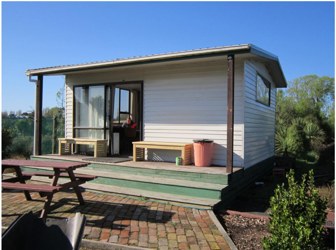
■ Figure 13 - Overview of building
