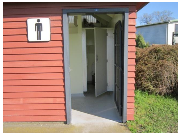
Photo 8: Internal view of male toilet
