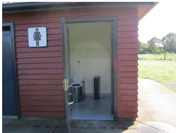
Photo 7: Internal view of female toilet
