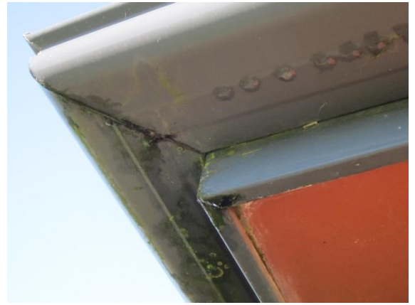
Photo 6: Water damage to underside of gutter (typical)
