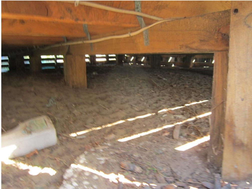
■ Figure 14 - Observed foundation for the building
