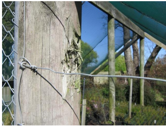
Photo 9: Impact damage on timber pole on east side of south plant nursery
