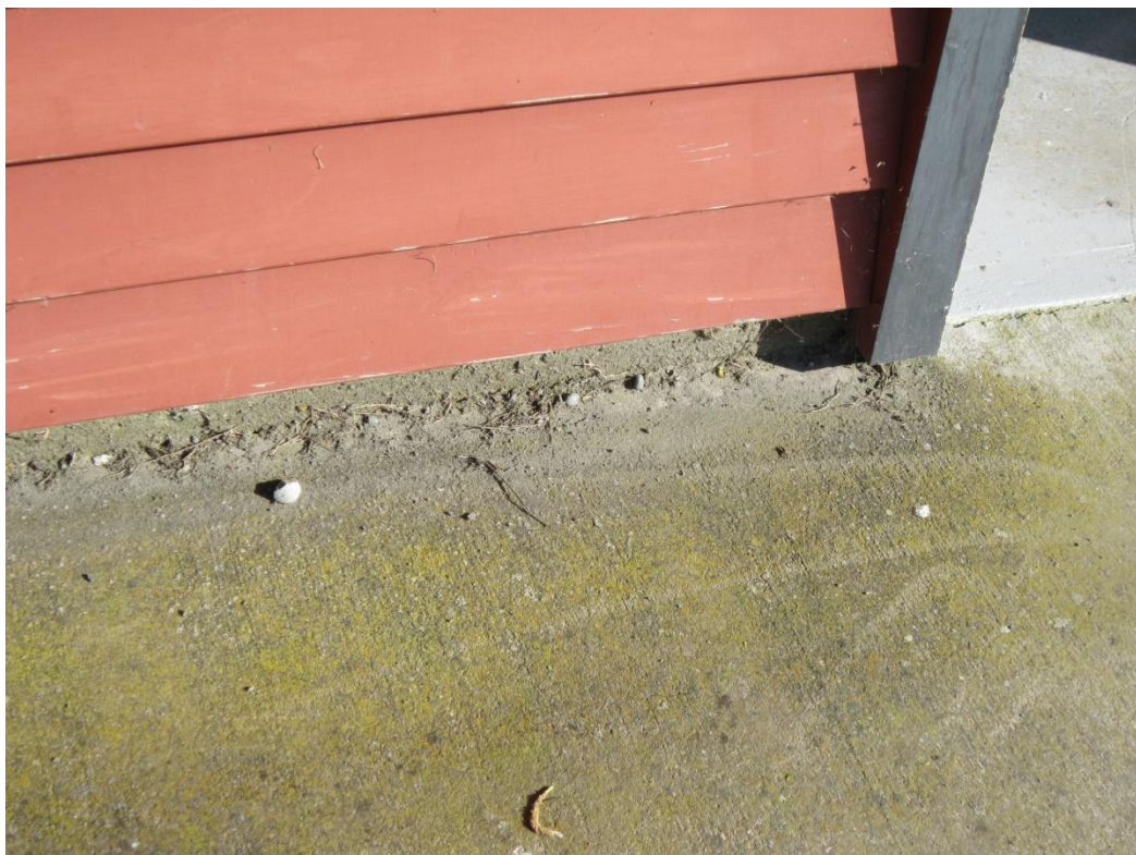
■ Figure 9 - Remaining silt ejecta from the earthquake event
