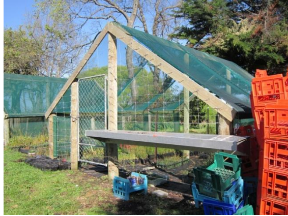
Photo 1: East elevation of north plant nursery
