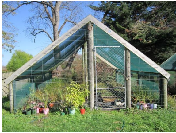
Photo 5: East elevation of south plant nursery
