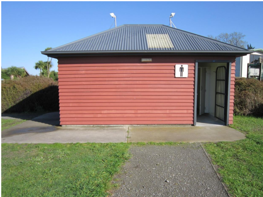
■ Figure 7 - Overview of the toilet block
