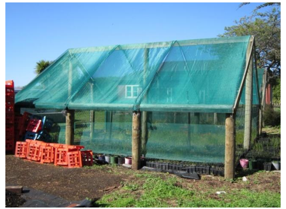
Photo 4: North elevation of north plant nursery
