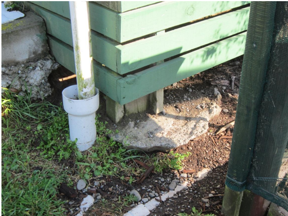
■ Figure 15 - Concrete encased piles some separation between the block and adjacent ground
