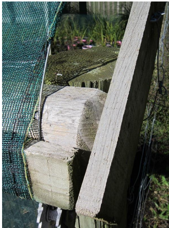
Photo 11: Connection between end timber frame rafter, timber pole and longitudinal beam
