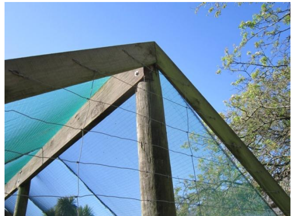
Photo 10: Connection of timber elements at apex on end timber frame
