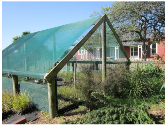
Photo 7: West elevation of south plant nursery
