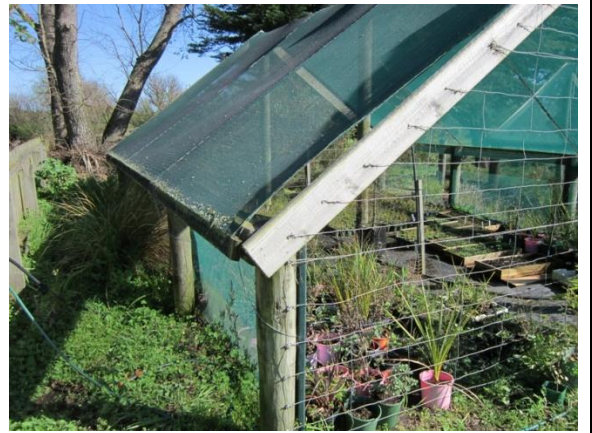
Photo 6: South elevation of south plant nursery
