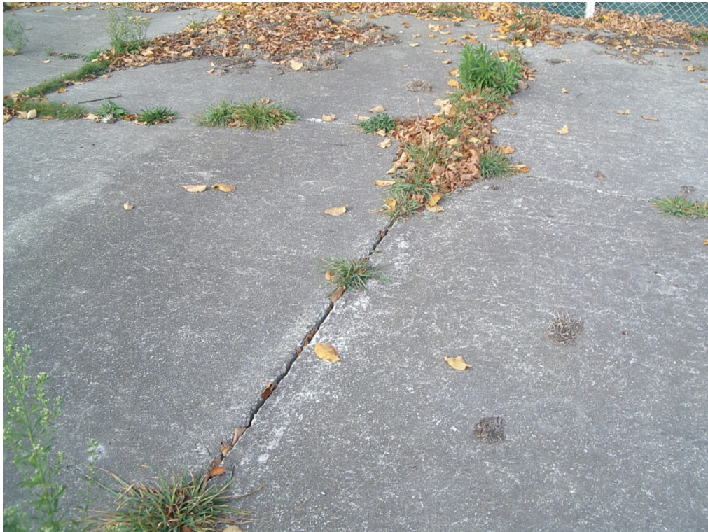
■ Figure 16 - Noted damage to the concrete paving
