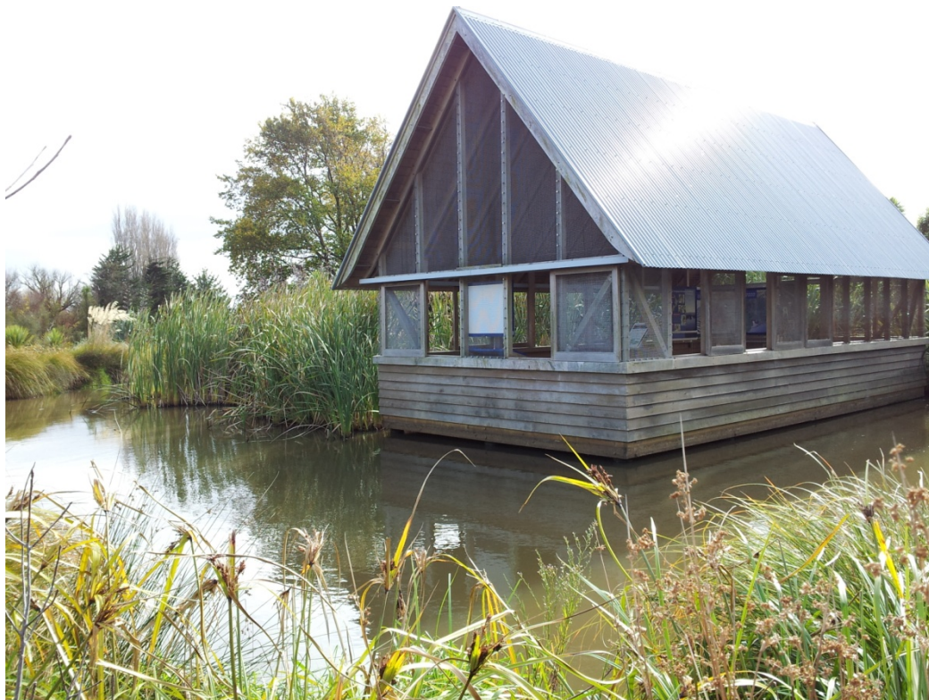
■ Figure 11 - Overview of the information kiosk (western elevation)
