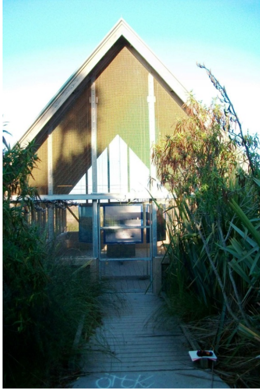
Photo 1: Information Kiosk - Eastern Elevation
