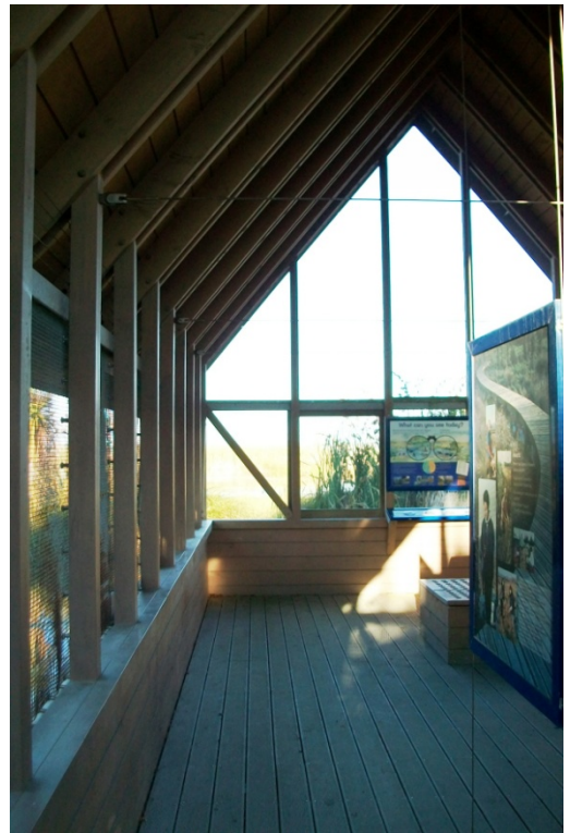
Photo 6: Internal View Looking West
