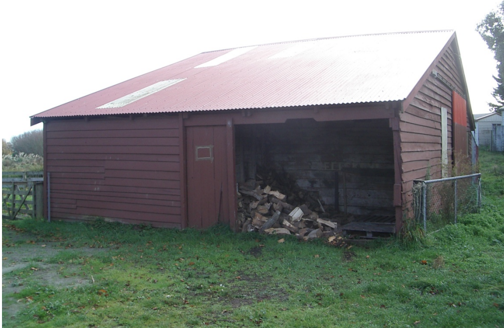
■ Figure 14 - Overview of the barn structure
