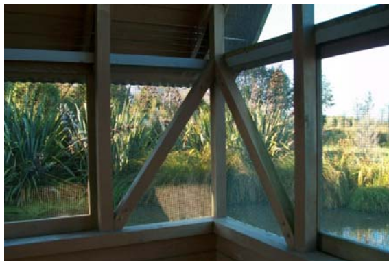
Photo 7: Corner Bracing -Typical
