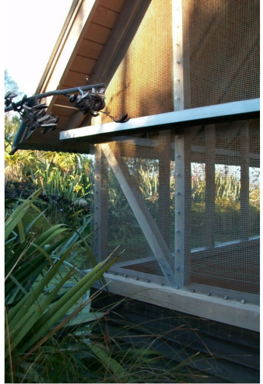
Photo 2: SE Corner Details
