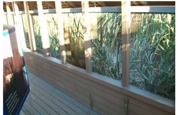
Photo 4: Typical Wall Details
