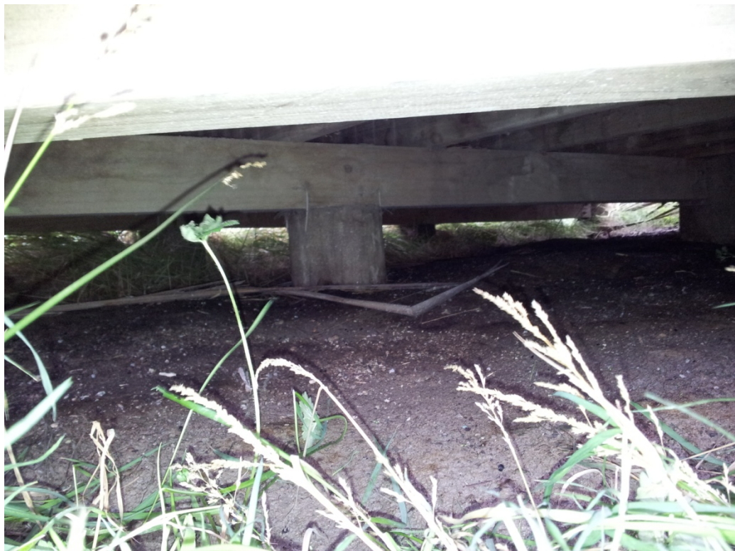
■ Figure 13 – Foundation details of the bird hide
