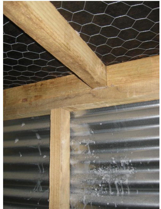
Photo 4: Typical Roof Structure Details
