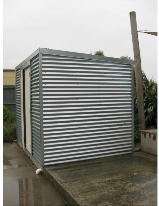
Photo 2: Side Elevation of Building
