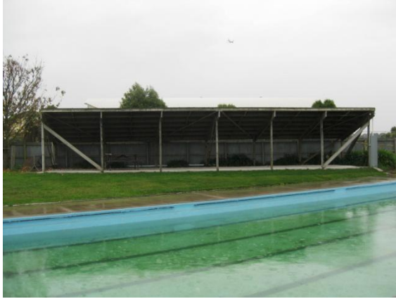
Photo 1: Front Elevation of Structure
