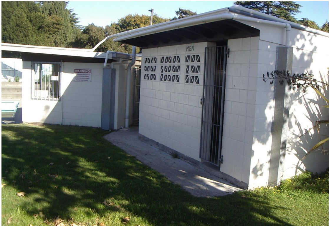
■ Figure 5 Overview of Toilet block and changing rooms
