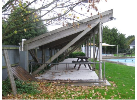
Photo 2: Side Elevation of Structure
