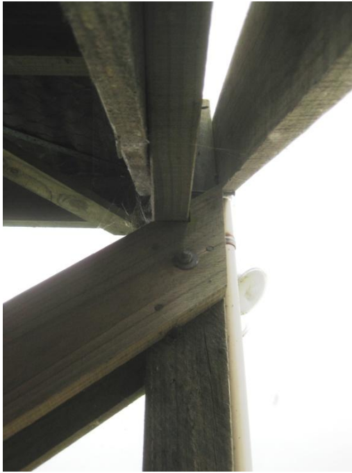
Photo 5: Close up of Bracing Connection
