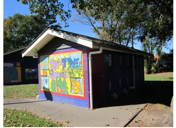
Photo 2: View of the building looking east
