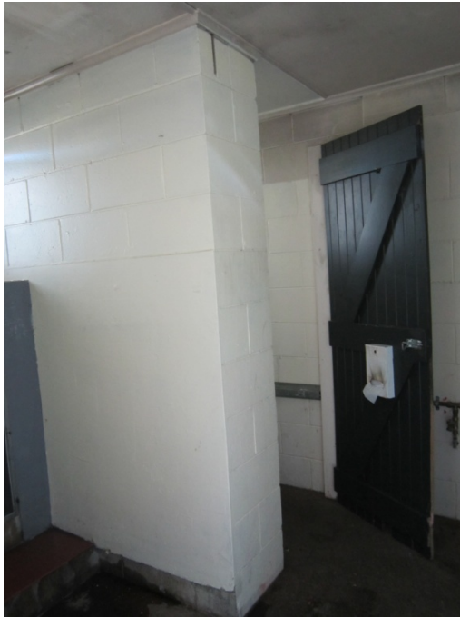
Photo 5: View of the block walls within the mens toilet area.
