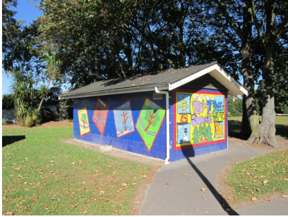
Photo 1: View of the building looking south
