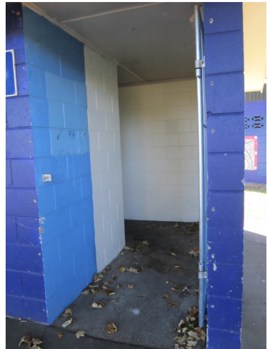
Photo 4: View of the mens toilet entrance block walls at either side of the opening
