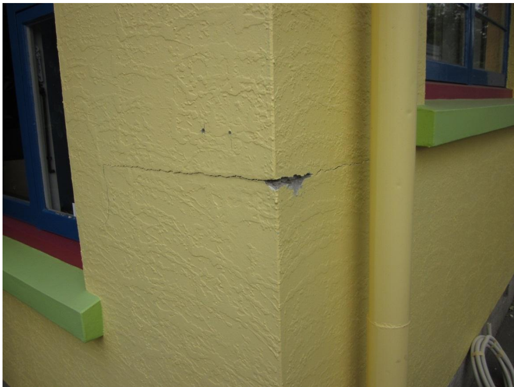
Photograph 4 Horizontal cracking traversing around the southernmost corner of the building, above and below window level.
