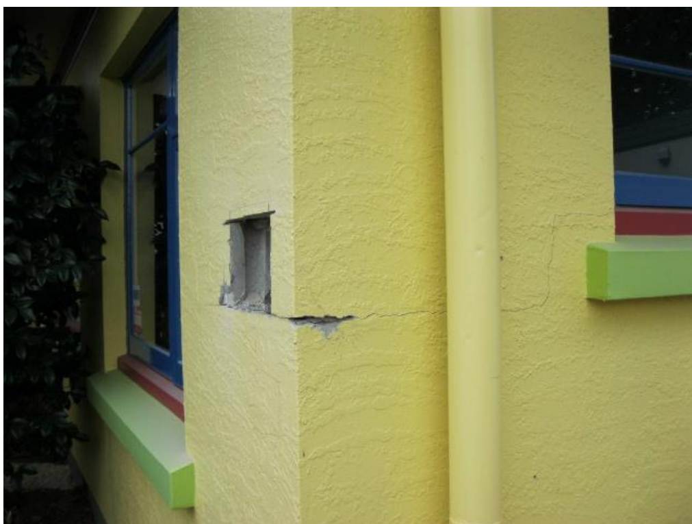
Photograph 13 Section of wall removed to expose a timber frame internal wall.
