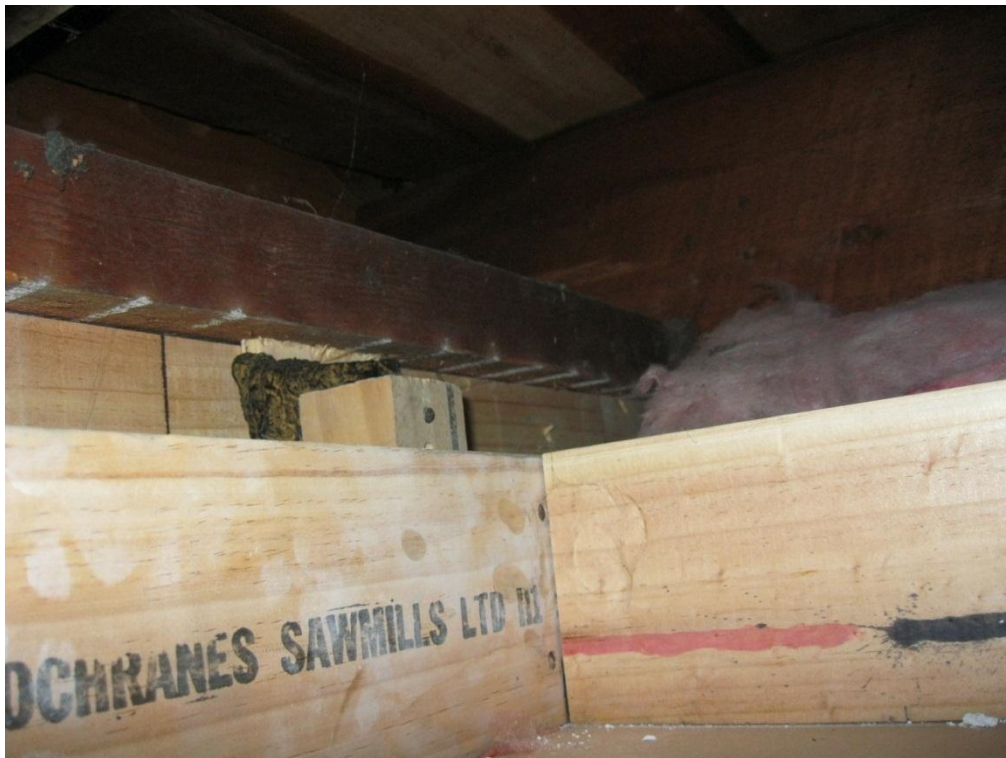
Photograph 21 View inside the roof space close to the intersection of the old roof and the 1996 extension showing old and new timbers and timber roof sarking.
