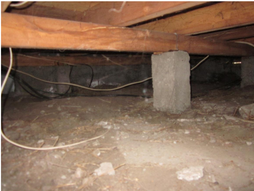
Photograph 10 As above, showing concrete piles.
