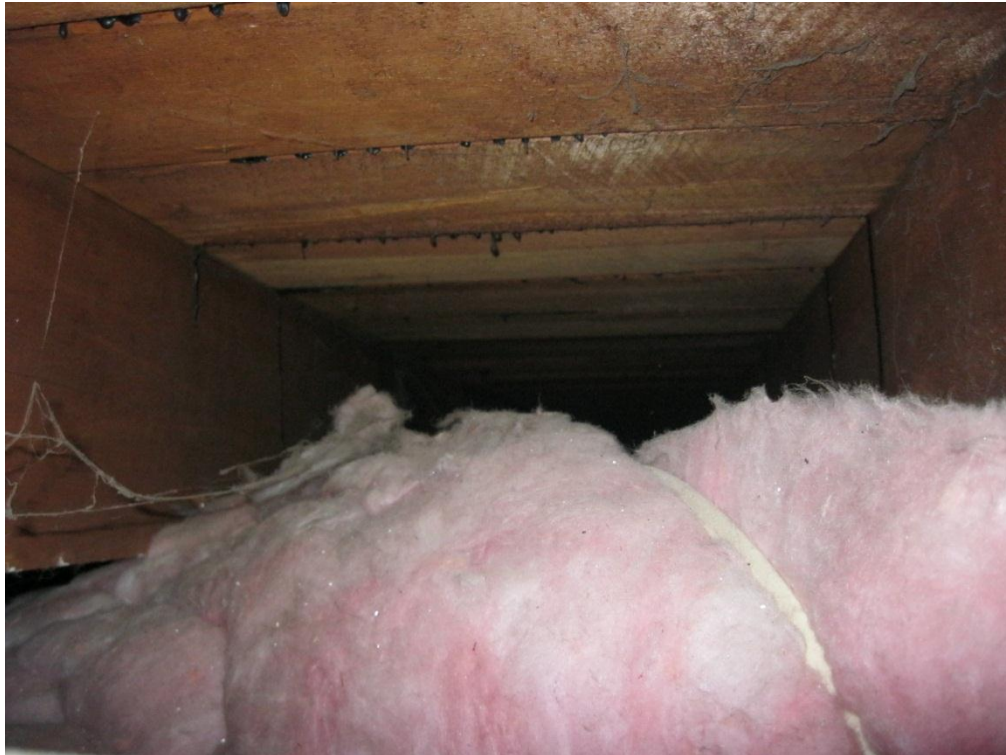
Photograph 22 View inside the roof space from showing timber sarking and roof joists.
