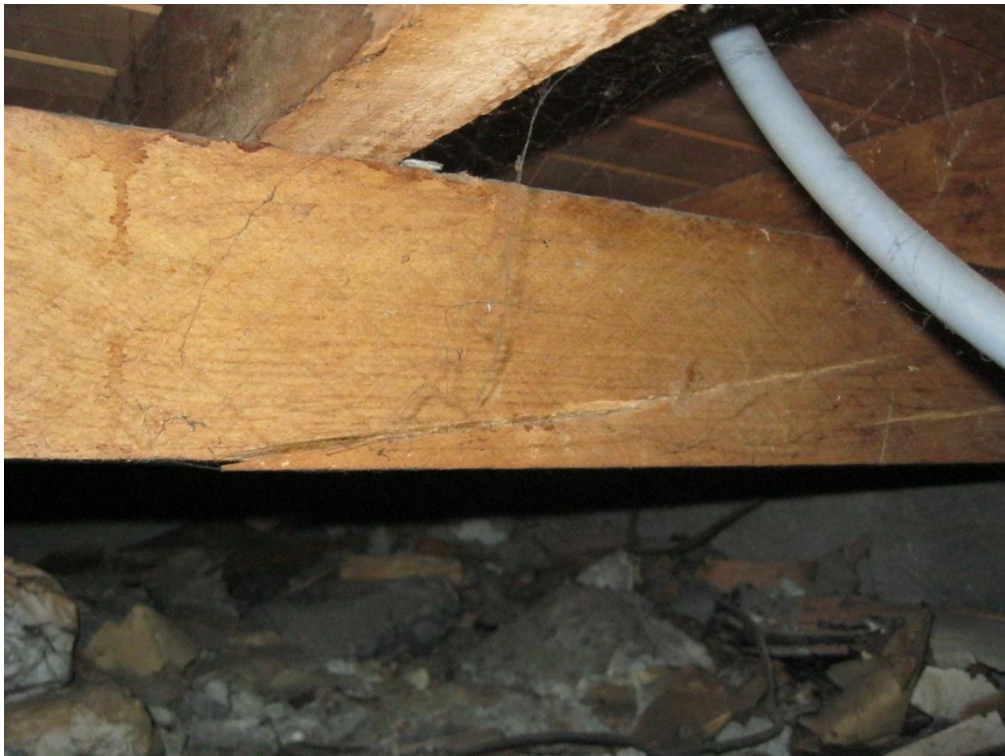
Photograph 20 Cracking noted to suspended timber ground floor bearers following opening up of a section of the floor.
