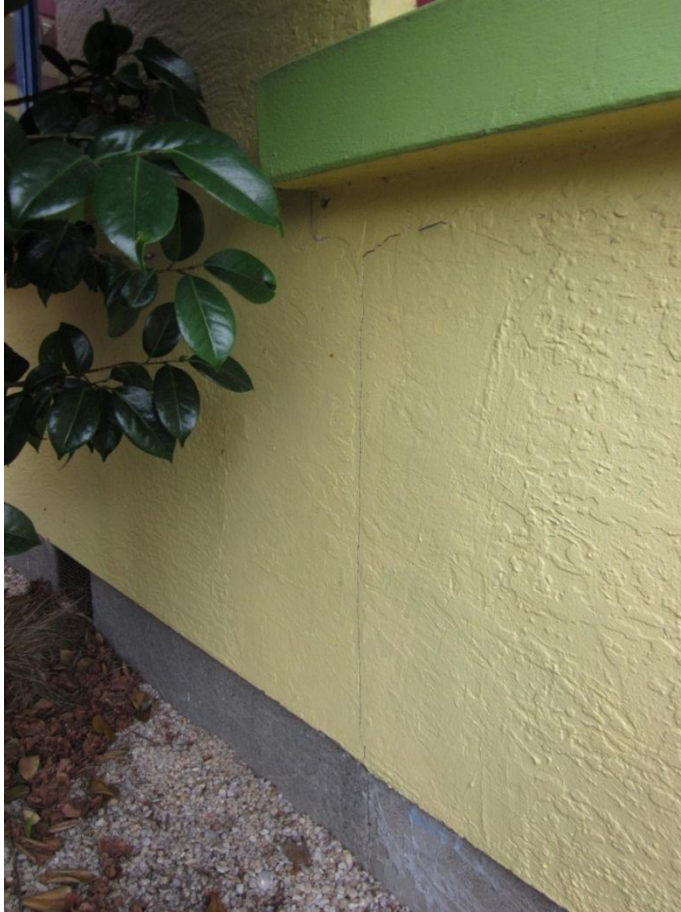
Photograph 3 Cracking below window at construction joint between the original building and the 1971 extension on the south-west.
