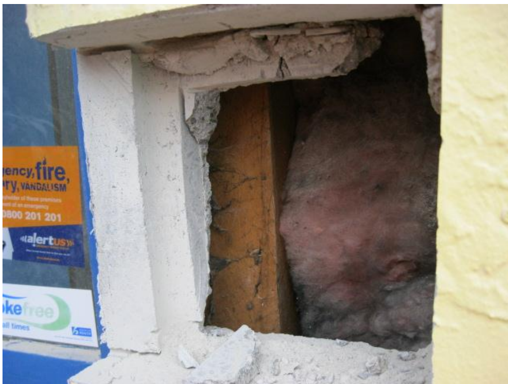
Photograph 16 No evidence of expected steel reinforcement as shown in CCC plans.
