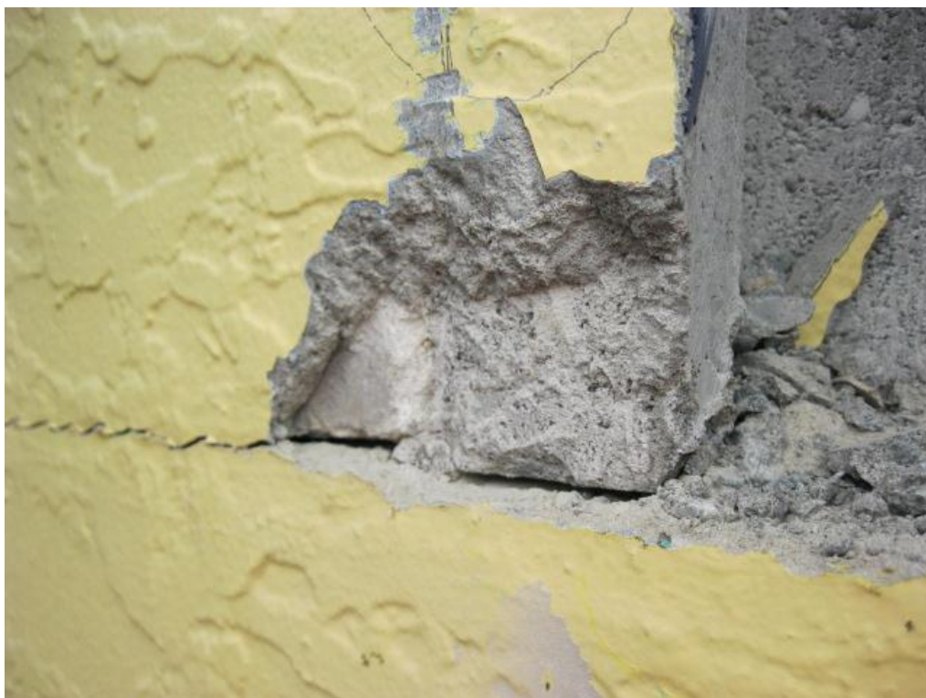
Photograph 12 Cracking penetrates through the wall along the mortar joint.
