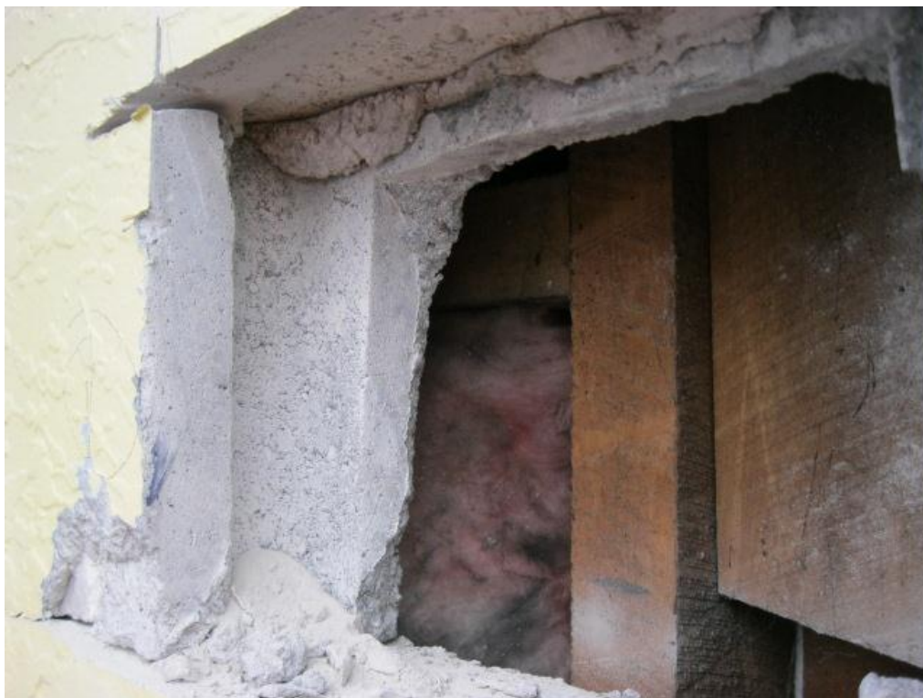
Photograph 13 Section of wall removed to expose a timber frame internal wall.
