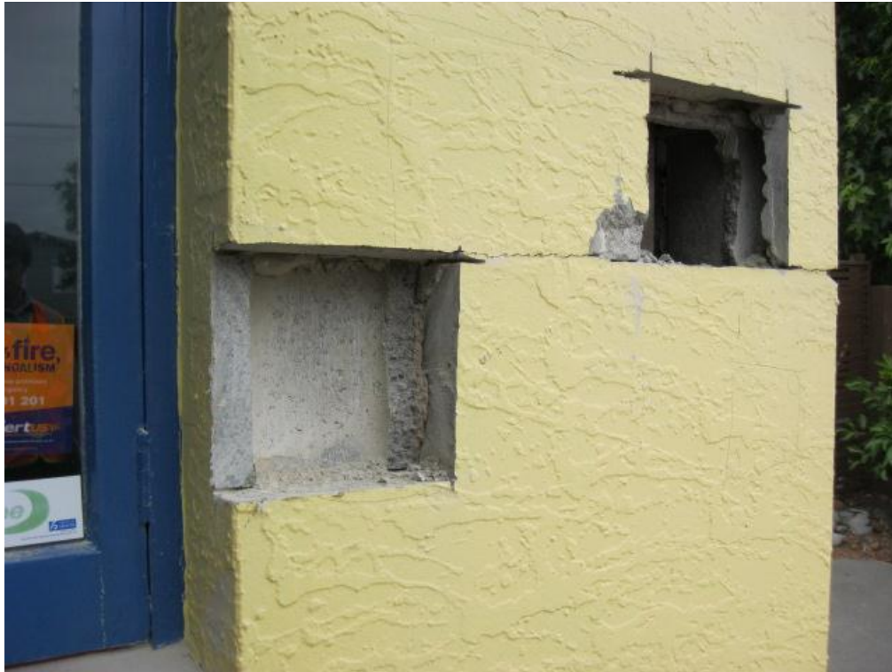
Photograph 15 Second section opened to expose steel reinforcement closer to window as shown in the CCC plans.
