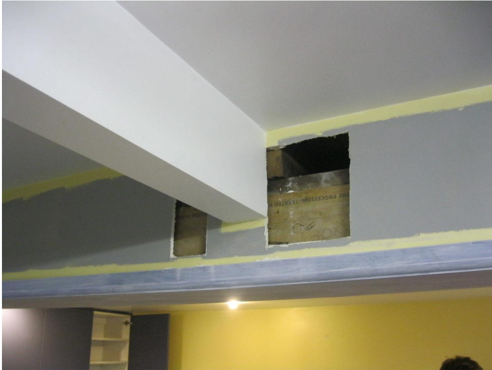
Photograph 19 Opening up around the connection of the 1996 extension beam to the roof support lintel. Connection detail differs to detail on record.
