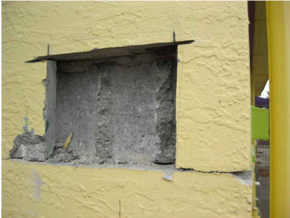
Photograph 11 Section of wall removed to expose steel reinforcement at the southernmost corner of the building.
