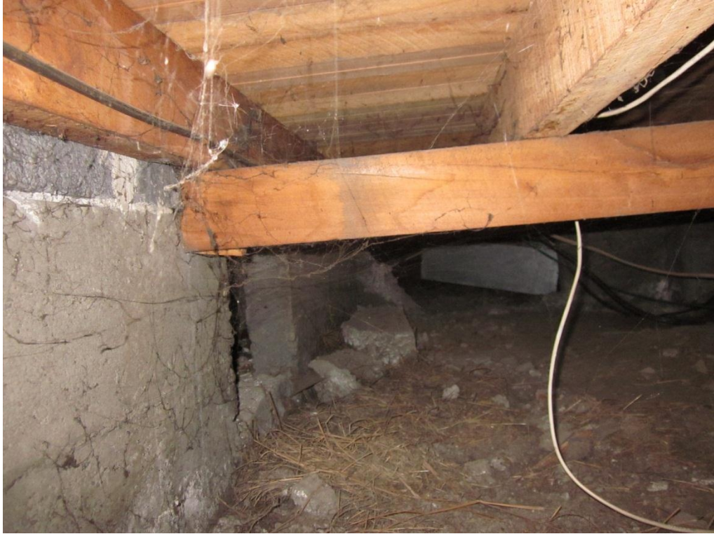
Photograph 9 Subfloor view looking South East along strip foundation to internal masonry wall.
