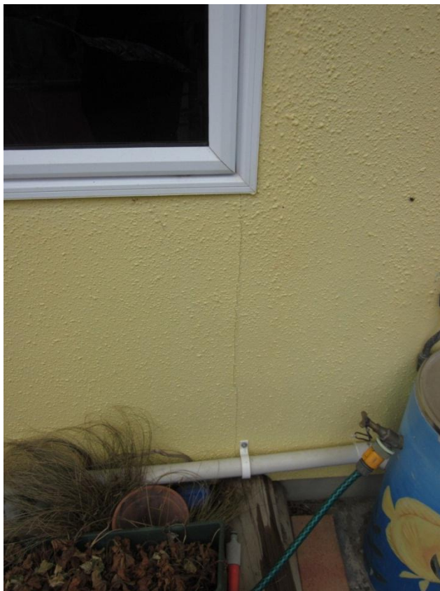
Photograph 6 Cracking below windows of the 1996 extension to the north-east of the building.
