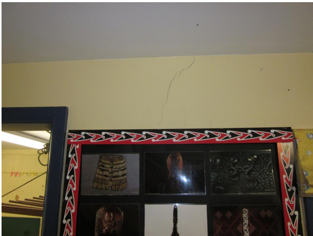
Photograph 7 Cracking of masonry wall where external walls connect to internal .
