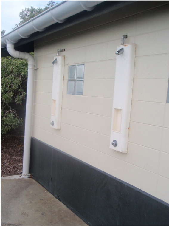
Photo 3: East Wall Elevation (wash down area)
