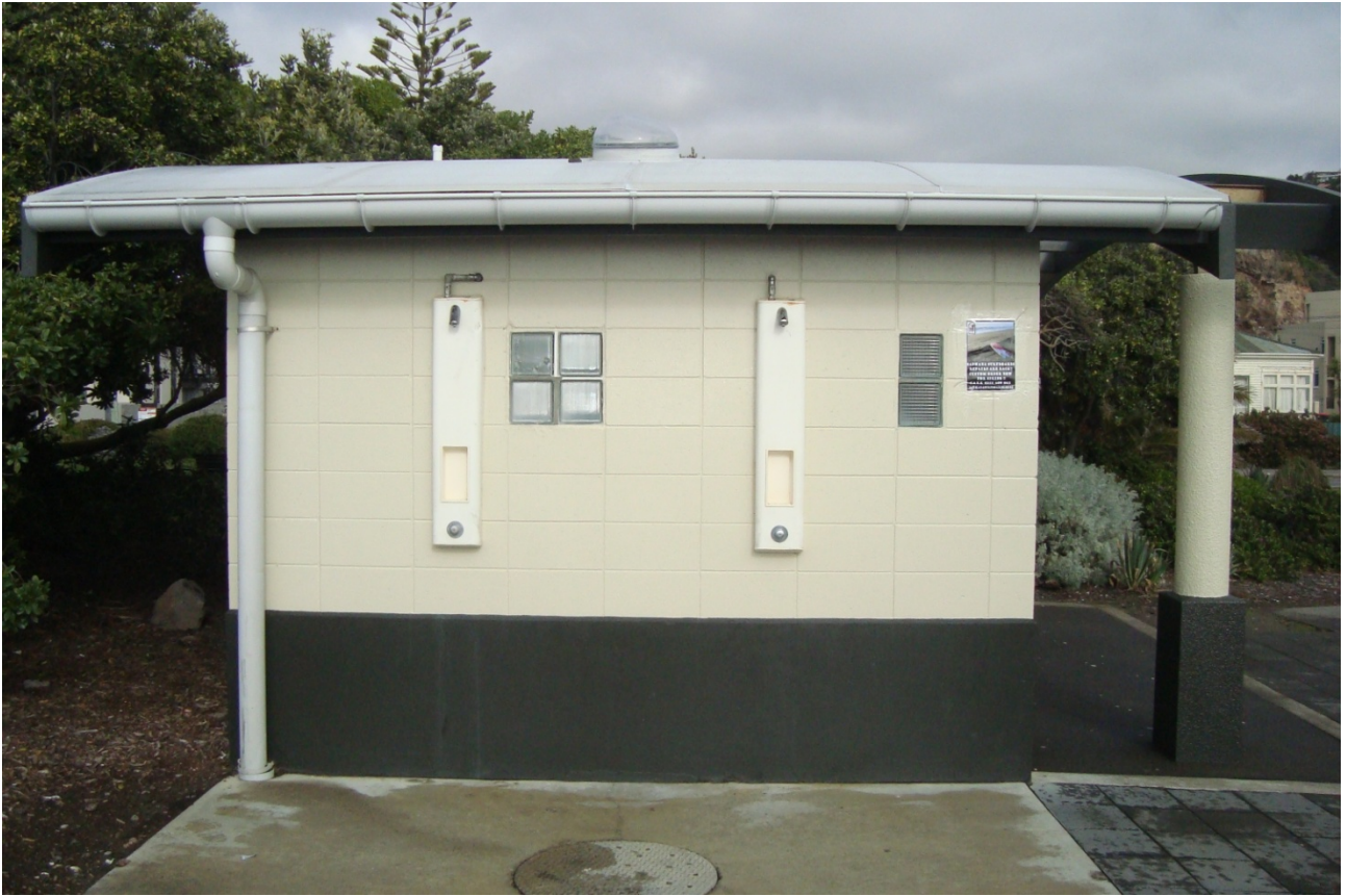
Photograph 3: East Elevation of Sumner Beach Toilet.
