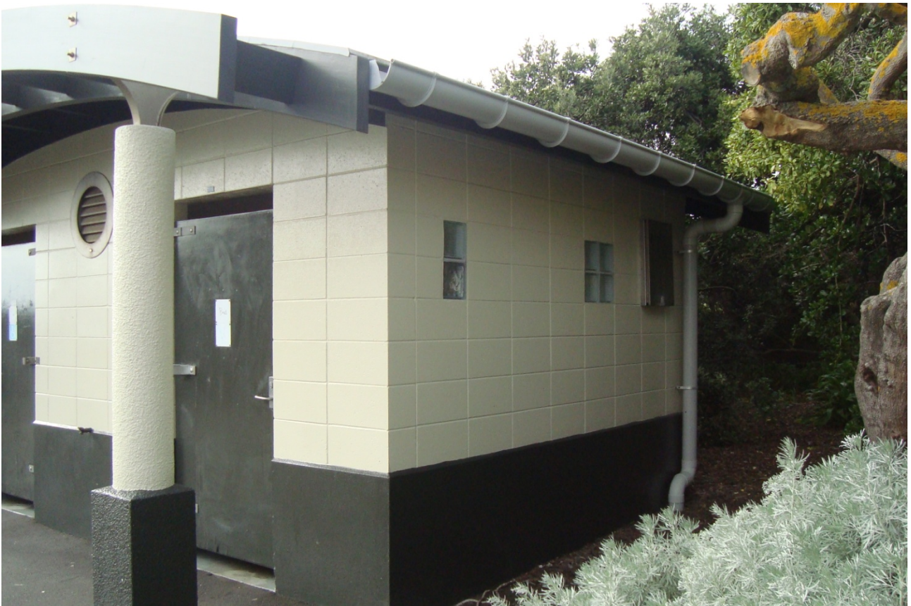
Photograph 4: West Elevation of Sumner Beach Toilet.
