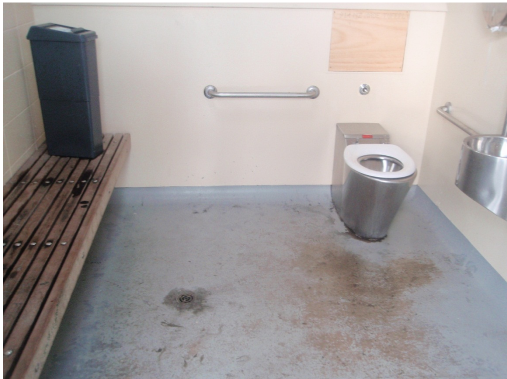
Photo 5: East Toilet Cubicle (West similar)
