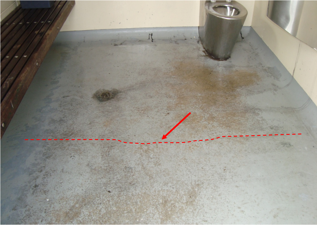
Photograph 7a: 2mm wide cracks floor slab inside the toilets.
