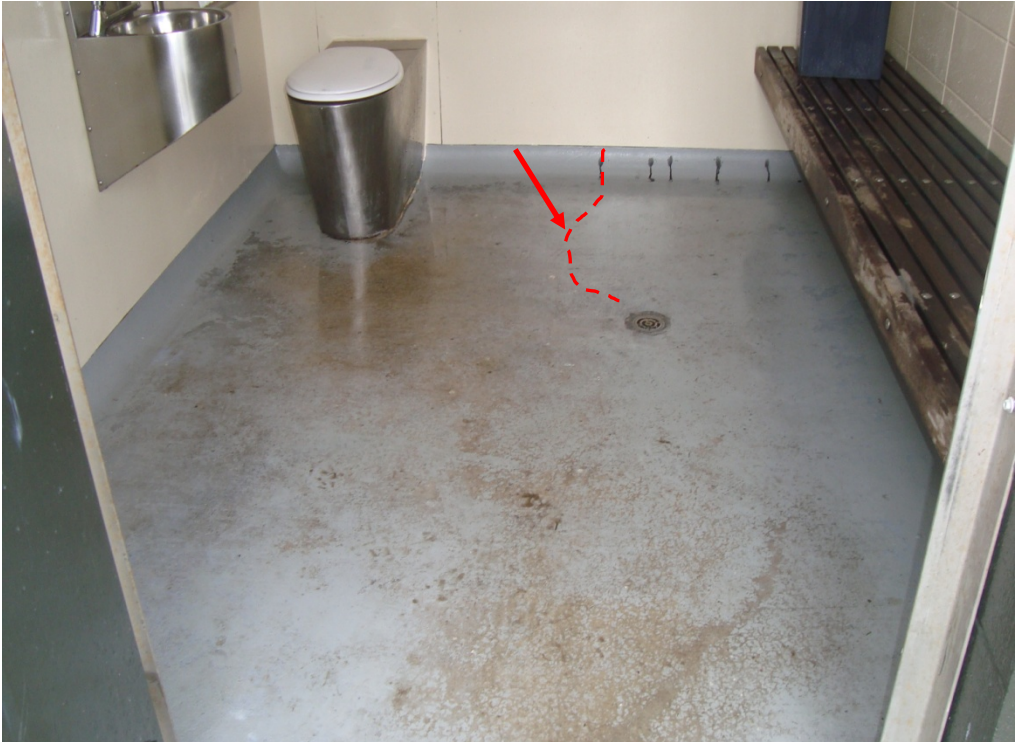
Photograph 7b: 2mm wide cracks floor slab inside the toilets.
