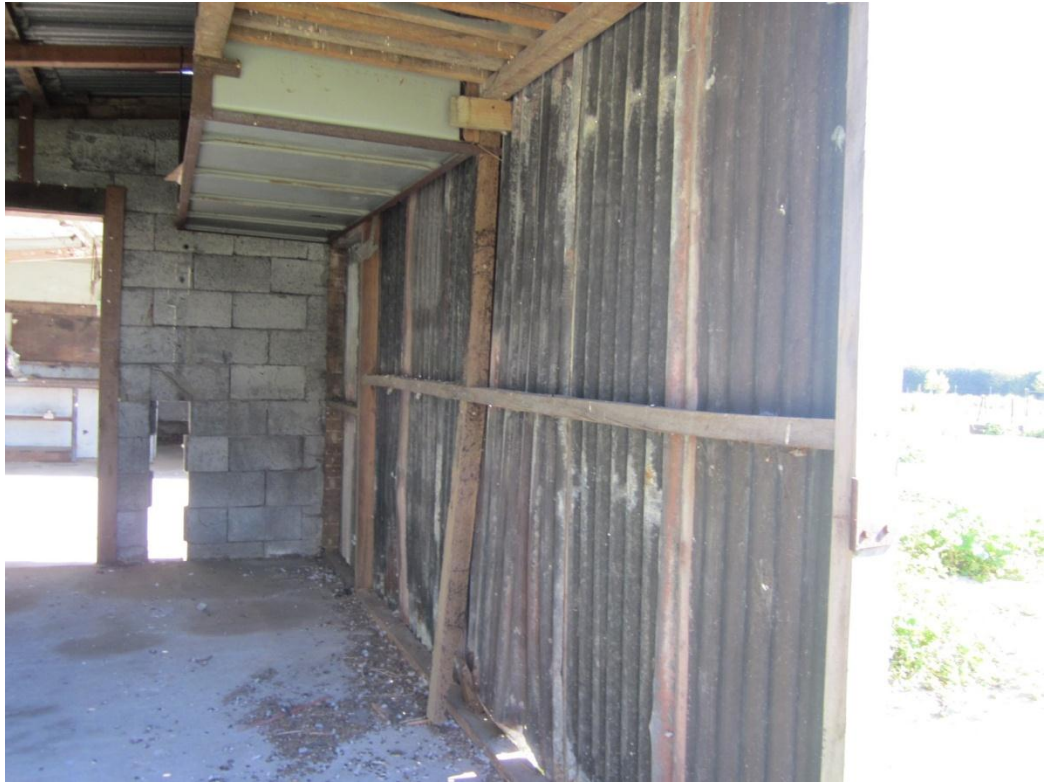
Photograph 9: Displaced timber wall and missing masonry at northern room.
