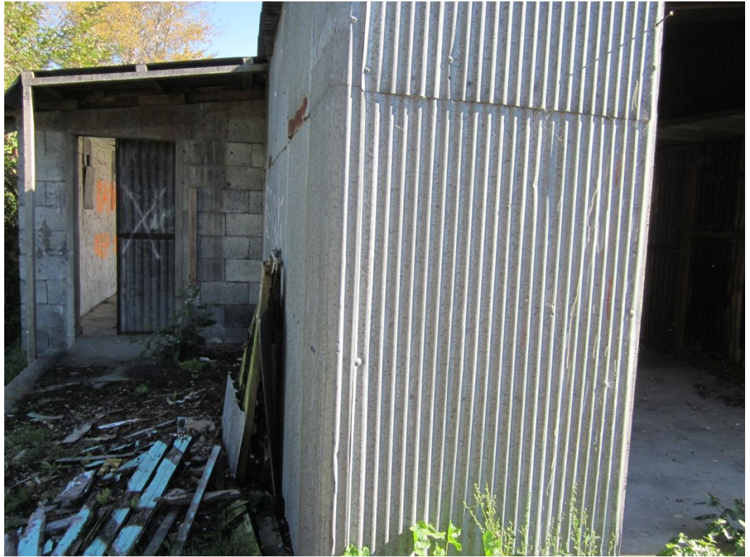
Photograph 3: East elevation at Southeast corner.
