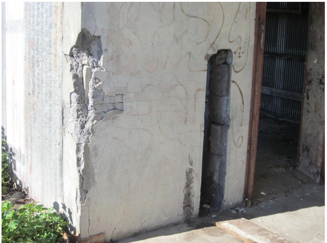
Photograph 10: Damaged masonry walls at southeast corner.
