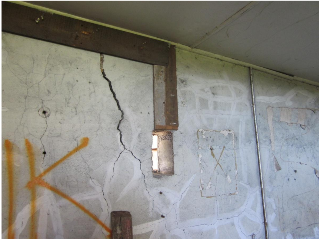
Photograph 13: Damaged masonry wall at western entry area.
