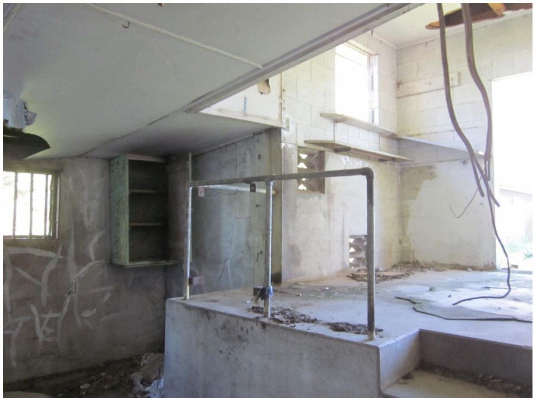
Photograph 8: Interior view of western entry area (facing southwest).
