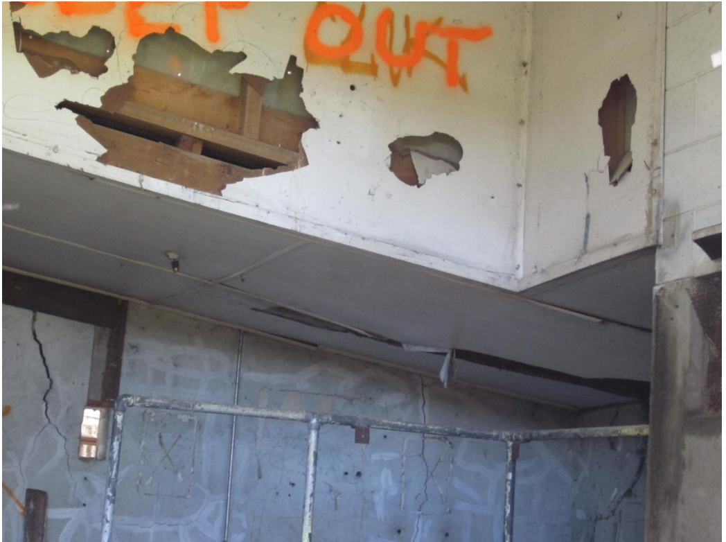
Photograph 11: Damaged linings and concrete walls at western entry area.
