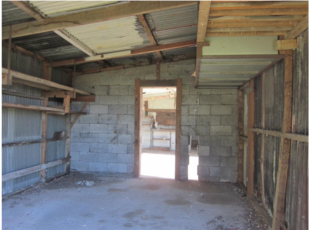
Photograph 7: Interior view of western room (facing east).
