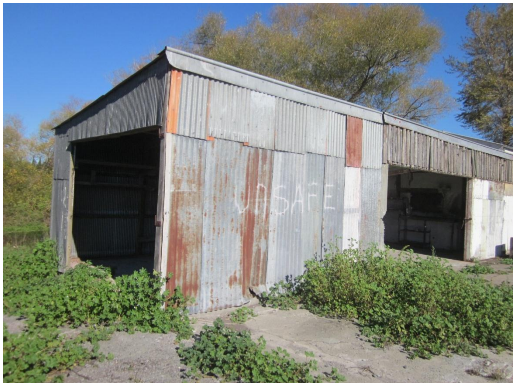
Photograph 2: Northeast corner elevation.
