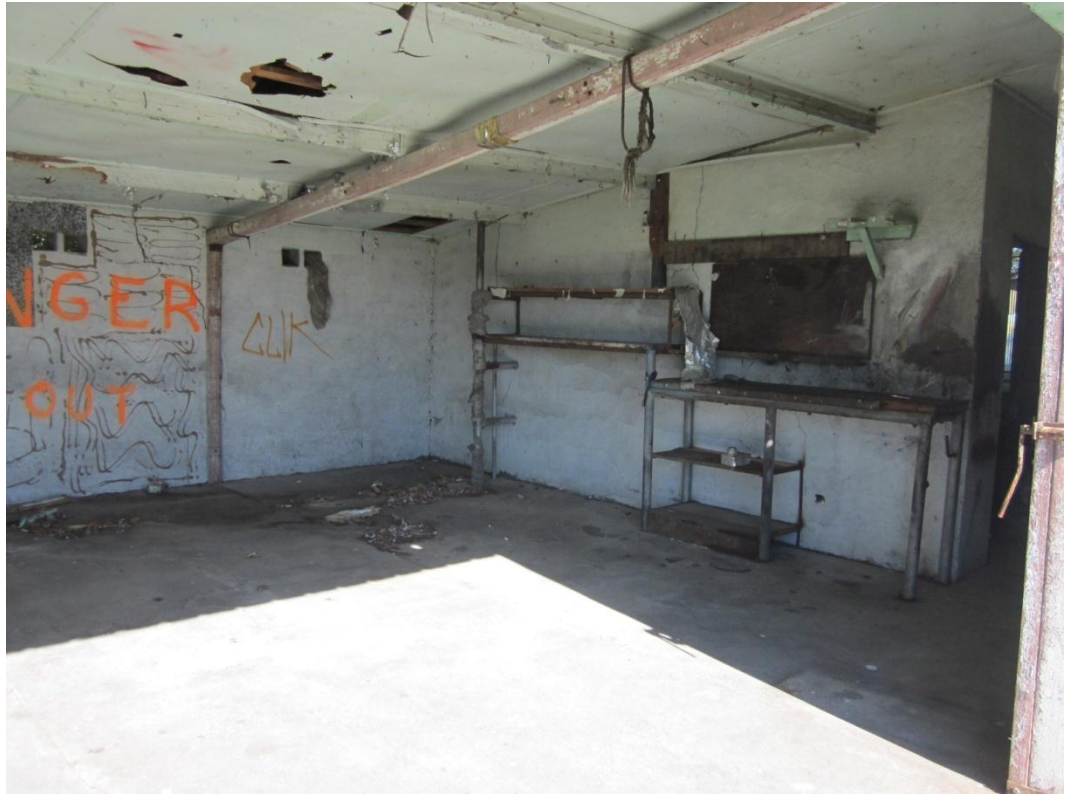
Photograph 5: Interior view of shed from large opening in northern wall.
