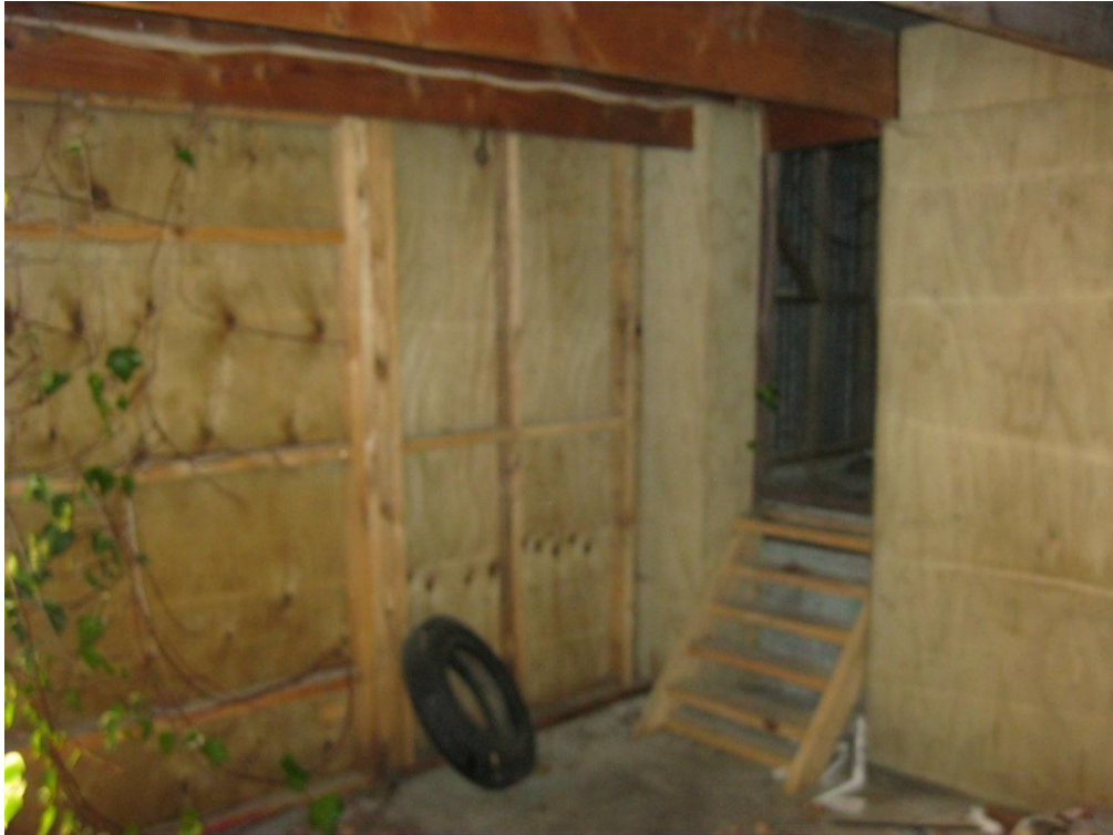
Photograph 3 Internal view of the access to the double garage.
