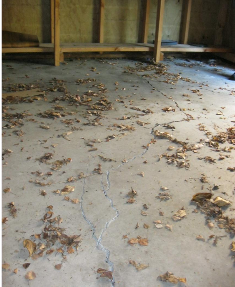
Photograph 5 Internal view of the building showing cracking of the concrete floor.
