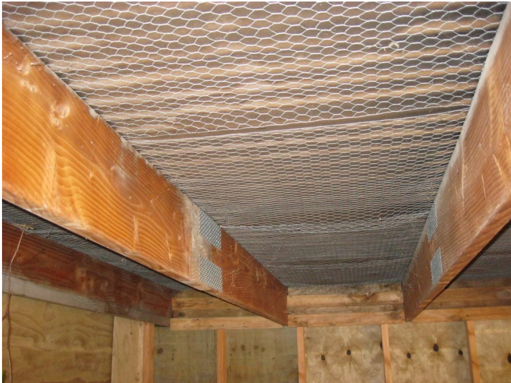
Photograph 4 Internal view of the building showing roof construction and connection of the rafters to the cladding.
