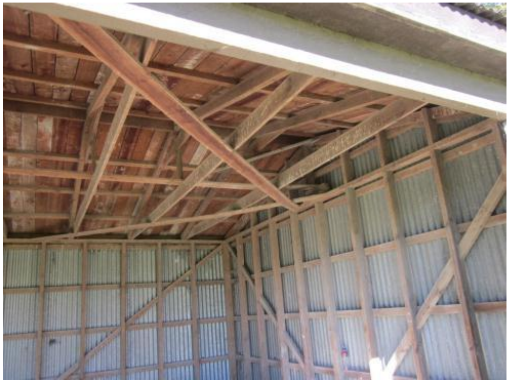
Photograph 3: Interior view at entry of cross-braced walls and truss roof members
