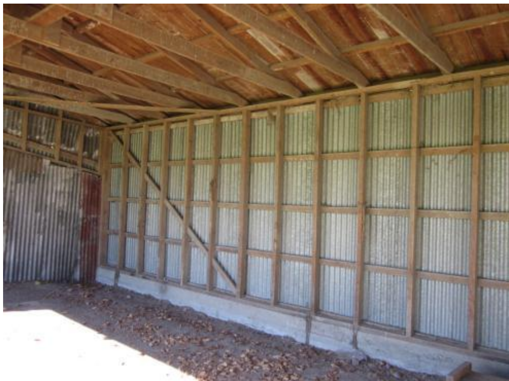
Photograph 6: Interior view of cross-braced rear wall and foundation wall, timber trusses above, and part of northern wall.
