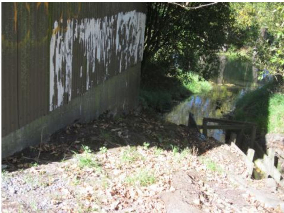
Photograph 10: Proximity of river at southeast corner. Note proximity to the creek.
