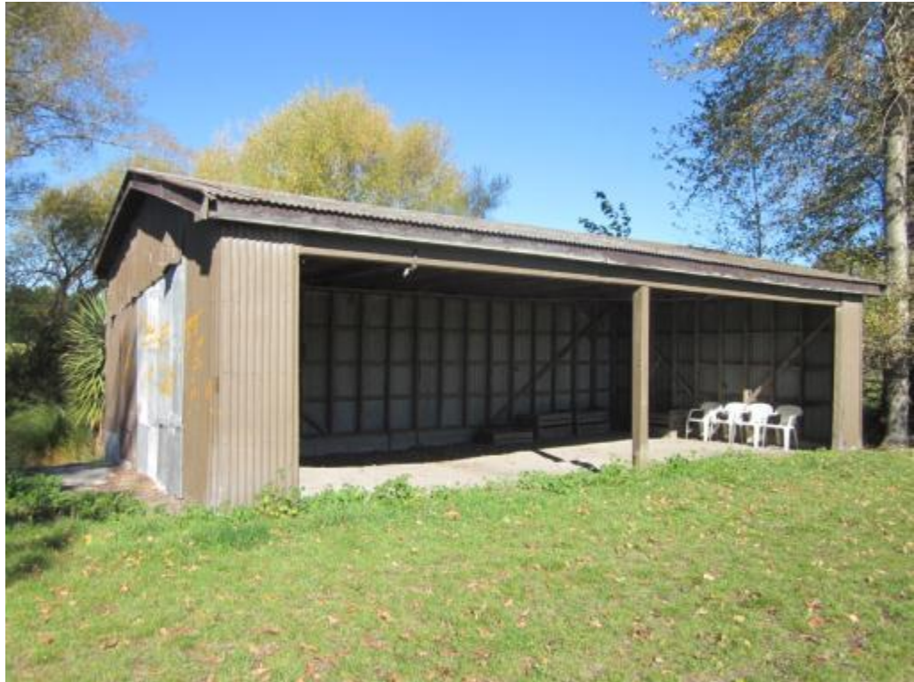
Photograph 1: Northwest corner elevation.
