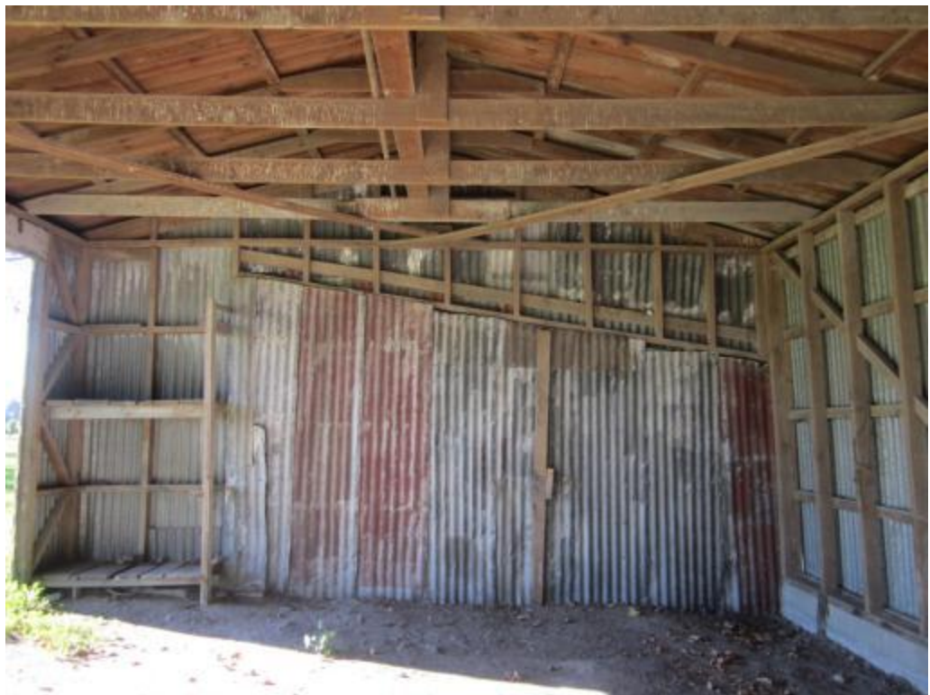
Photograph 8: Interior view of the northern wall, trusses above, partial view of entry and partial view of rear wall and its foundations.
