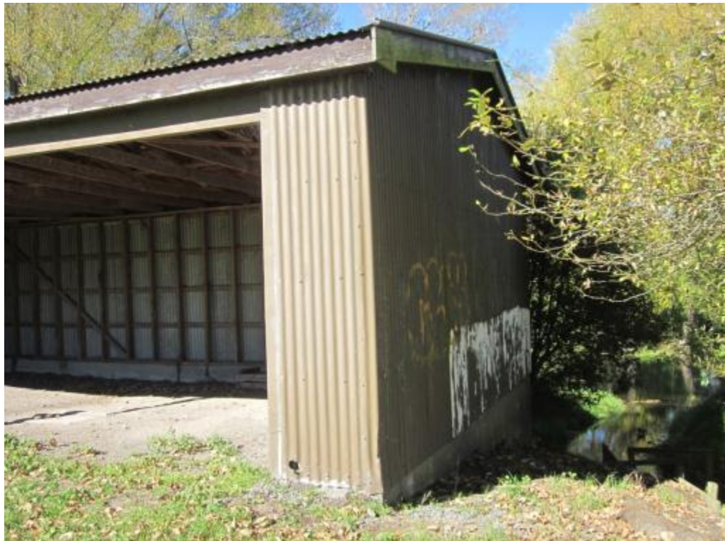
Photograph 2: Southwest corner elevation. Note proximity to the creek at the corner of the building.
