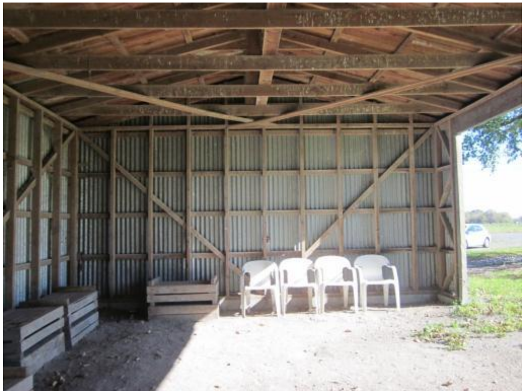
Photograph 7: Interior view of southern wall and foundations below, trusses above, and partial view of entry.
