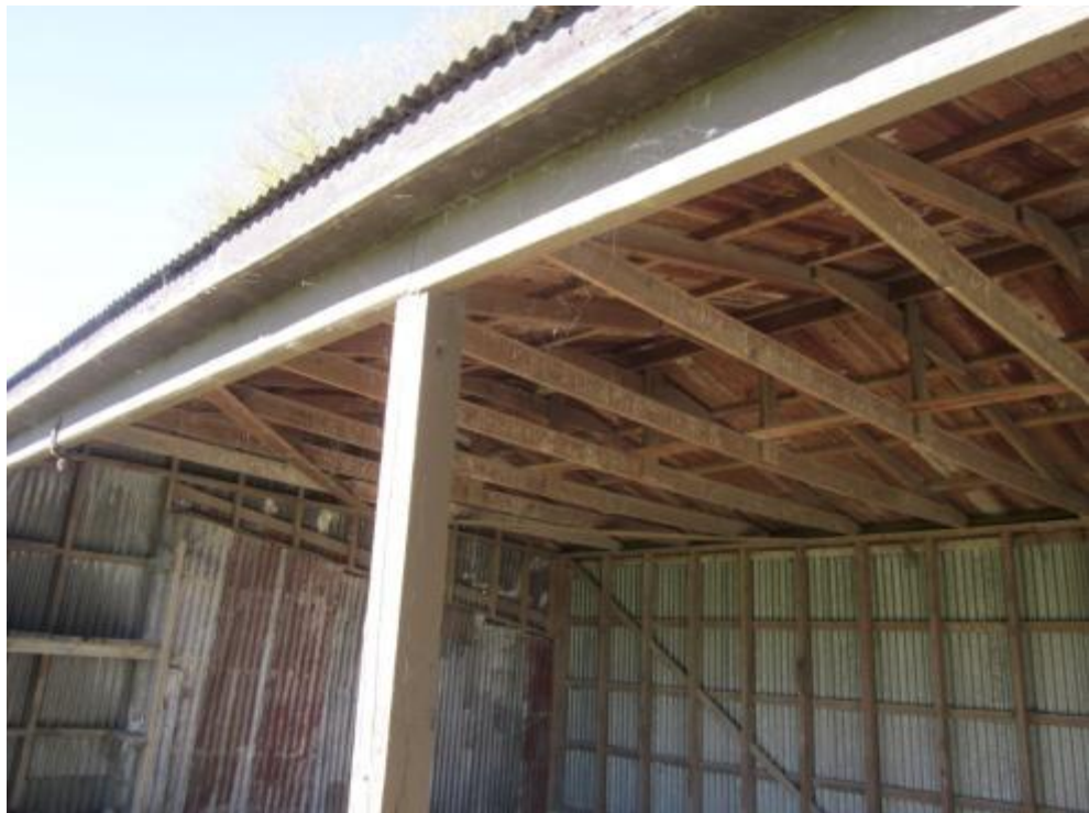
Photograph 4: Interior view at entry of cross-braced walls and truss roof members, including mid-span lintel post.
