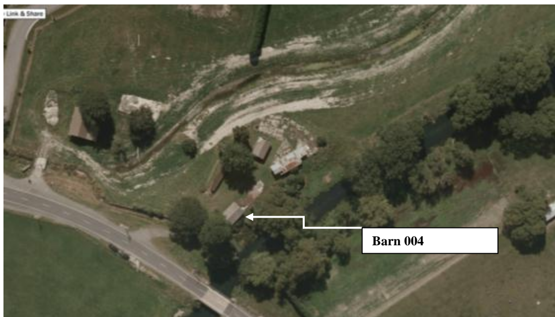
Figure 3 Post February 2011 Earthquake Aerial Photography 2
