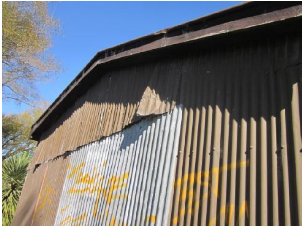
Photograph 9: Exterior wall cladding at northern wall.
