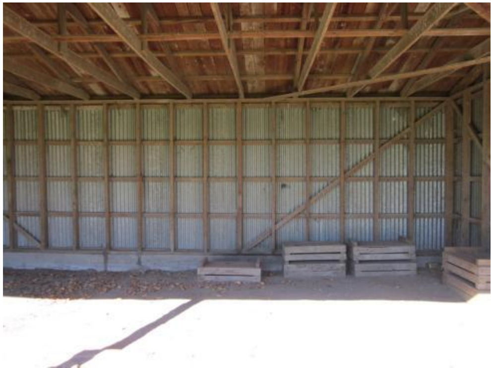
Photograph 5: Interior view of cross-braced rear wall and foundation wall below, and timber trusses above.
