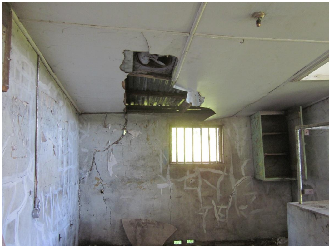
Photograph 10: Damaged walls, ceiling and roof at western entry area.
