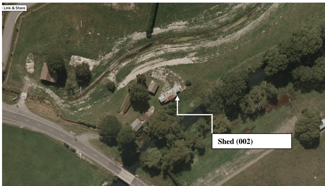
Figure 3 Post February 2011 Earthquake Aerial Photography 2
