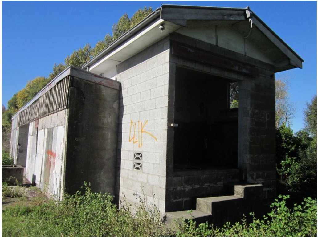
Photograph 1: Northwest corner elevation.
