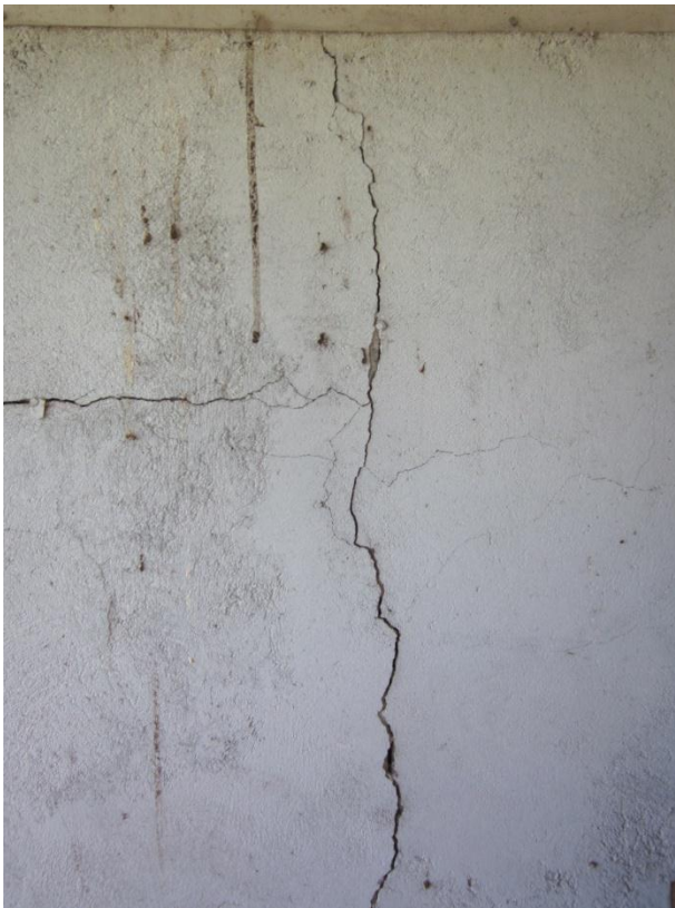
Photograph 12: Damaged masonry wall at western entry area.
