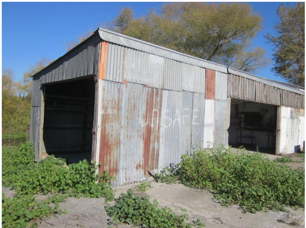
Photograph 2: Northeast corner elevation.
