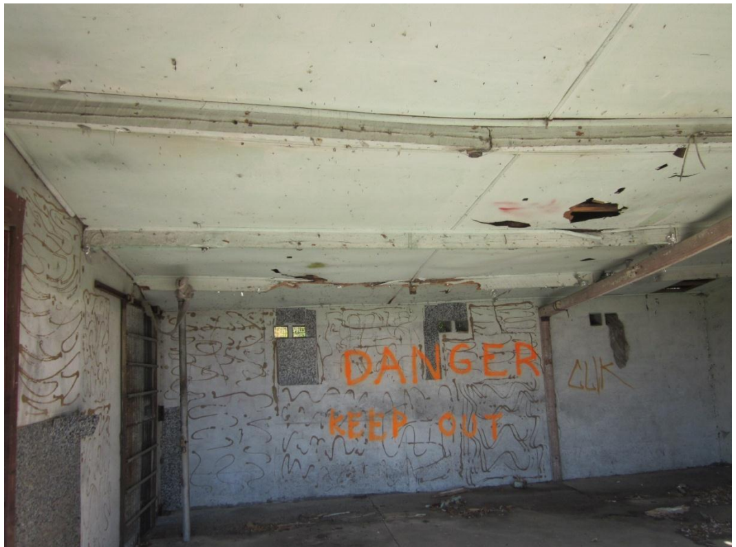
Photograph 6: Interior view of shed from large opening in northern wall.
