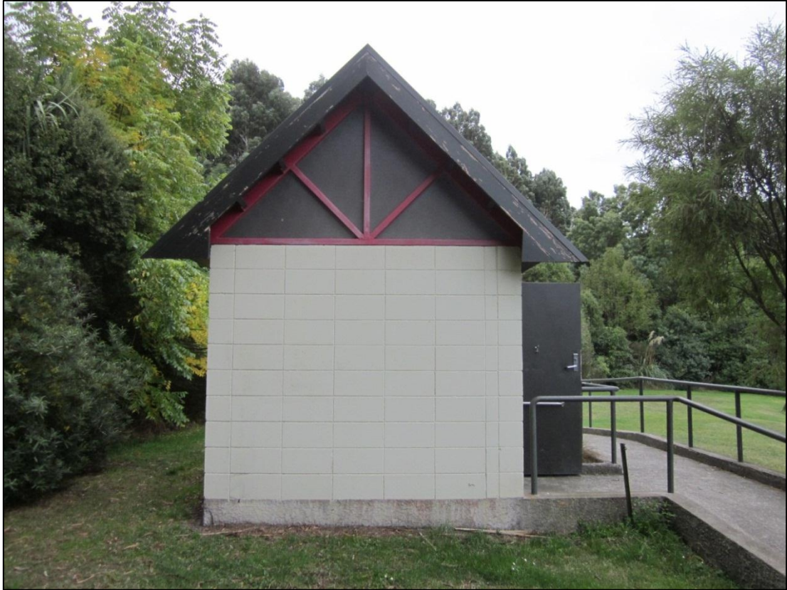
Photo 3 Park Toilet (Sideways, photo is taken facing northeast).
