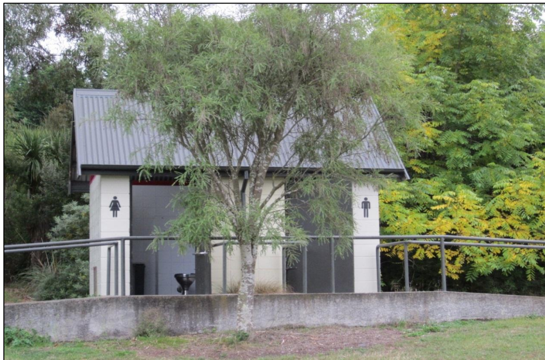
Photo 2 Park Toilet (Front, photo is taken facing northwest).
