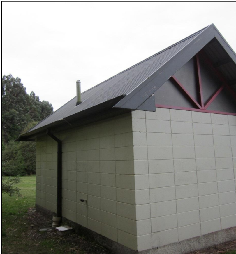
Photo 4 Park Toilet (Rear, photo is taken facing northeast).
