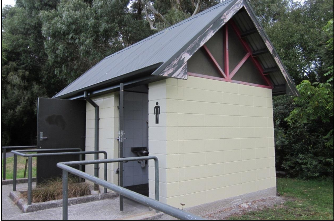
Photo 5 Park Toilet (Sideways, photo is taken facing southwest).
