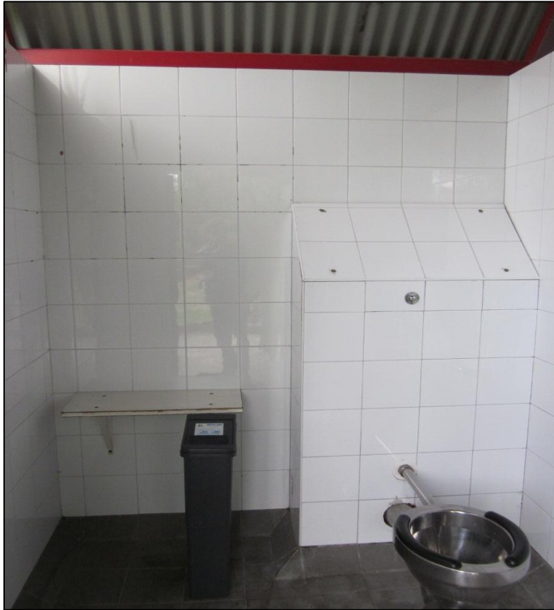
Photo 7 View of ceramic tiles cladding the perimeter and partition walls.
