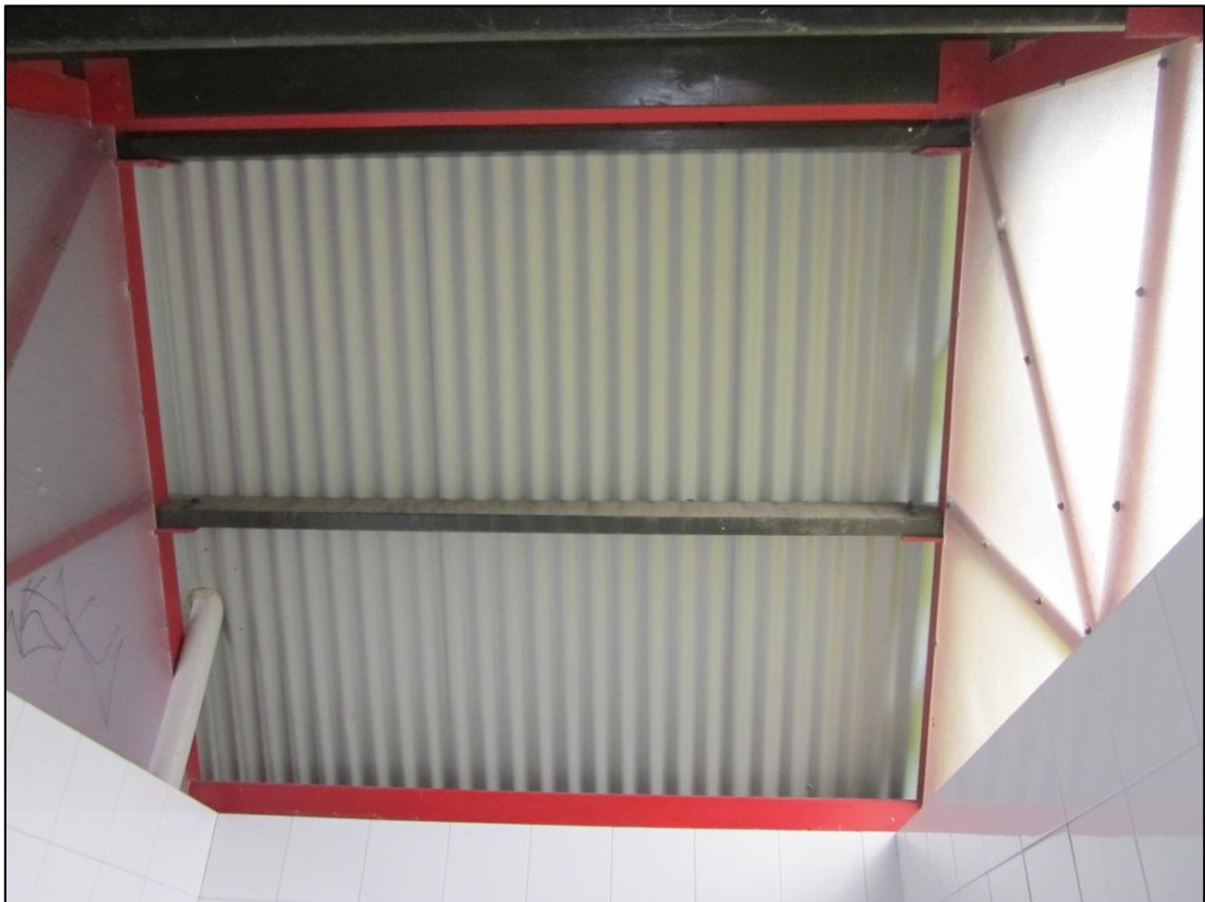
Photo 6 View of the roof structure.
