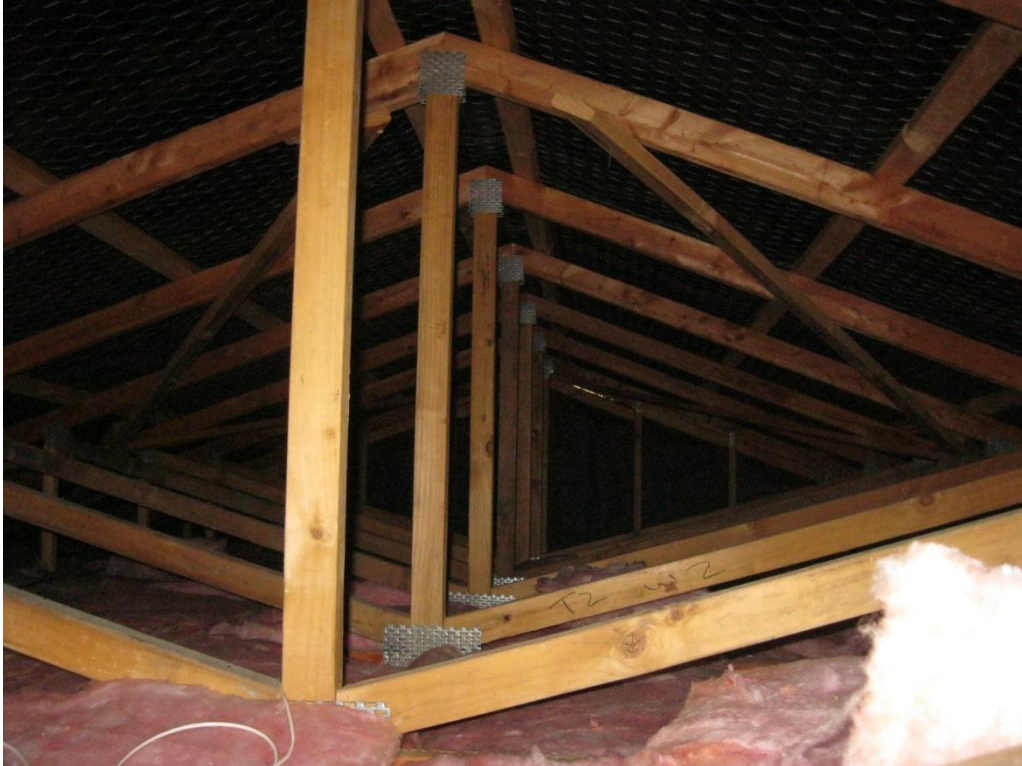
Photograph 6 View of roof trusses and diagonal bracing.
