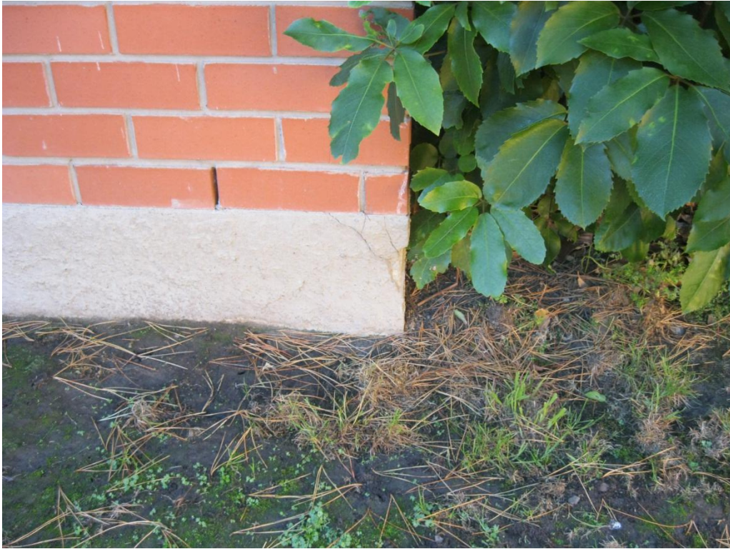
Photograph 5 Cracking in strip footing render.
