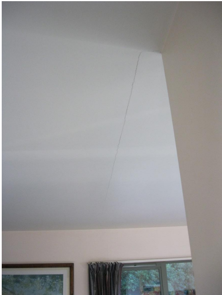
Photograph 3 Minor cracking above window.
