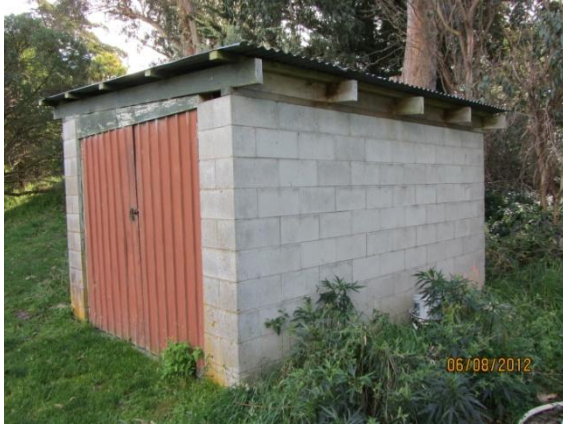
Photo 1: View of Stoddart Point Reserve Garage
