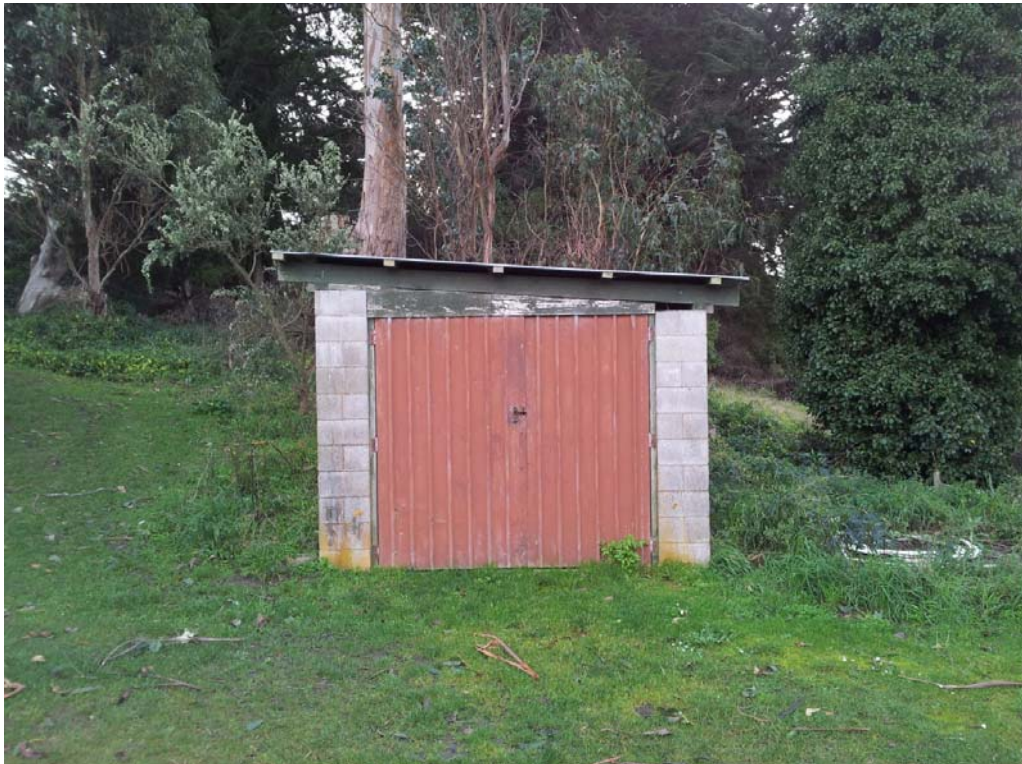
■ Figure 3 - Overview of the building (southern elevation)
