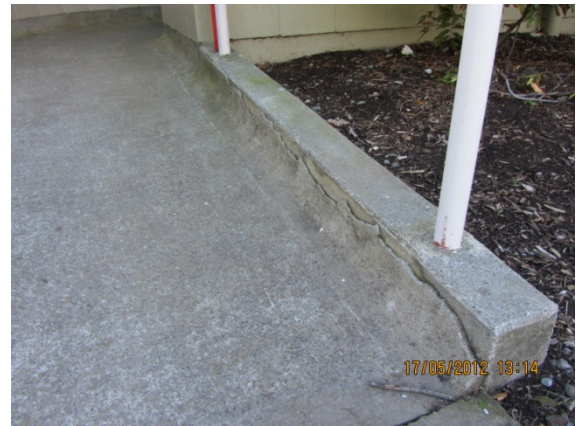
Photo 18: Spalling at coving in mens toilet entrance
