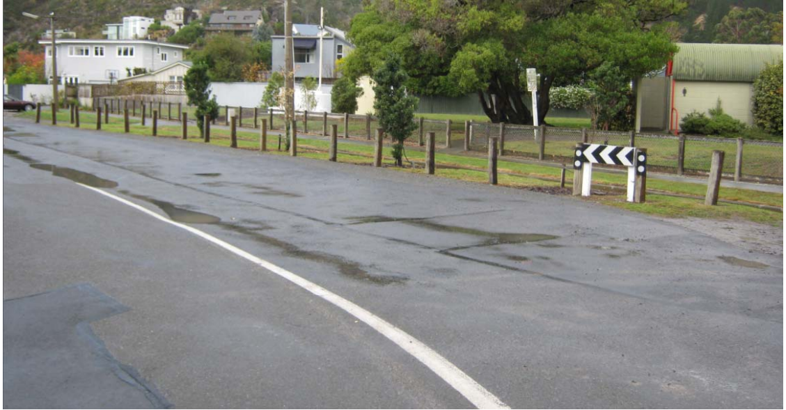
■ Figure 6: Possible settlement of service trenches on Duncan Street near the toilet block.
