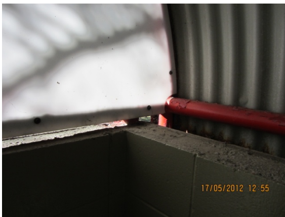
Photo 11: Photo above the walls showing the masonry is filled
