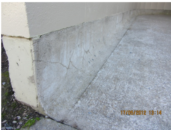
Photo 19: coving in mens toilet entrance showing signs of deterioration
