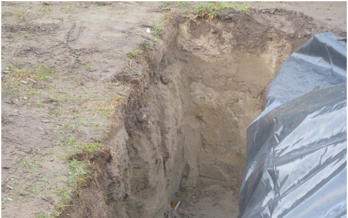
■ Figure 6: Excavation of ground indicating sand to 1 m depth with no groundwater.
