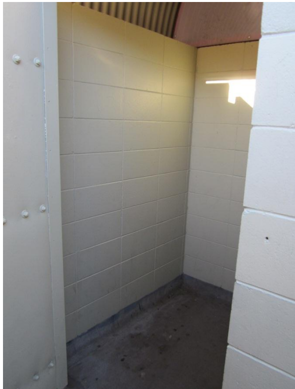
Interior view of reinforced concrete block walls.
