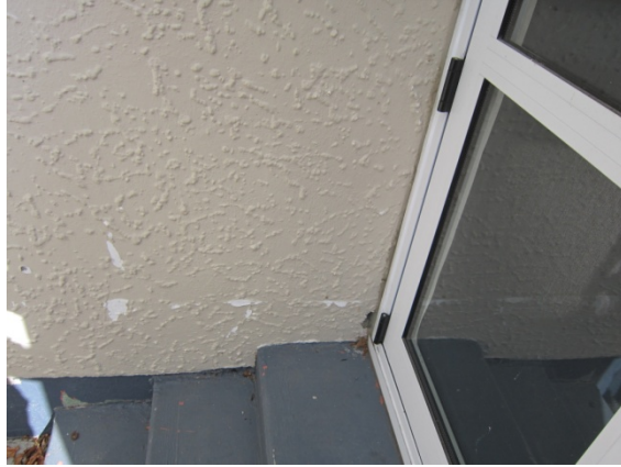
Photo 9: Cladding damage at the South east entry
