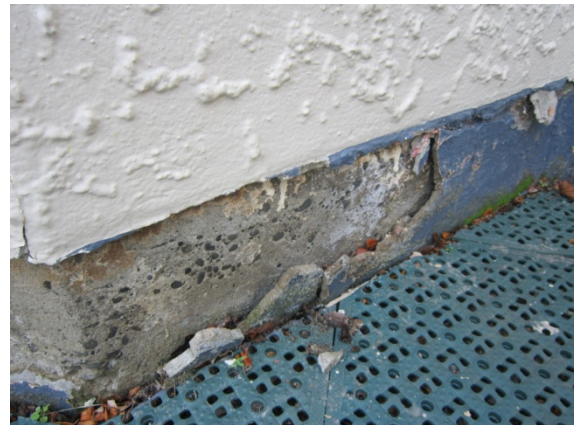
Photo 20: Detail of perimeter ring beam
