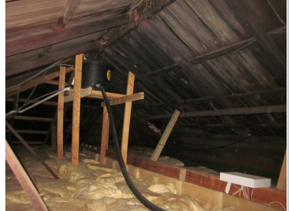
Photo 42: View of Creche roof space
