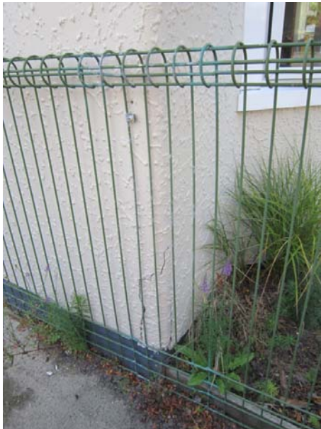
Photo 11: South west corner damage
