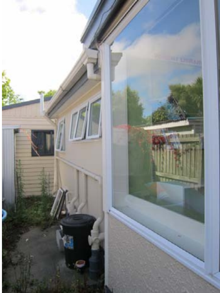
Photo 5: West side looking North along Creche to offices
