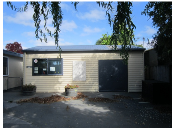
Photo 36: Office and storage building
