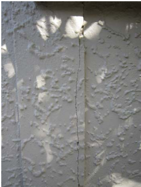
Photo 7: One of the larger exterior cladding cracks
