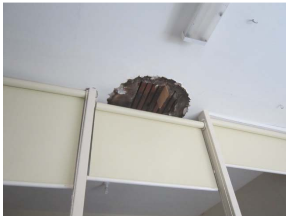
Photo 27: Roof opening showing lathe and plaster ceiling system
