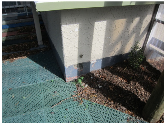
Photo 15: Cracking to the perimeter ringbeam south east corner
