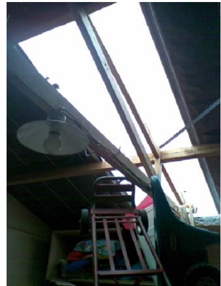
Photo 40: No damage to the timber trusses was observed
