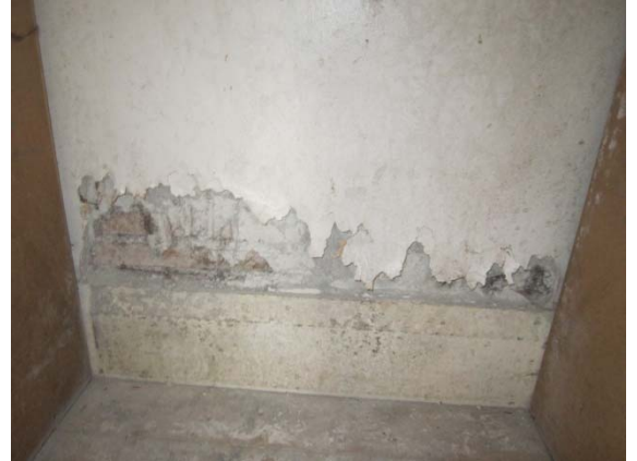
Photo 26: Open area of wall showing lathe and plaster bracing
