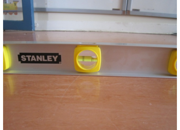
Photo 34: Severe dip to the North
