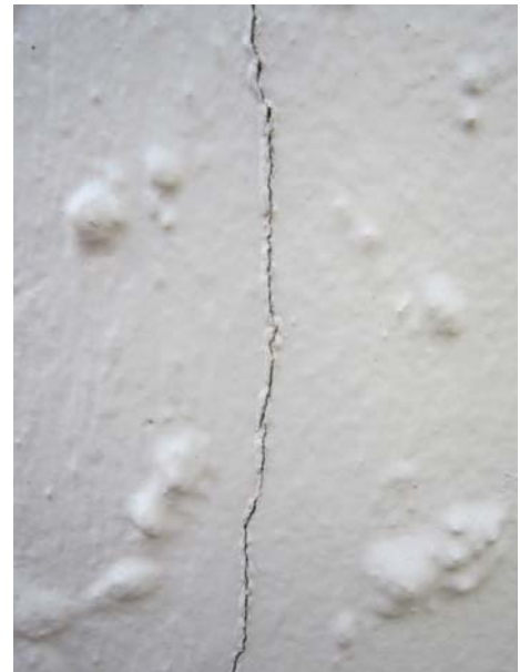
Photo 24: Cracking hairline – 0.3mm typically
