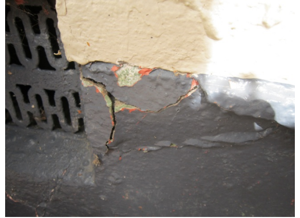
Photo 14: close up of perimeter ring beam damage
