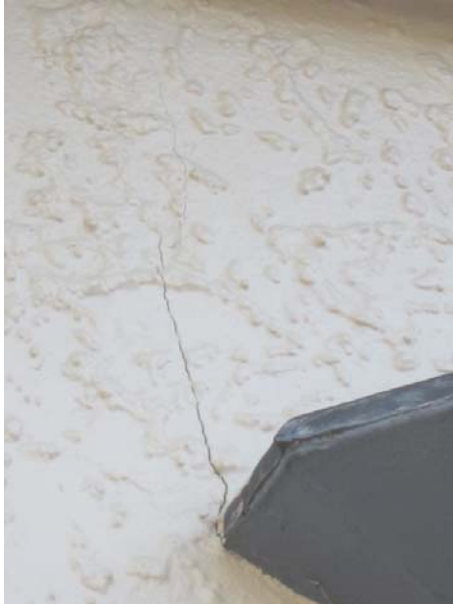
Photo 21: Typical cracking seen around wall penetrations
