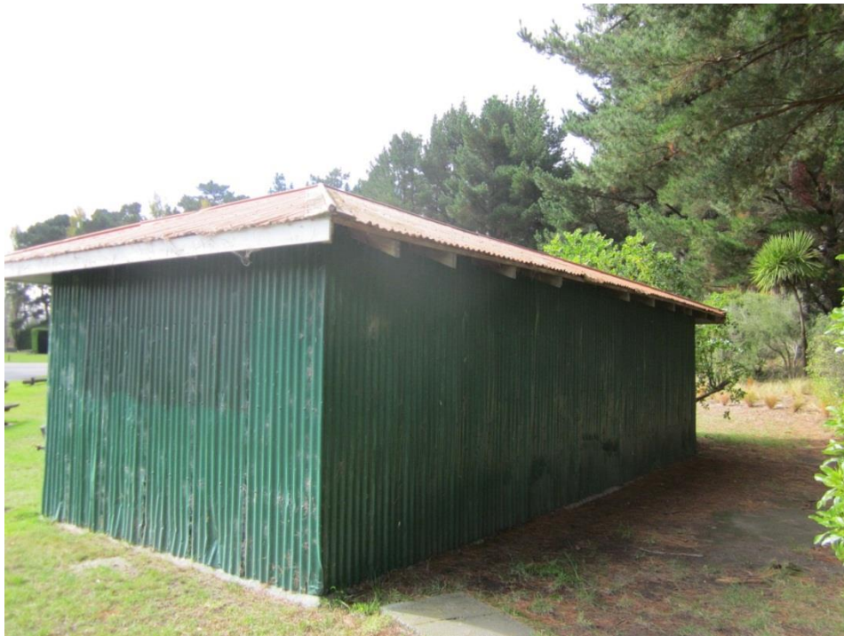
Building southern elevation
