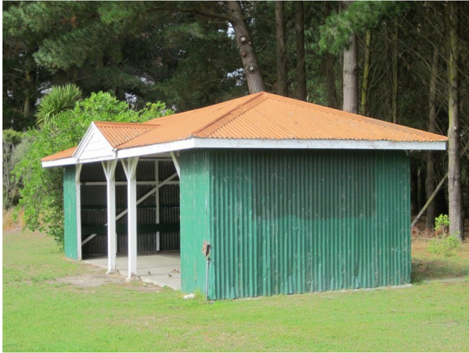
Building northern elevation
