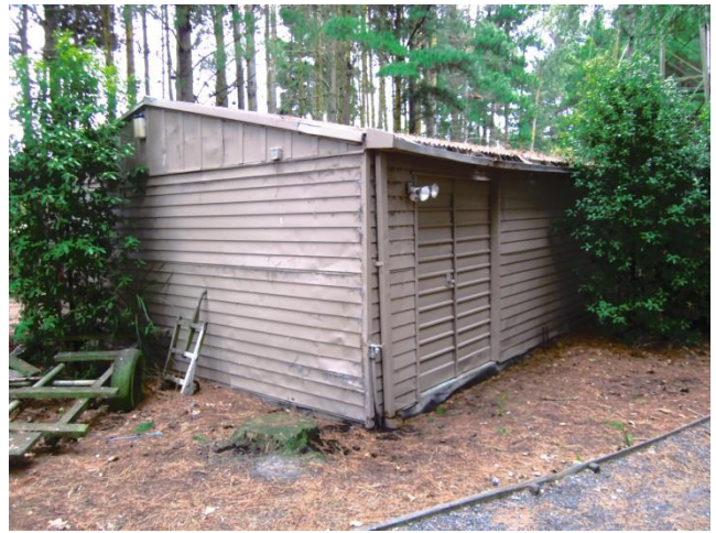
North Western elevation of the Spencer Park Camping Ground Workshop.
