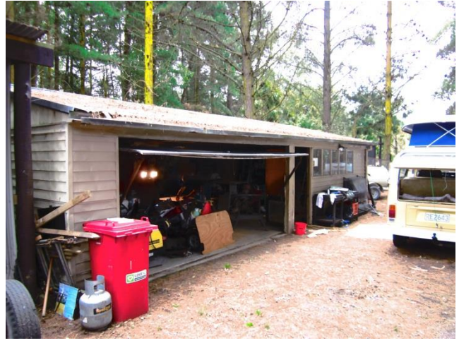
South Eastern elevation of the Spencer Park Camping Ground Workshop.
